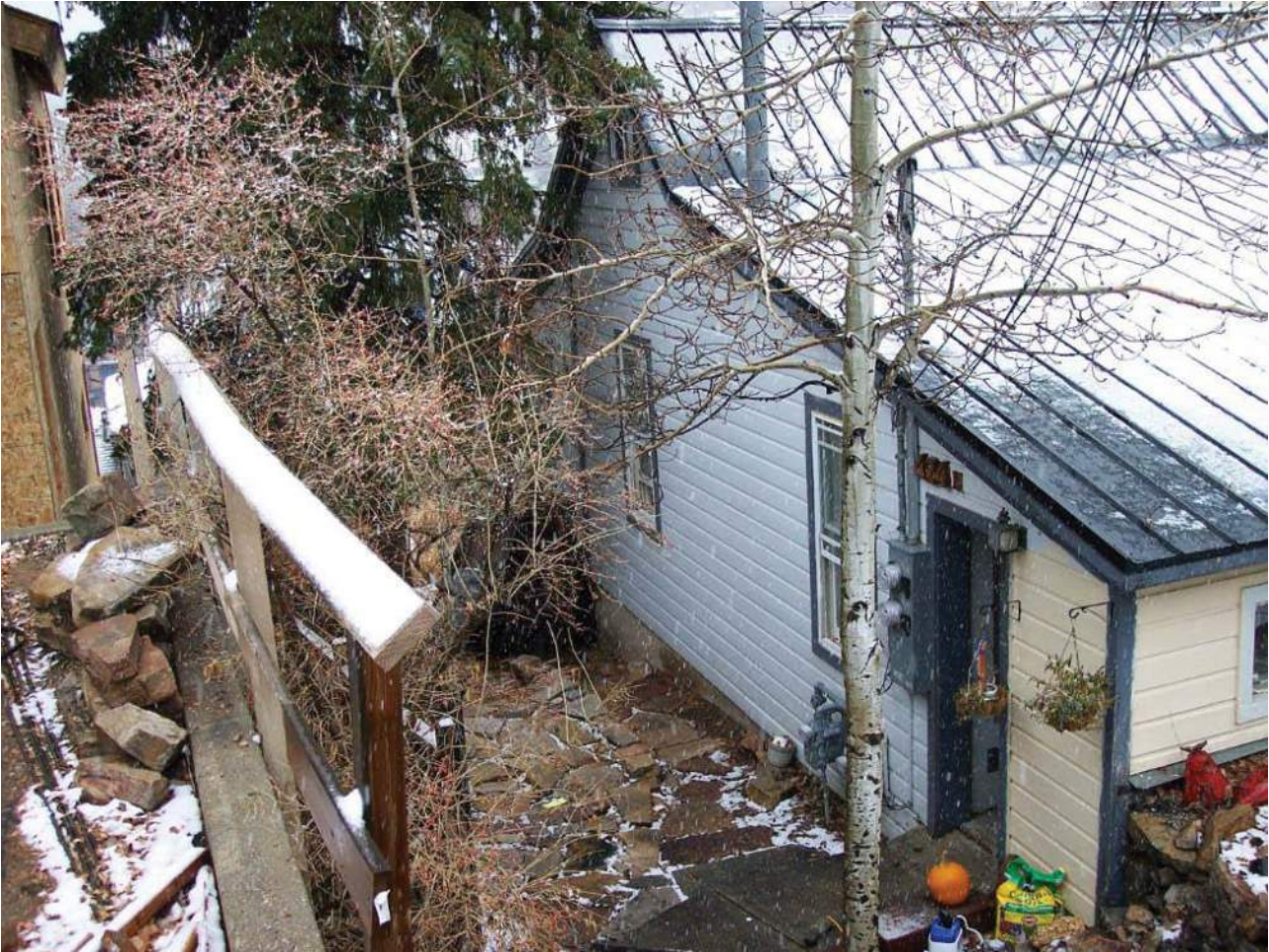
Roof looking southeast
