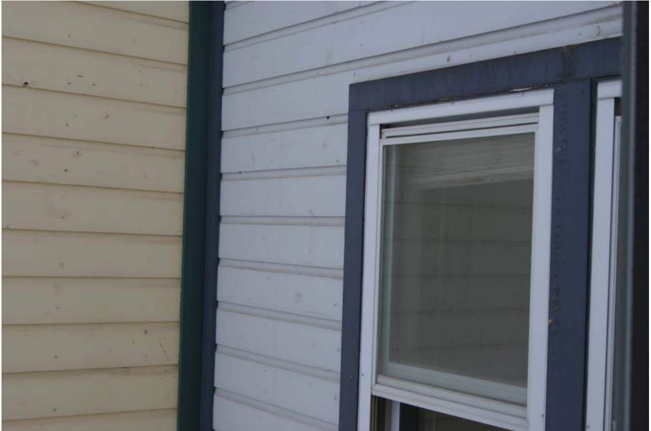
Wood aluminum clad window- typical
