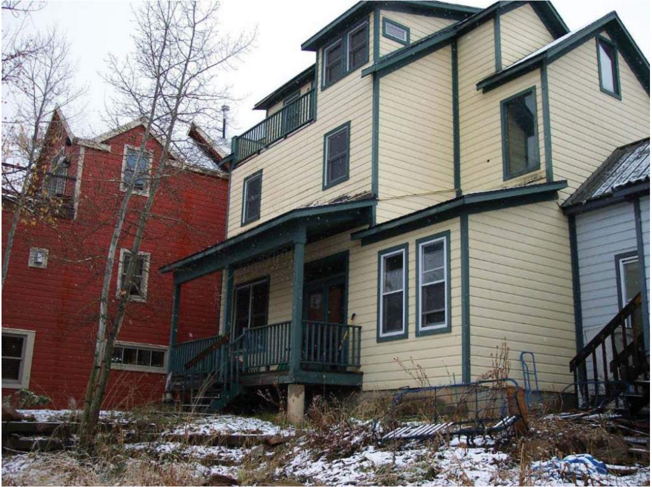
Addition on the south elevation built after 1993
