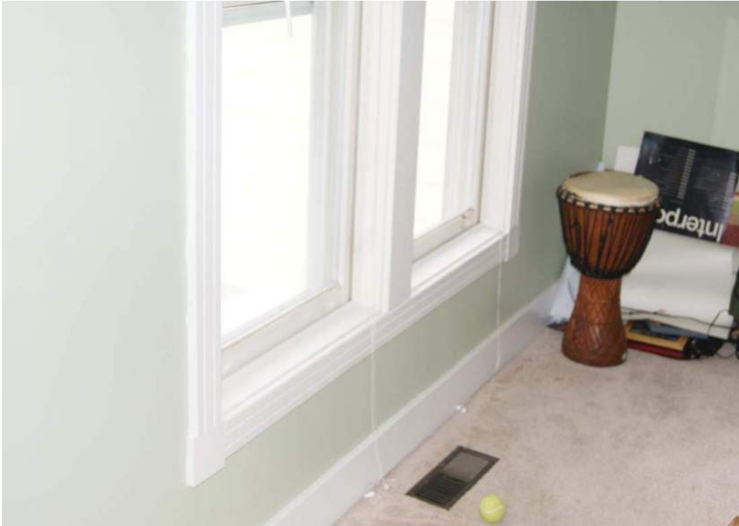
Typical base and window casing
