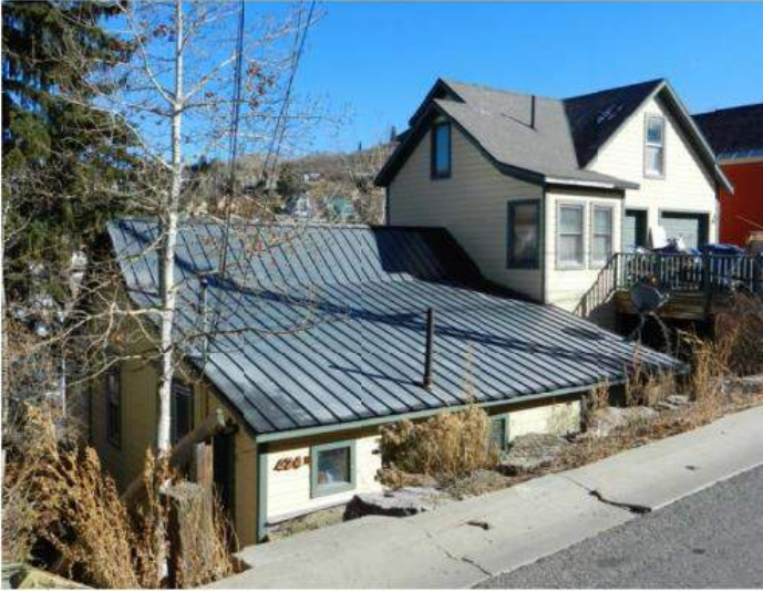
Figure 1: Current Site Orientation – Photographs West Façade
