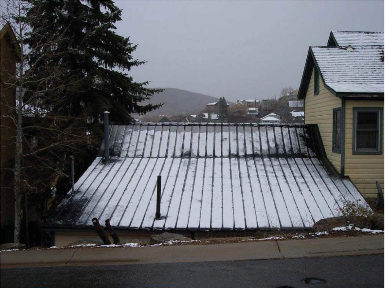
Roof looking east
