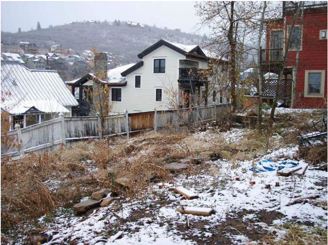
Rear yard fence
