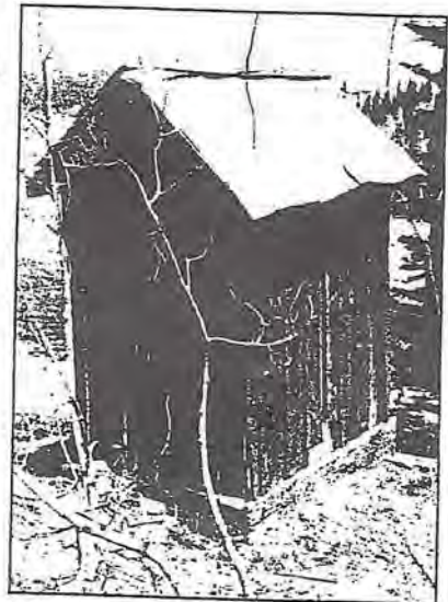
Figure 30 – Another fire shack.
