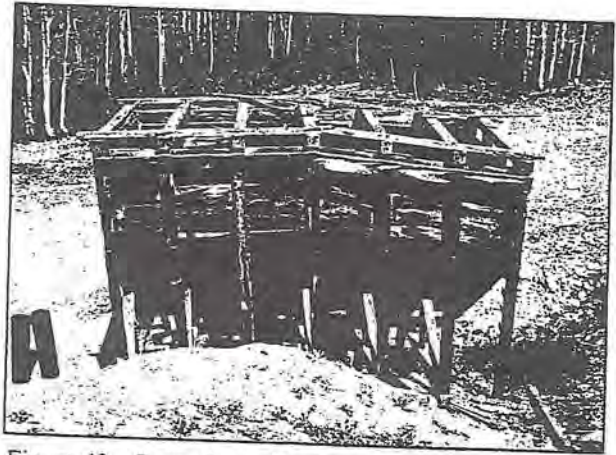
Figure 43 – Rear view, showing sagging corner.
