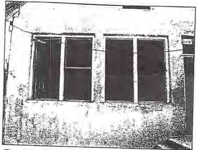
Figure 20 – Window frames in front wall.
