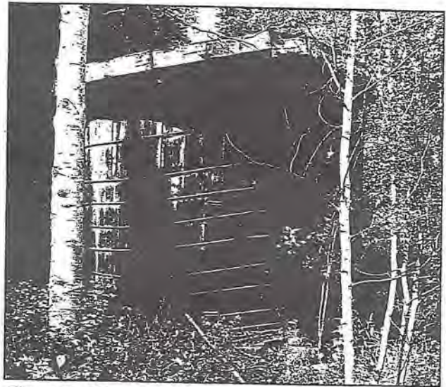
Figure 8 – Water Tank E.
