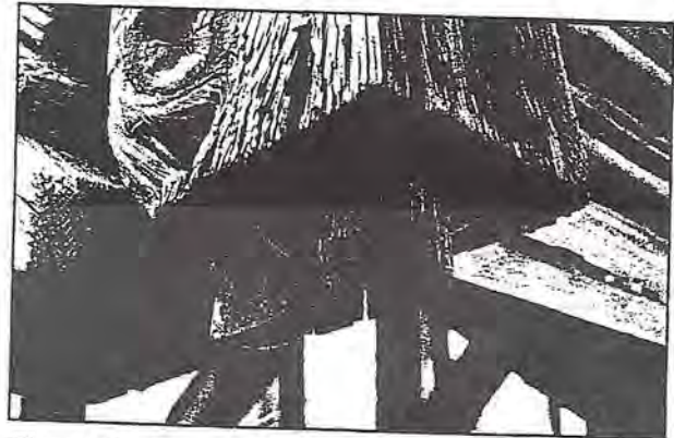
Figure 40 – Tenon of a mortise and tenon joint.
