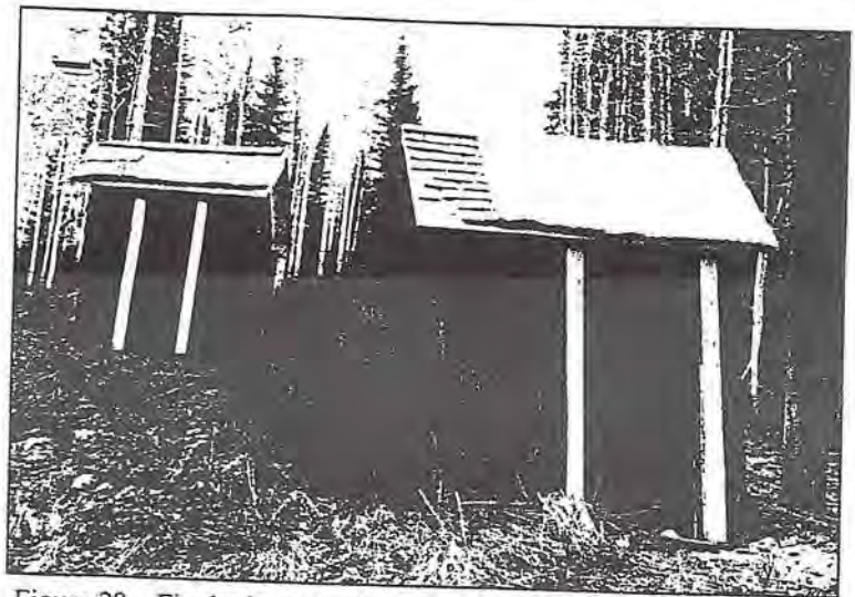
Figure 29 – Fire hydrant shacks at the Daly-West Mine site.
