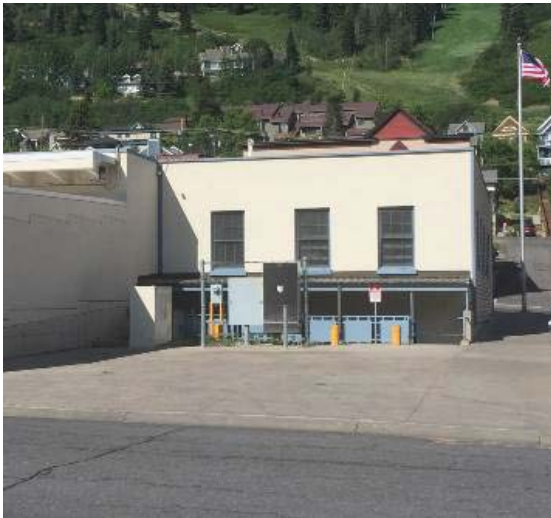
The mechanical equipment behind the Post Office is also not shielded.
