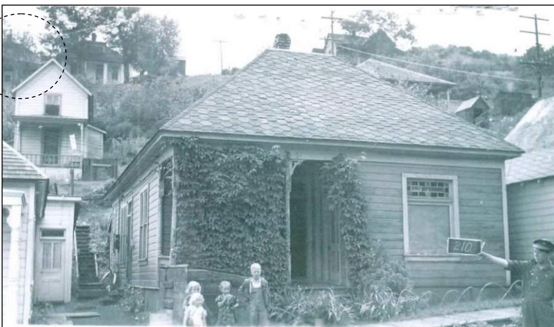
Figure 3: Circa 1940 tax photograph of 412 Marsac Avenue. Facing northeast.
