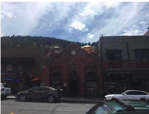
The rooftop addition at No Name at 447 Main Street meets the intent of the Design Guidelines. Because it is setback substantially from the front façade, the addition is not visible from the primary right-of-way, Main Street.
