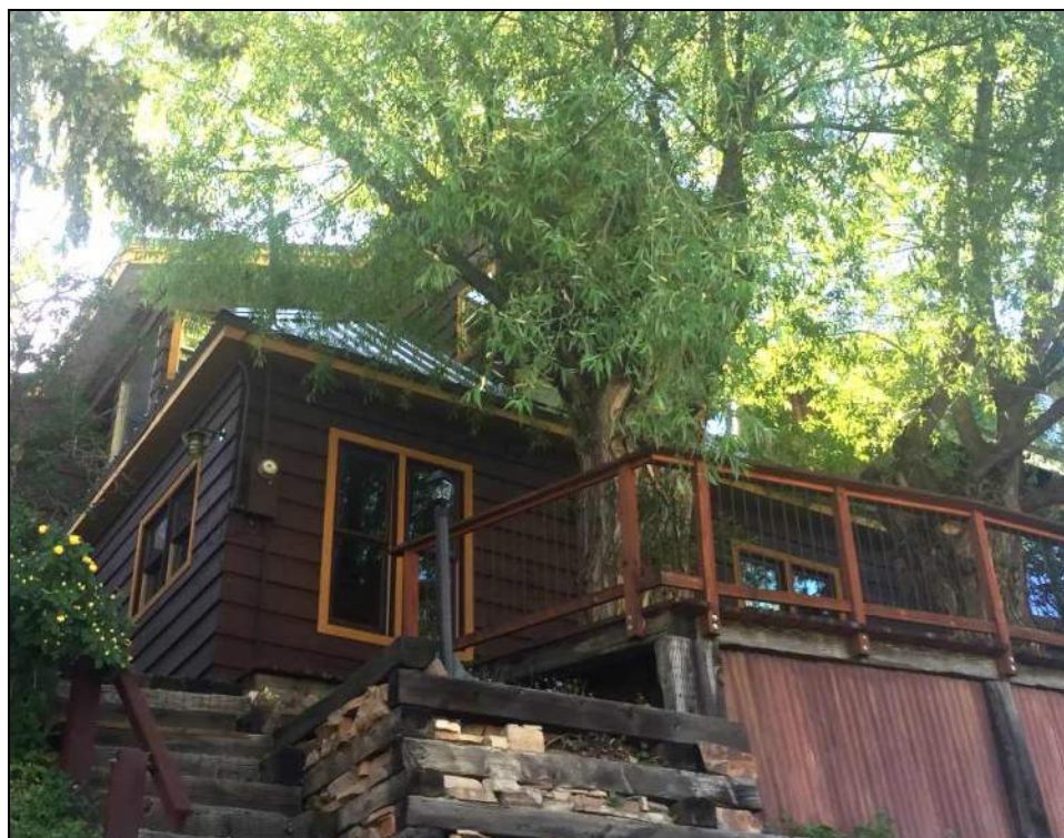
416 Ontario Avenue. Southwest Oblique. June 2016.
