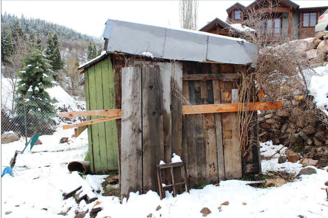
Figure 6. Northwest side of outbuilding, facing southeast. Note square openings cut in vertical plank on right side, providing access for poultry ramps.
