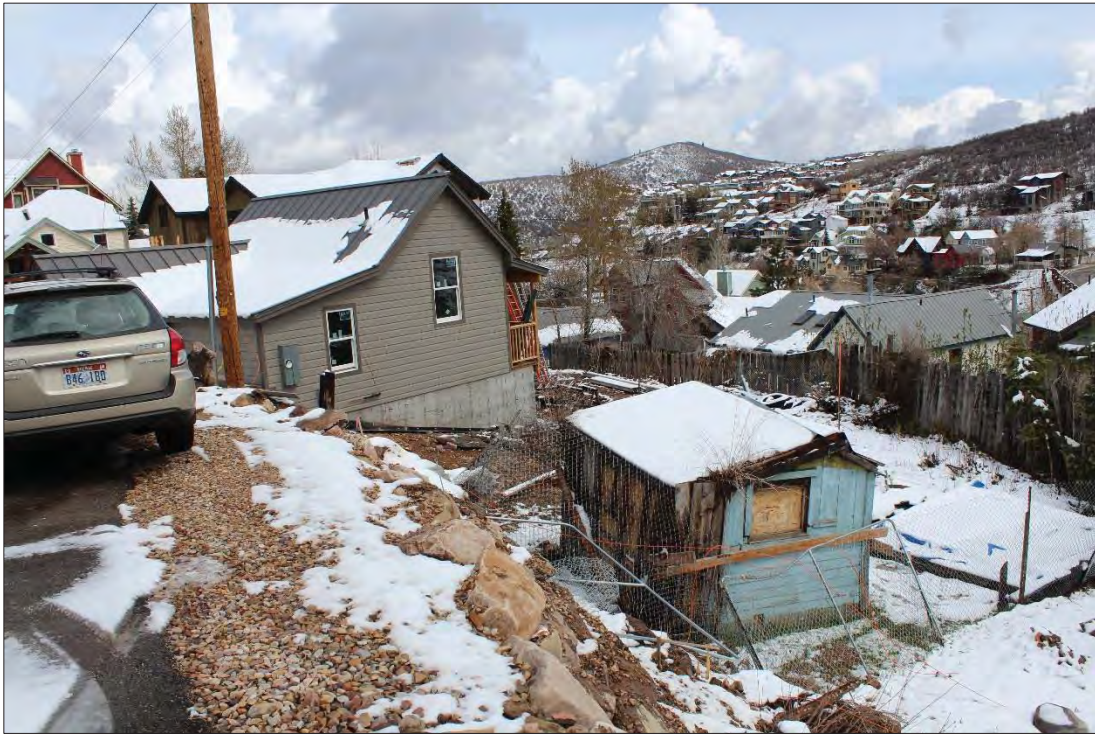
Figure 4. Overview of outbuilding in its present location, facing north.
