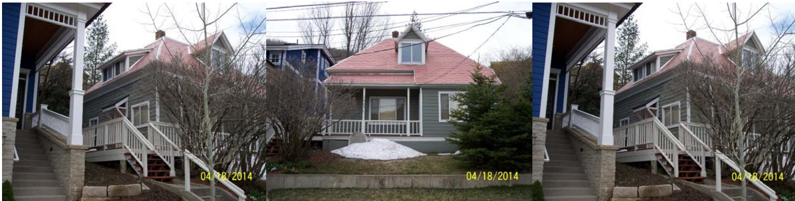
Figure K. Historic chimney located at midpoint of roof
