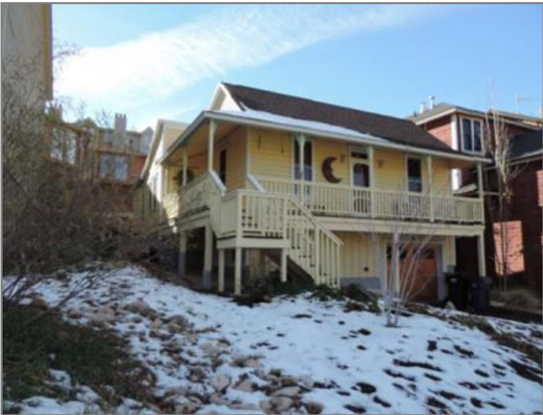
Figure 7: Southeast oblique. Camera facing northwest. November 2014. After the 2002 renovation.
