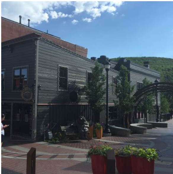
562 Main Street's side elevation faces a pedestrian right-of-way. The applicant provided a small transition to visually separate the new addition from the historic building.
