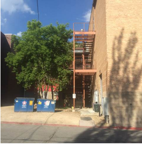
Stairway/fire escape to the south of the Egyptian Theatre on Swede Alley.
