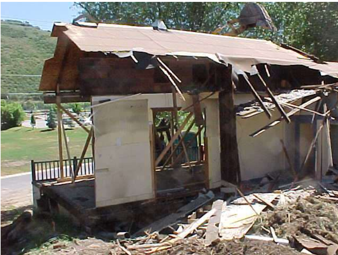
Date of photo: 7/11/2002 Back side of the demolition of the structure.
