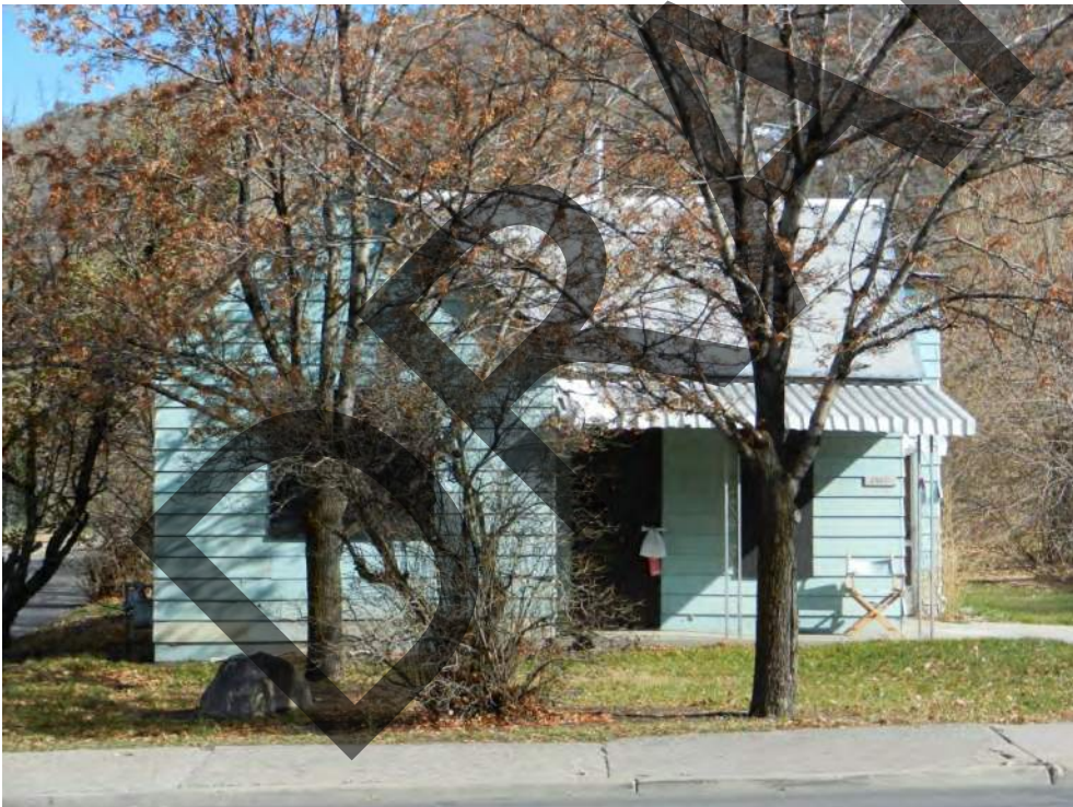
1460 Park Avenue. West elevation. November 2013.
