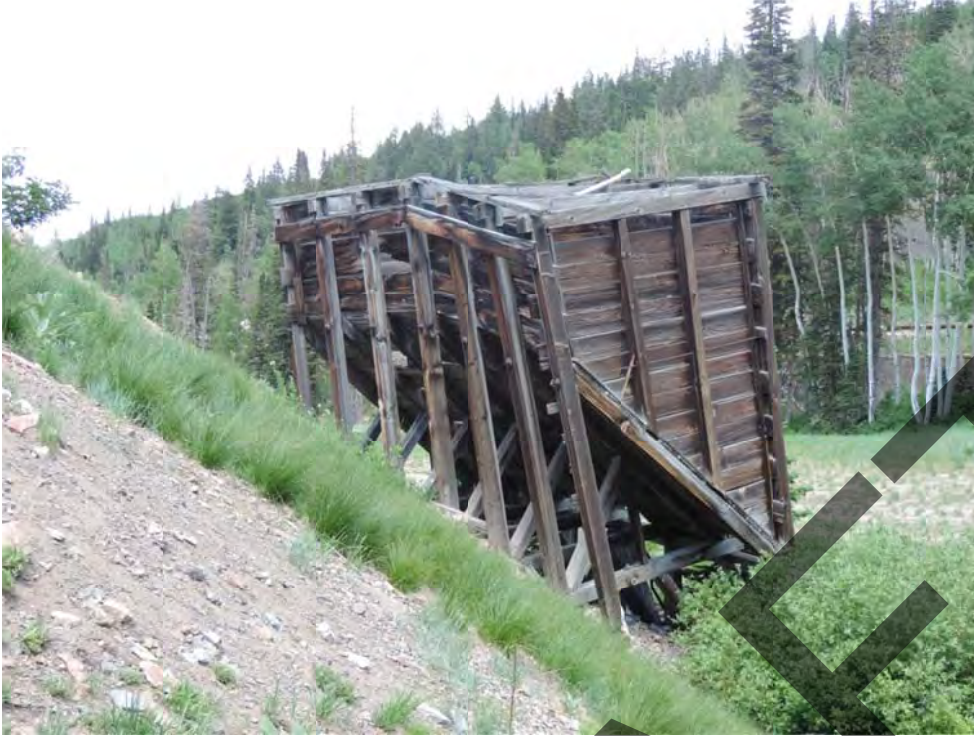
Little Bell Ore Bin. From southwest. June 2016.
