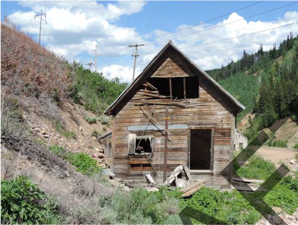
Alliance Tunnel office-dwelling. From west. July 2016.
