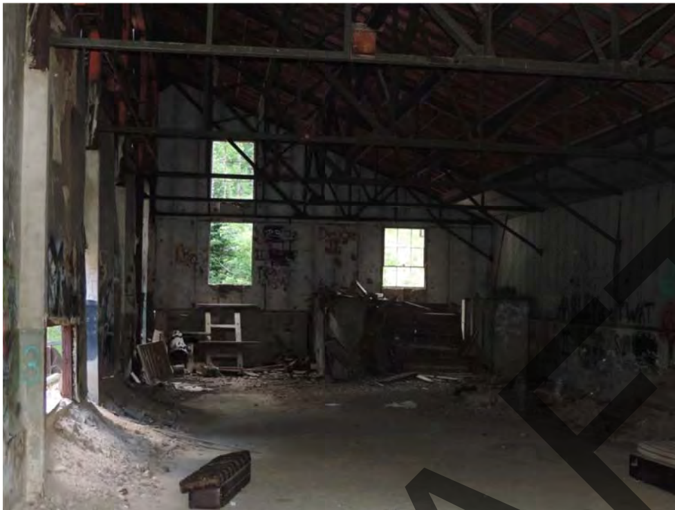
Alliance Tunnel change room interior. From east exterior. July 2016.
