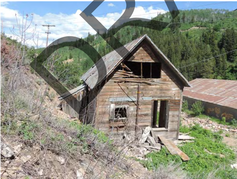
Alliance Tunnel office-dwelling. From northwest. July 2016.
