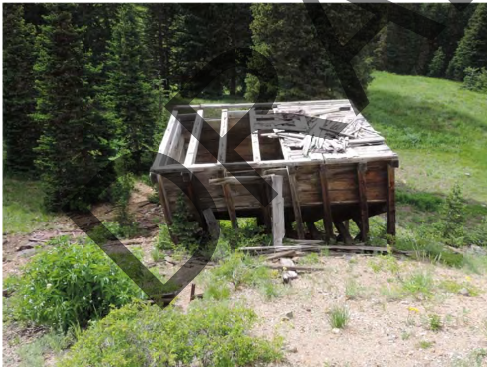
Jupiter Mine Ore Bin. From southeast. July 2016.
