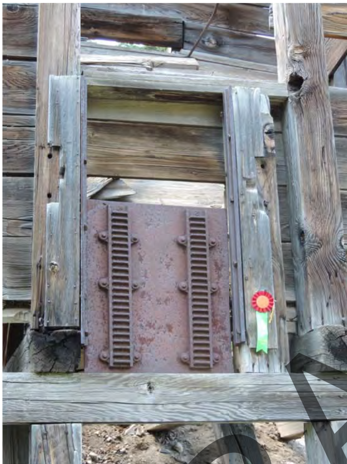
Little Bell Ore Bin, chute detail. From east. June 2016.
