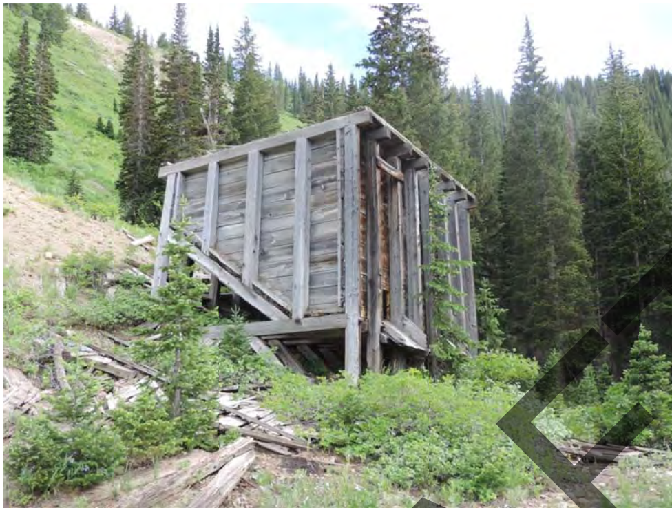
Jupiter Mine Ore Bin. From north. July 2016.
