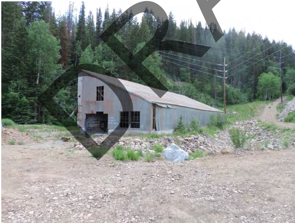
Alliance Tunnel change room. From northeast. July 2016.
