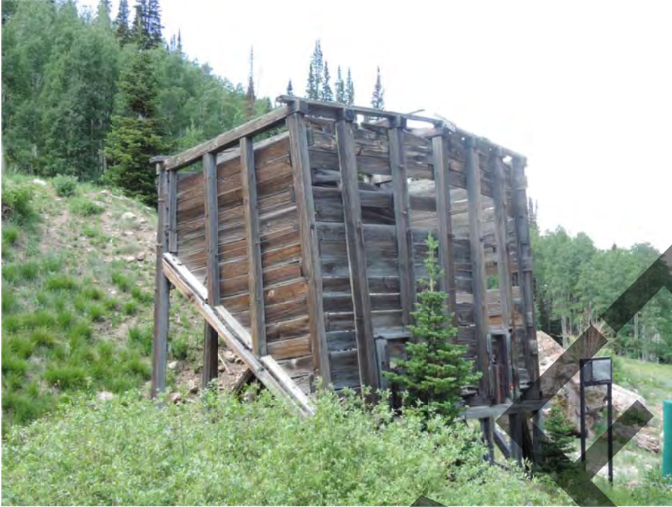
Little Bell Ore Bin. From southeast. June 2016.
