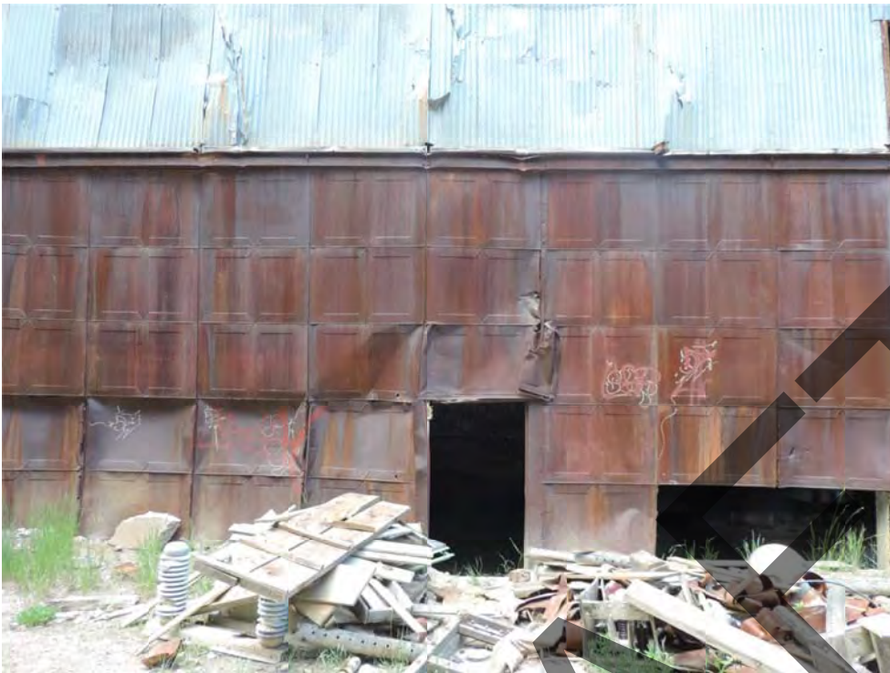
Alliance Tunnel change room. From south. July 2016.
