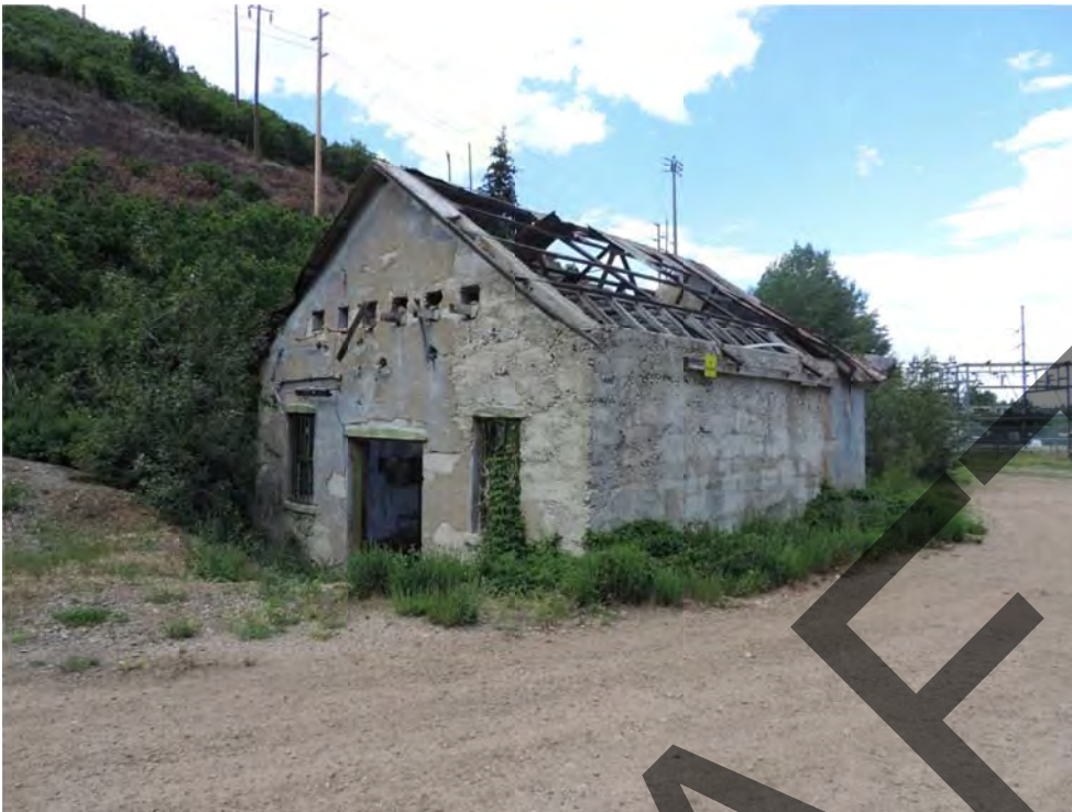
Alliance Tunnel pump house. From south. July 2016.
