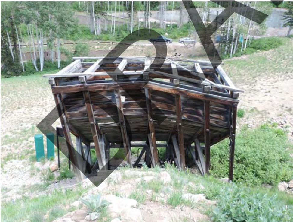
Little Bell Ore Bin. From west. June 2016.
