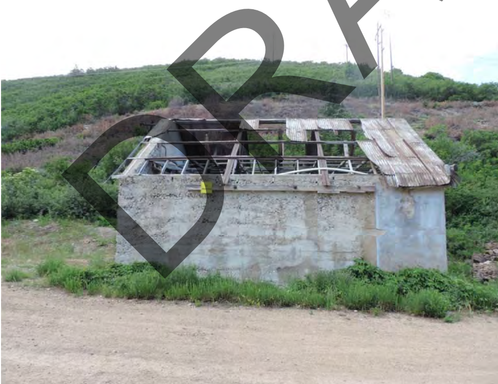
Alliance Tunnel pump house. From southeast. July 2016.
