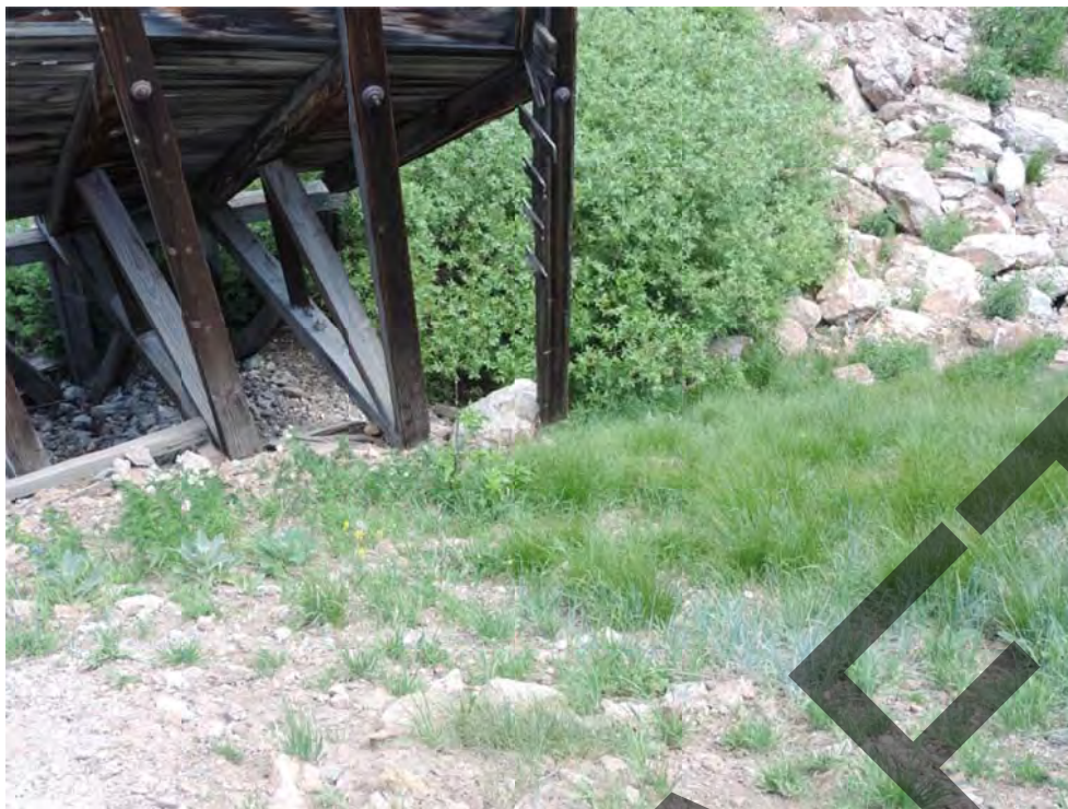
Little Bell Ore Bin, structural detail. From northwest. June 2016.
