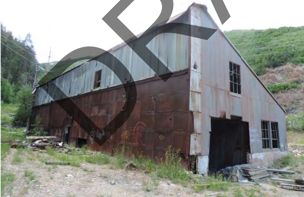
Alliance Tunnel change room. From southeast. July 2016.
