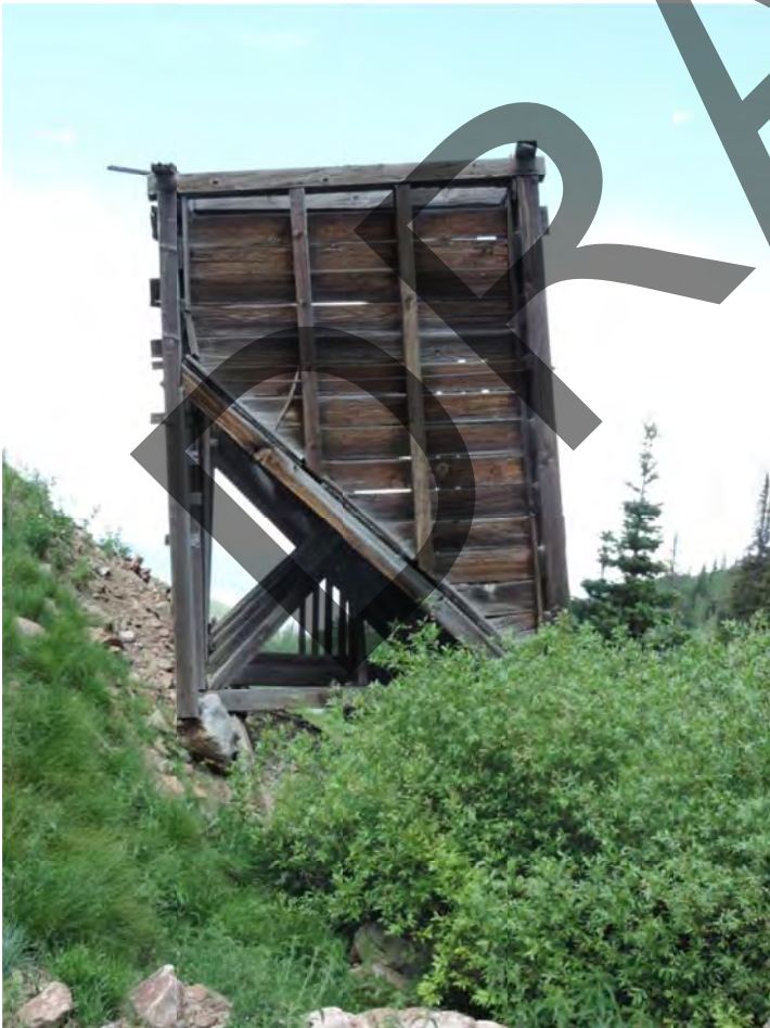
Little Bell Ore Bin. From south. June 2016.
