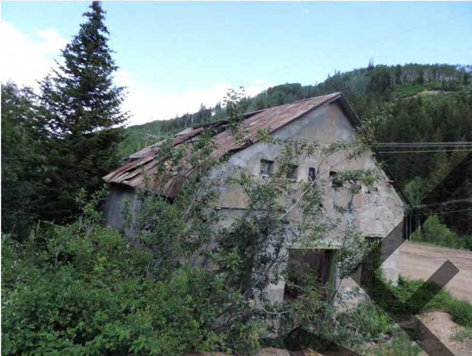
Alliance Tunnel pump house. From west. July 2016.
