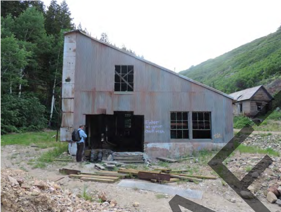
Alliance Tunnel change room. From east. July 2016.
