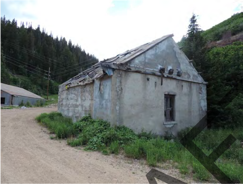
Alliance Tunnel pump house. From east. July 2016.
