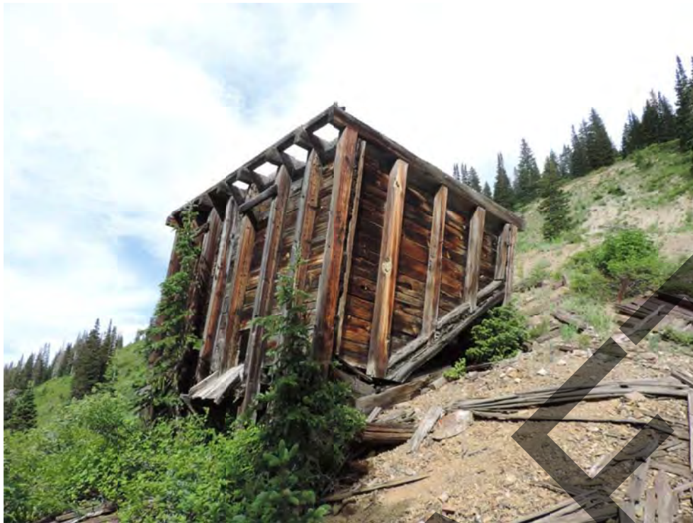
Jupiter Mine Ore Bin. From west. July 2016.
