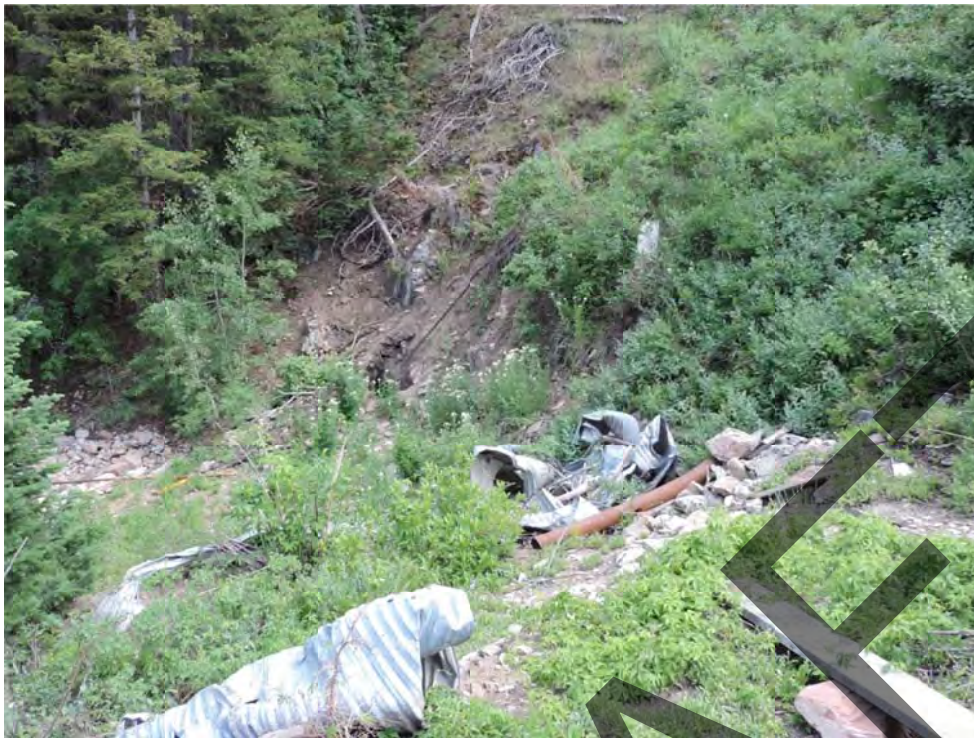
Alliance Tunnel site, former tunnel entrance location. From east. July 2016.
