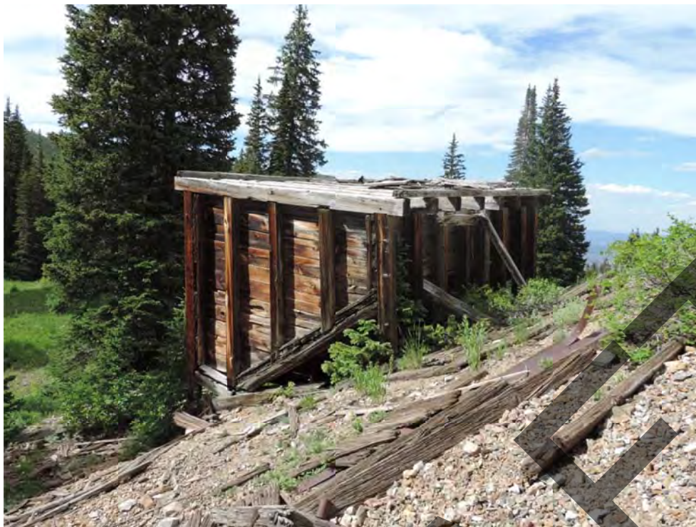
Jupiter Mine Ore Bin. From south. July 2016.
