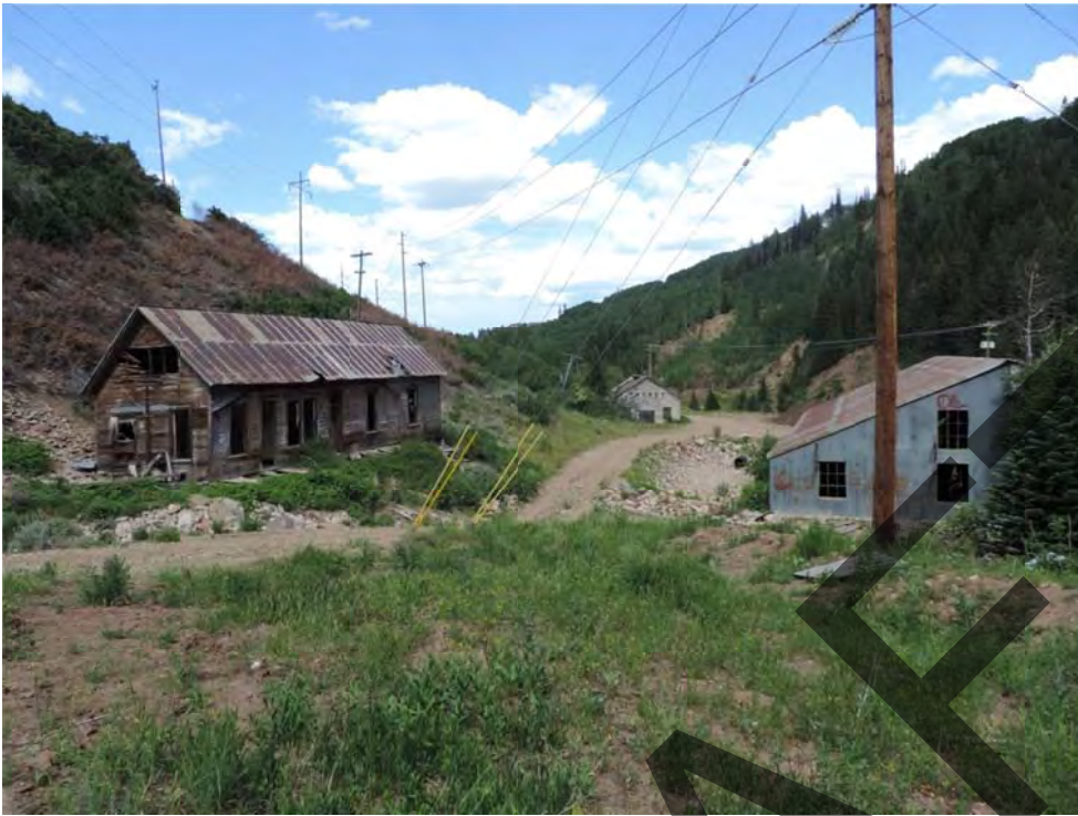
Alliance Tunnel Site. Office-Dwelling left foreground. Change room right foreground. Pump house center background. From west. July 2016.
