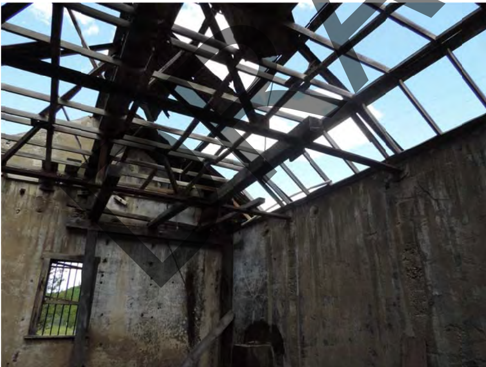
Alliance Tunnel pump house, ceiling detail. From southwest exterior. July 2016.
