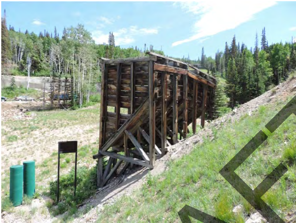
Little Bell Ore Bin. From northwest. June 2016.
