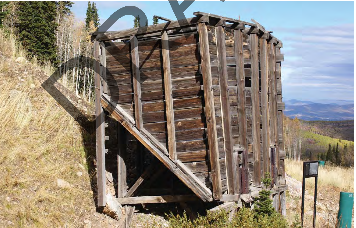
Little Bell Ore Bin, southeast oblique, 2009 (photo: Preservation Solutions)
