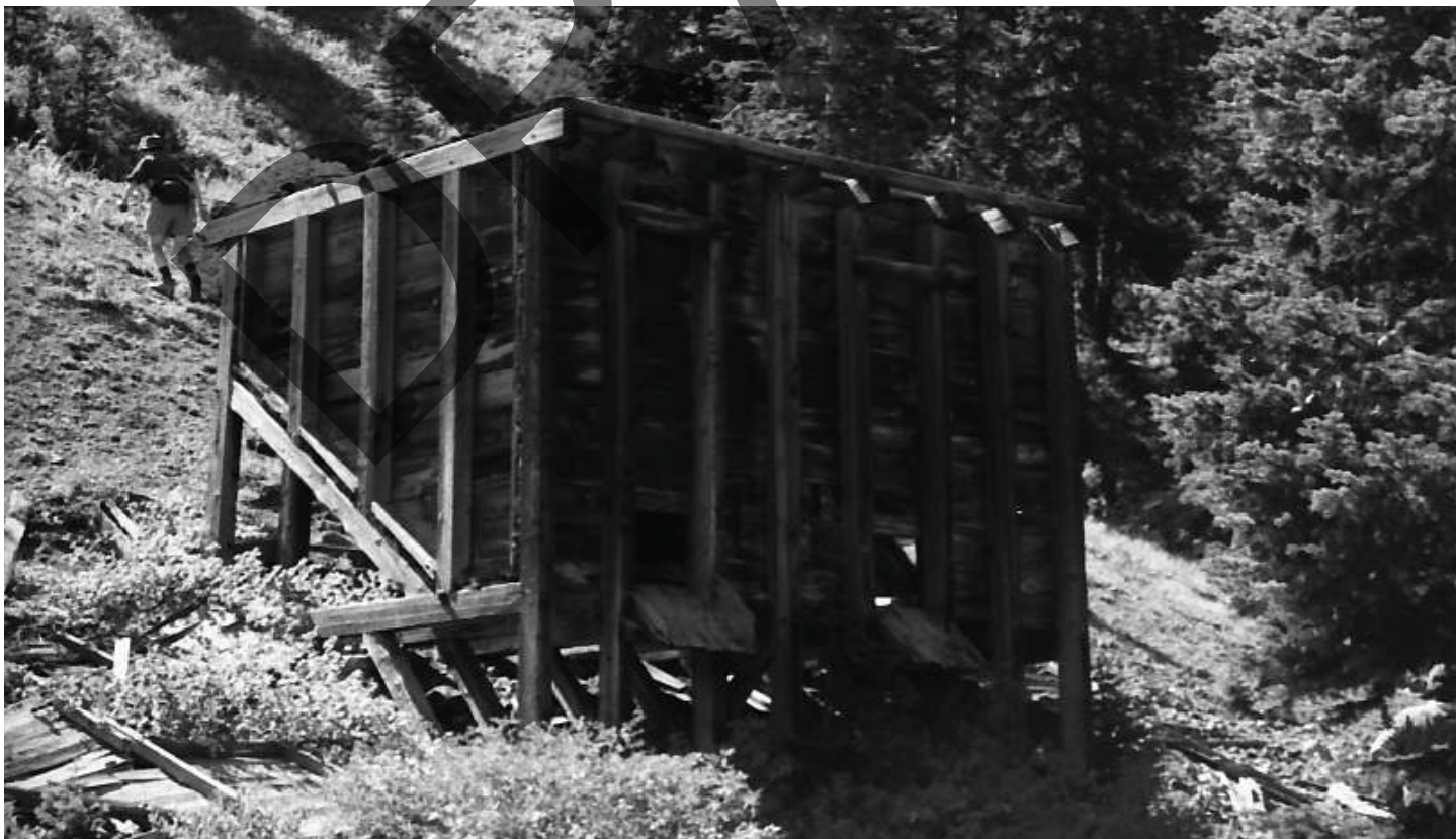
Jupiter Mine Ore Bin, south oblique, 1999 (photo: Sandra Morrison)
