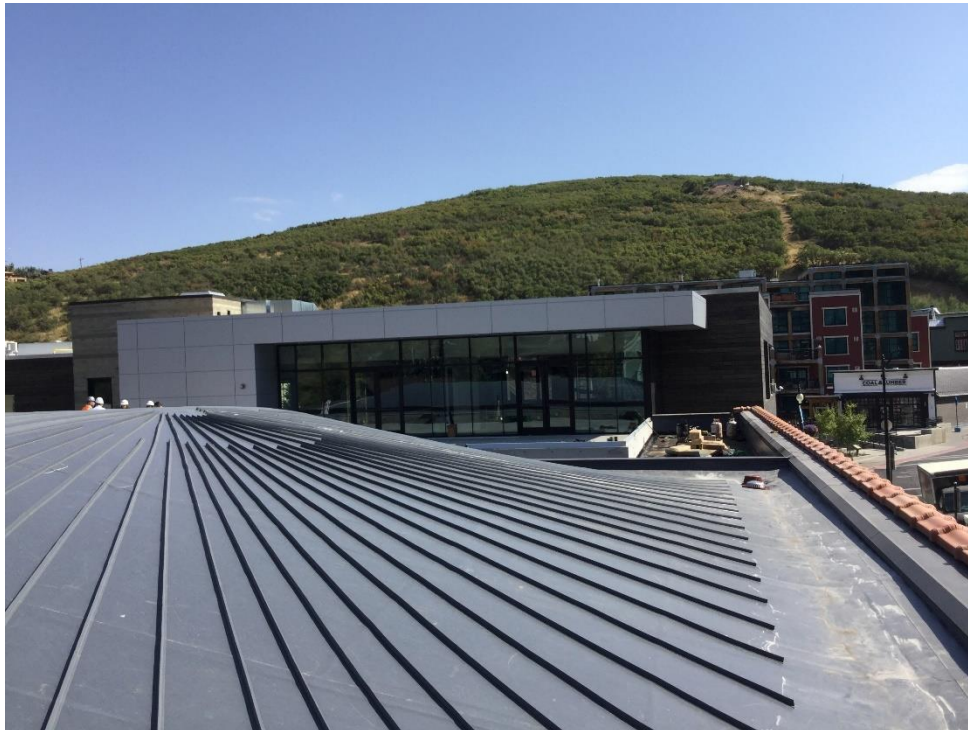
Figure 1: Collaboration of Kimball Building team from measurement location 1 (refer to Figure 2 for measurements locations)
