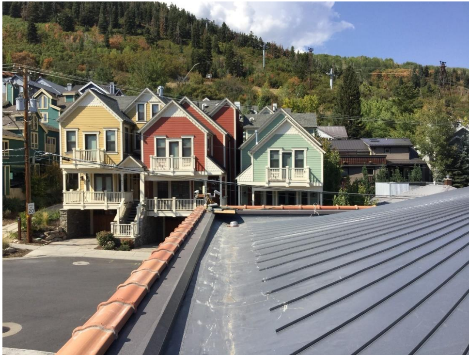
Figure 3: Measurement Location on Kimball Building Rooftop
