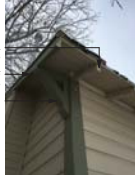
(2) 2x4 INTERNAL OUTRIGGERS 2x6 OUTRIGGER @ ROOF ENDS ORNAMENTAL OUTRIGGER - SEE BELOW
