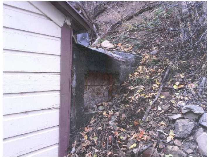
Photo of north elevation. The root cellar is the concrete structure built into the hill.
