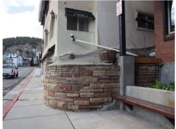
Retaining Wall #2 (North Side of Façade)
