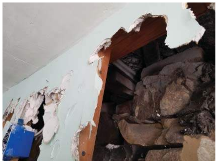
57 - L0 - S. side of Central Stone Wall
