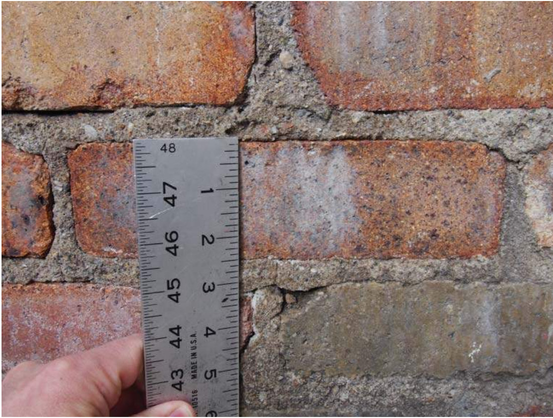
29 - Chimney Brick Height
