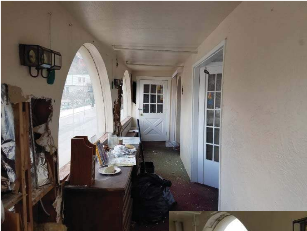
64 - L1 - Entry Looking South
