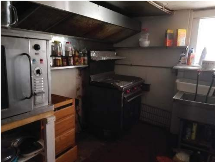
71 - L1 - Kitchen - NW Wall
