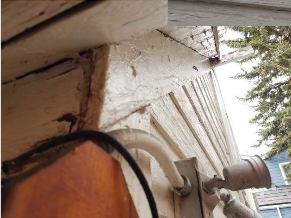
24 - NW Eave Detail
