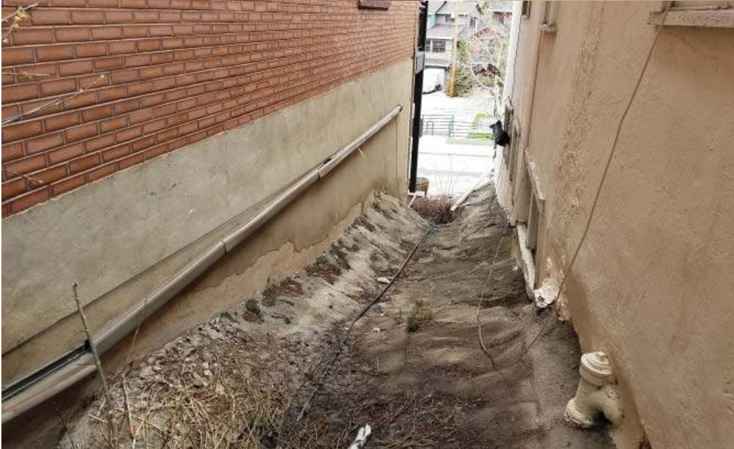
10 - North Concrete Site Detail
