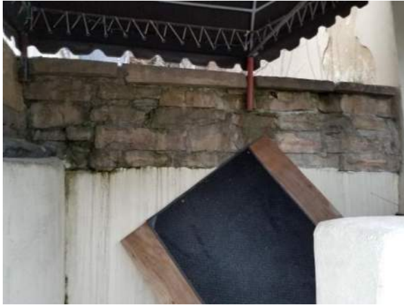
Retaining Wall #1 (South Side of Façade)
