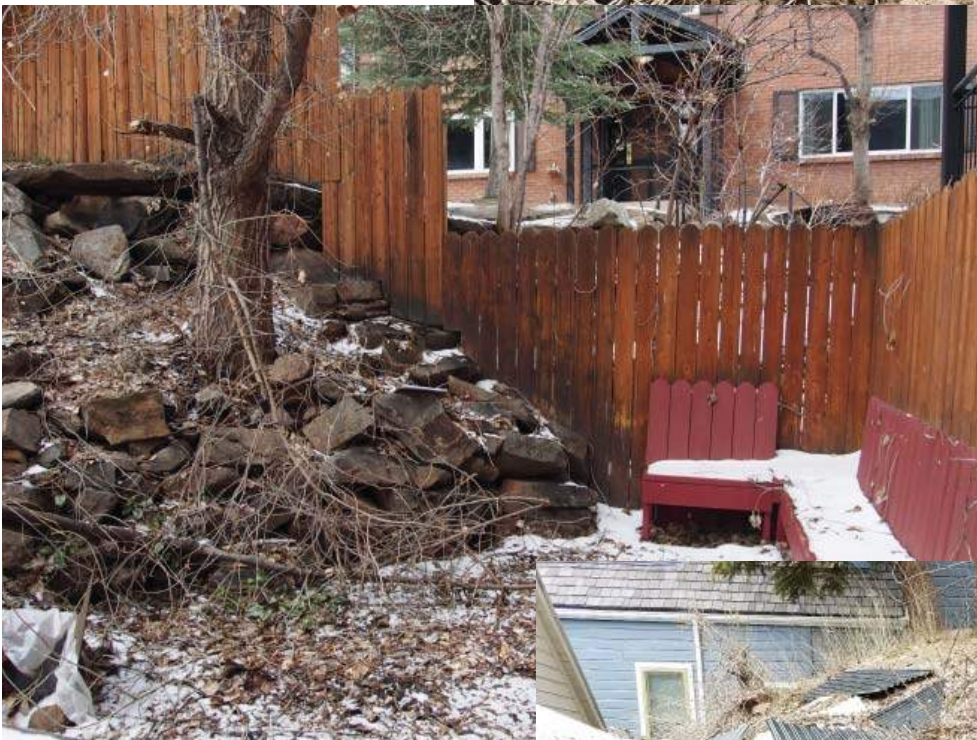
17 - West Deck & Retaining Wall
