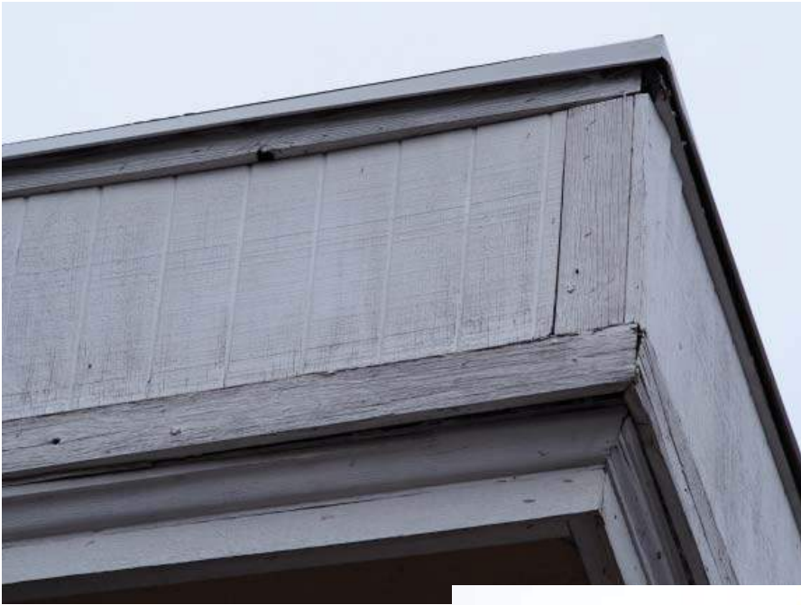
19 - East Eave Detail
