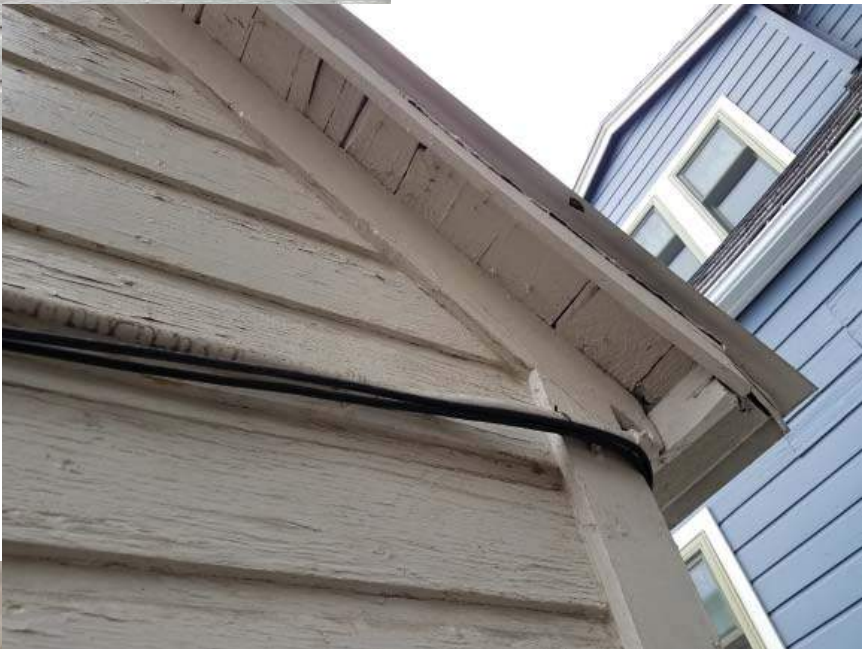
23 - SW Eave Detail
