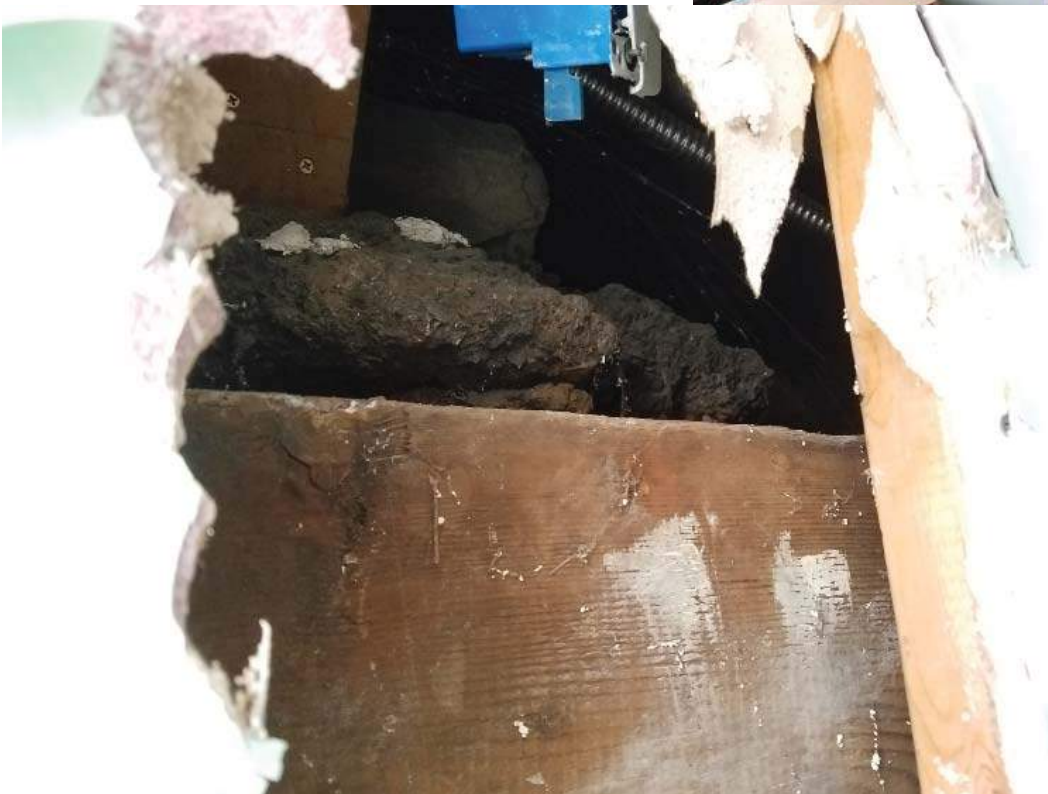
53 - L0 - Retail South Wall Detail
