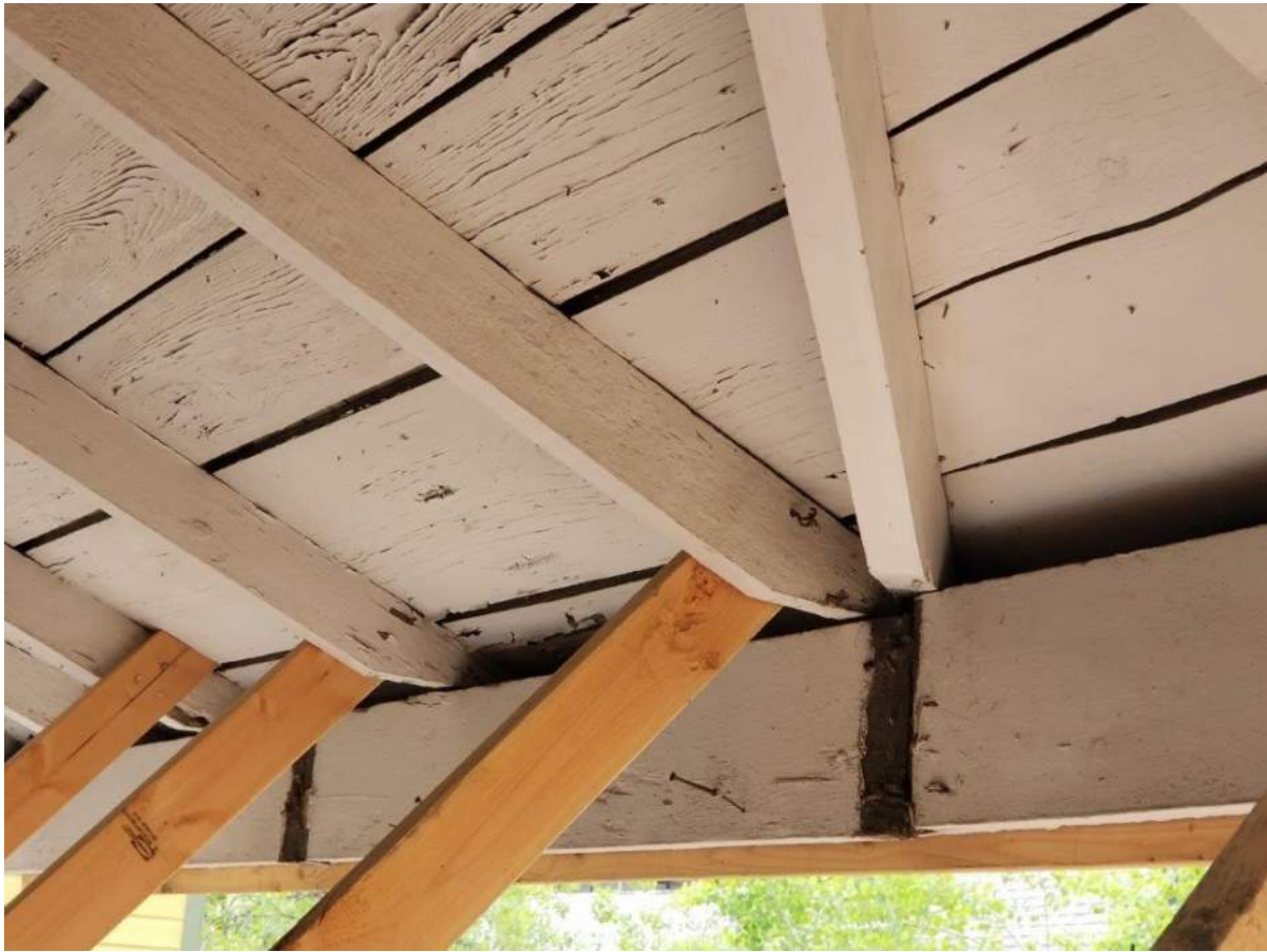
Above: Porch roof.
