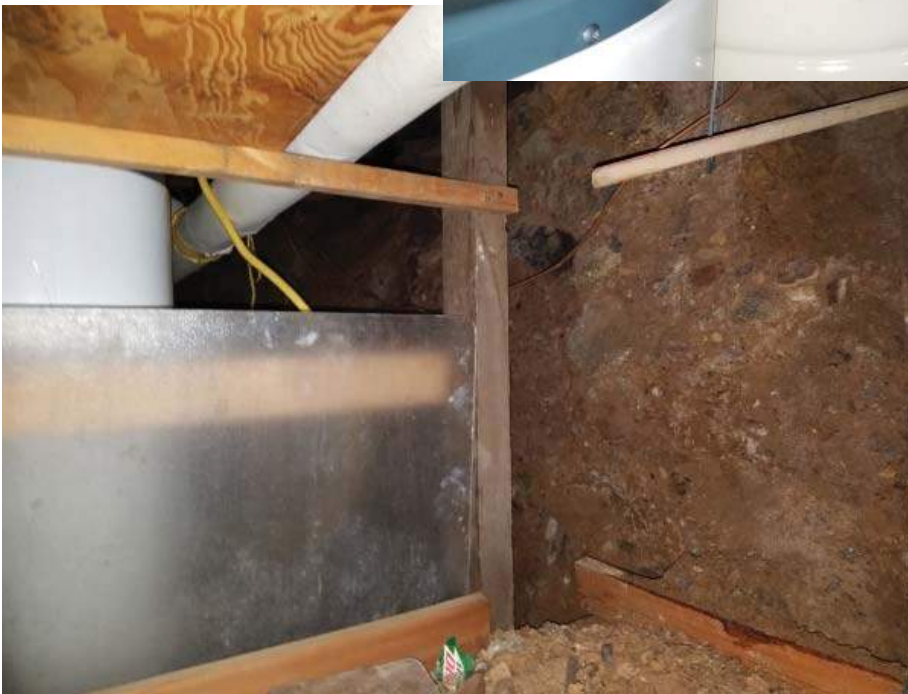
60 - L0 - Dirt Foundation
