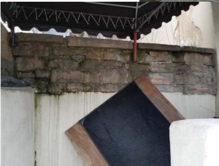
27 - East Retaining Wall
