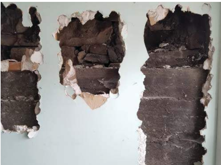
56 - L0 - Detail of Wall
