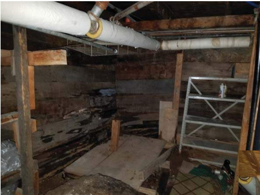
61 - L0 - Wood Shoring
