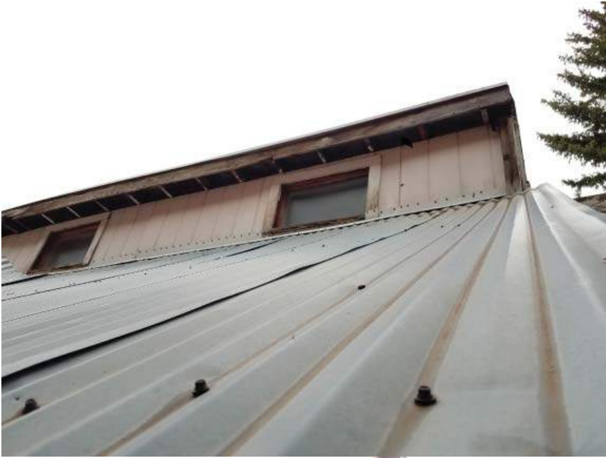
8 - North Corrugated Roofing
