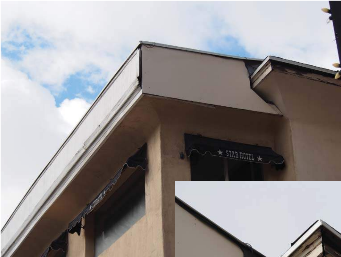
31 - NE Eave Detail
