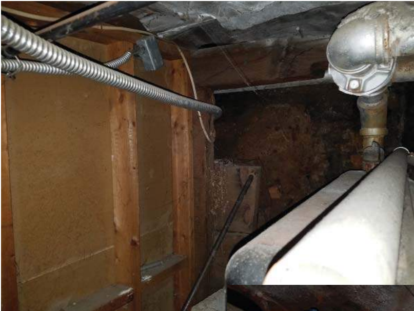
58 - L0 - South Foundation in Mech.
