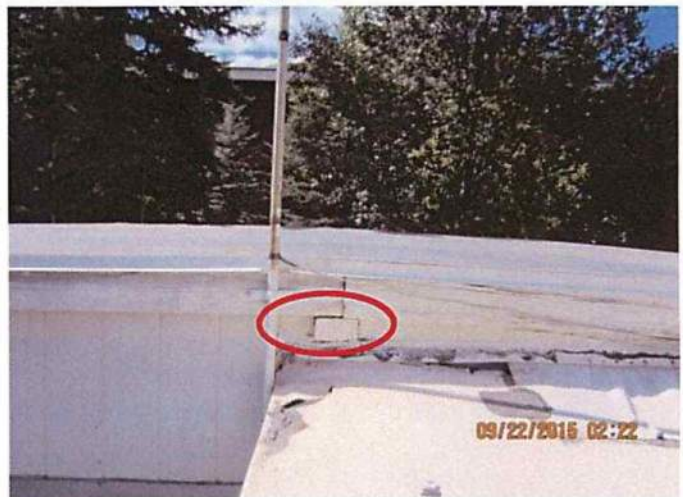
Photo 8 Note structural beam. Refer to photo 9
