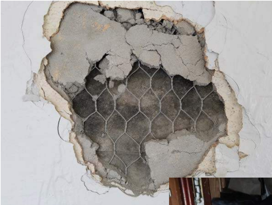
80 - L1 - Stucco Assembly Inside Wall of Entry
