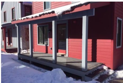
Figure 3: The Retreat at the Park, 8 single family homes built in 2017
