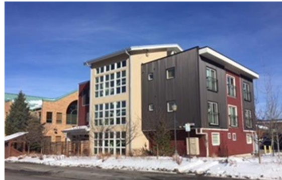
Figure 2: Transit Housing, 13 studios built by the city with a grant from the Federal Transportation Administration in 2013
