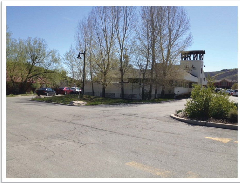
Figure 2a – on site project west elevation
