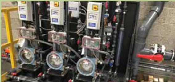
Chlorine-feed pumps
