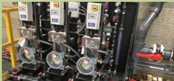
Chlorine-feed pumps
