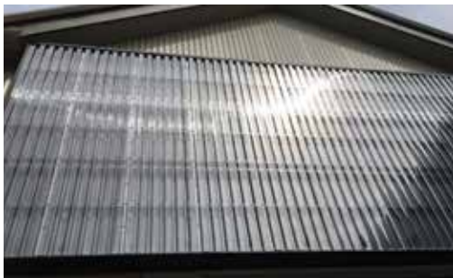
South-facing solar wall
