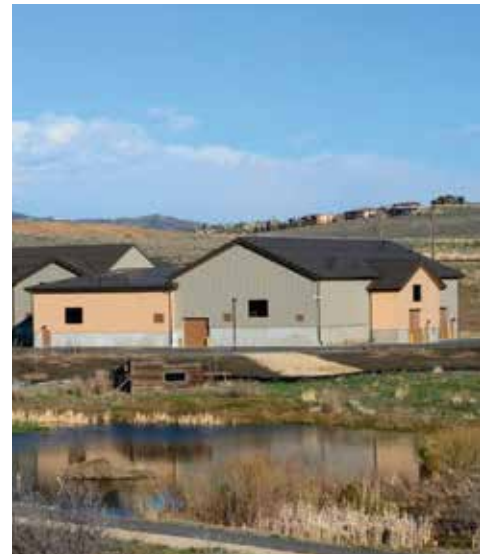
Quinns Junction WTP
