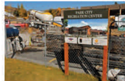
Progress on Recreation Center
