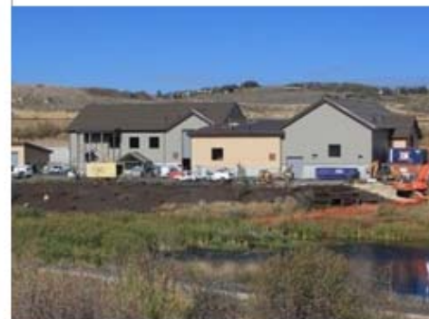
Quinn's Junction Water Treatment Plant
