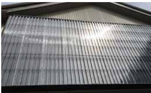
South-facing solar wall
