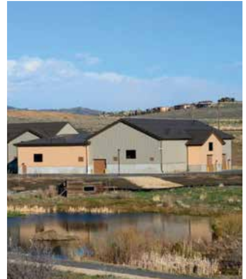
Quinns Junction WTP
