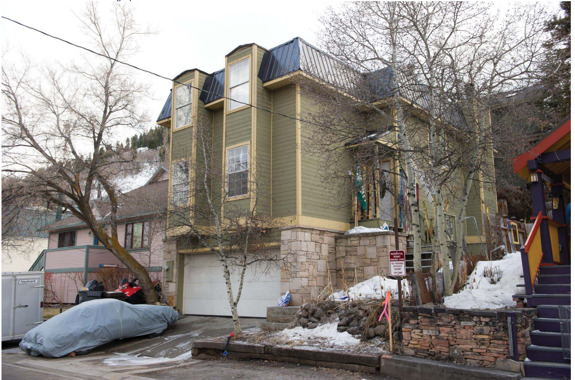
813 Woodside Avenue - looking southerly
