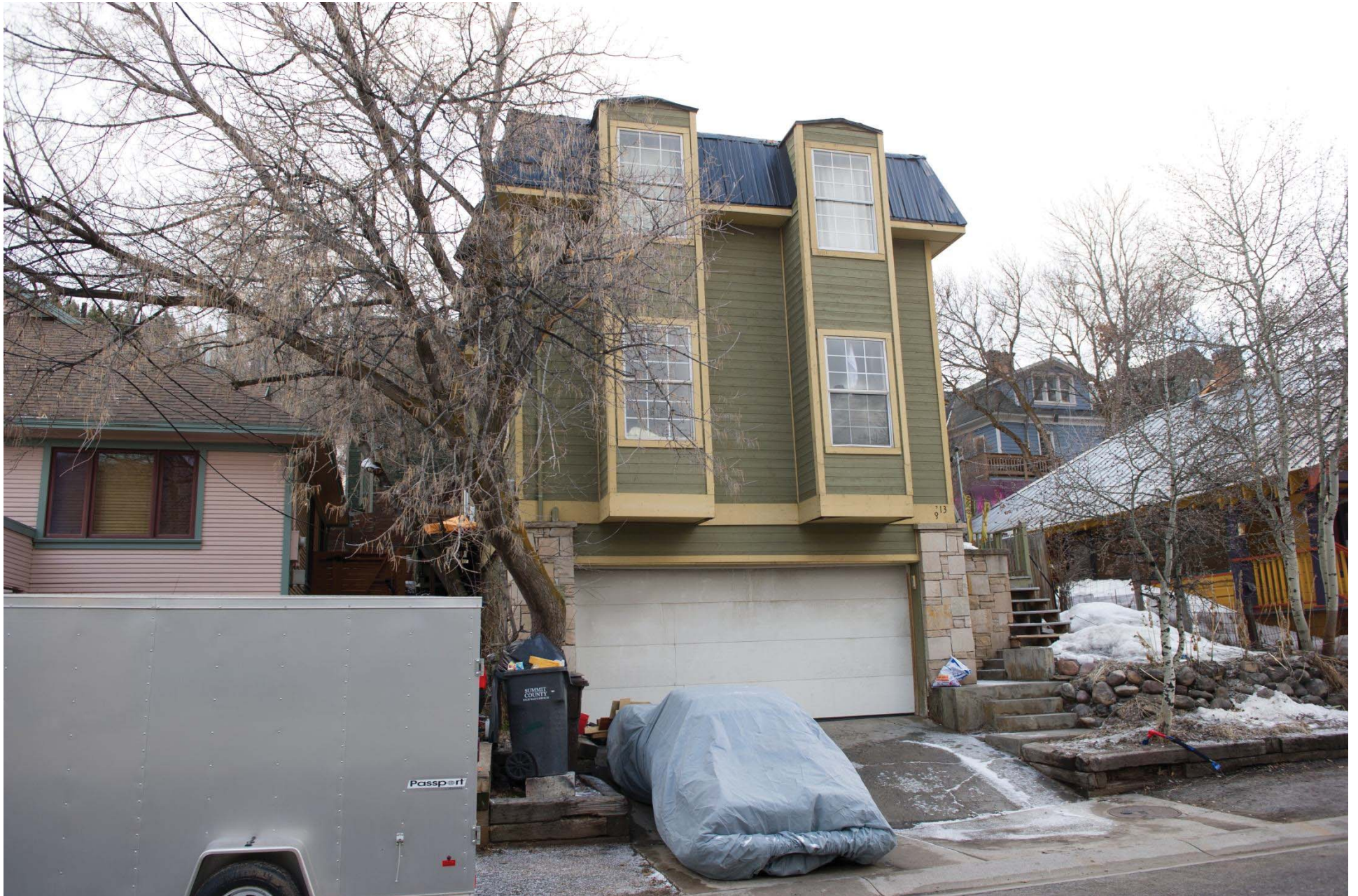
813 Woodside Avenue - looking westerly
