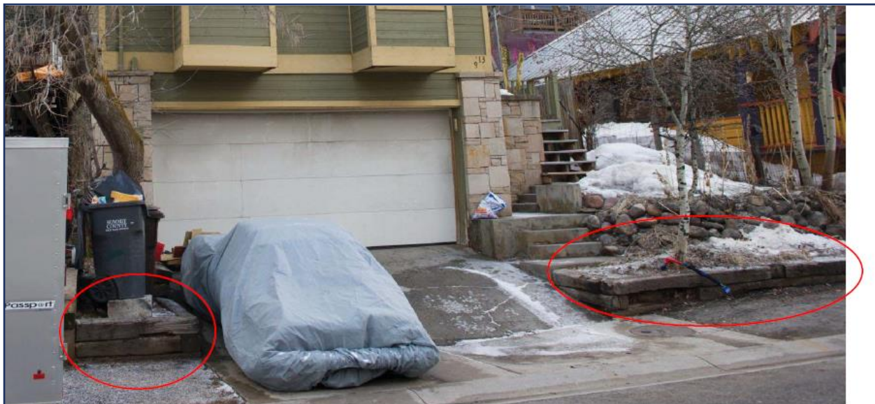
813 Woodside Avenue - looking westerly
