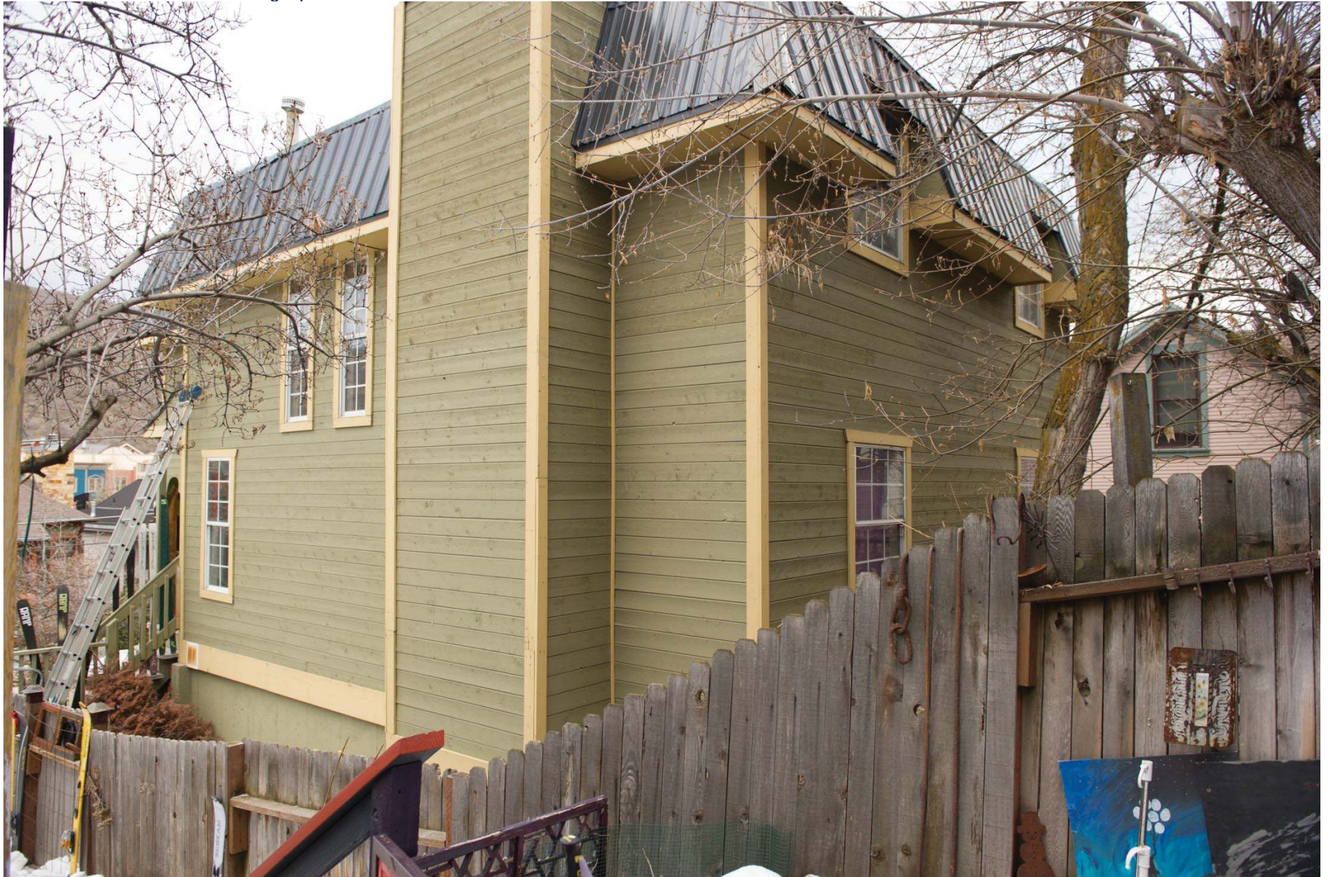
813 Woodside Avenue - looking easterly
