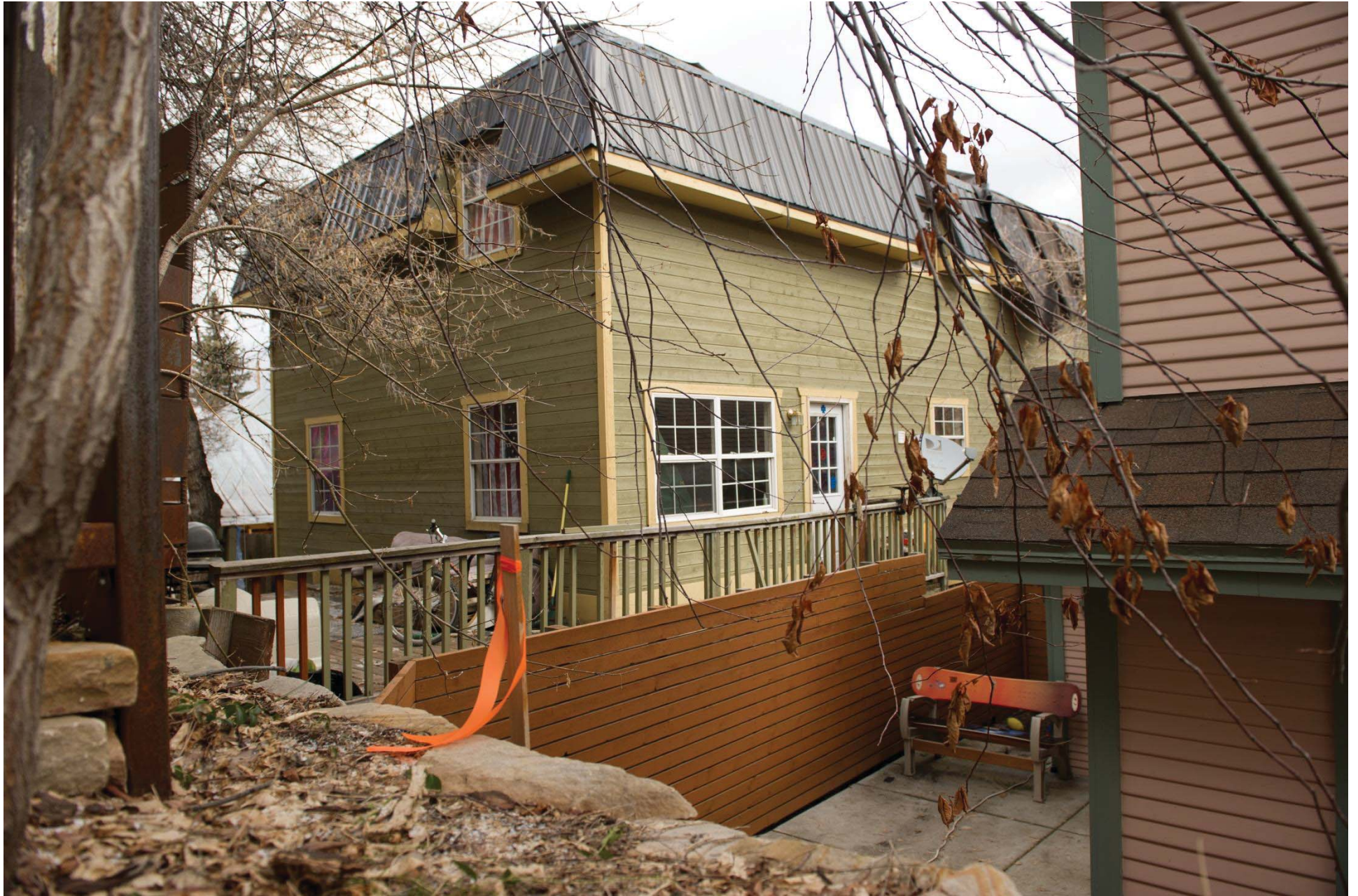
813 Woodside Avenue - looking to the north
