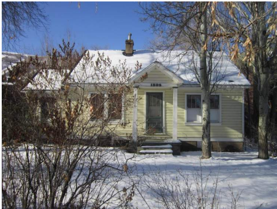
1503 Park Avenue. East elevation. November 2013.
