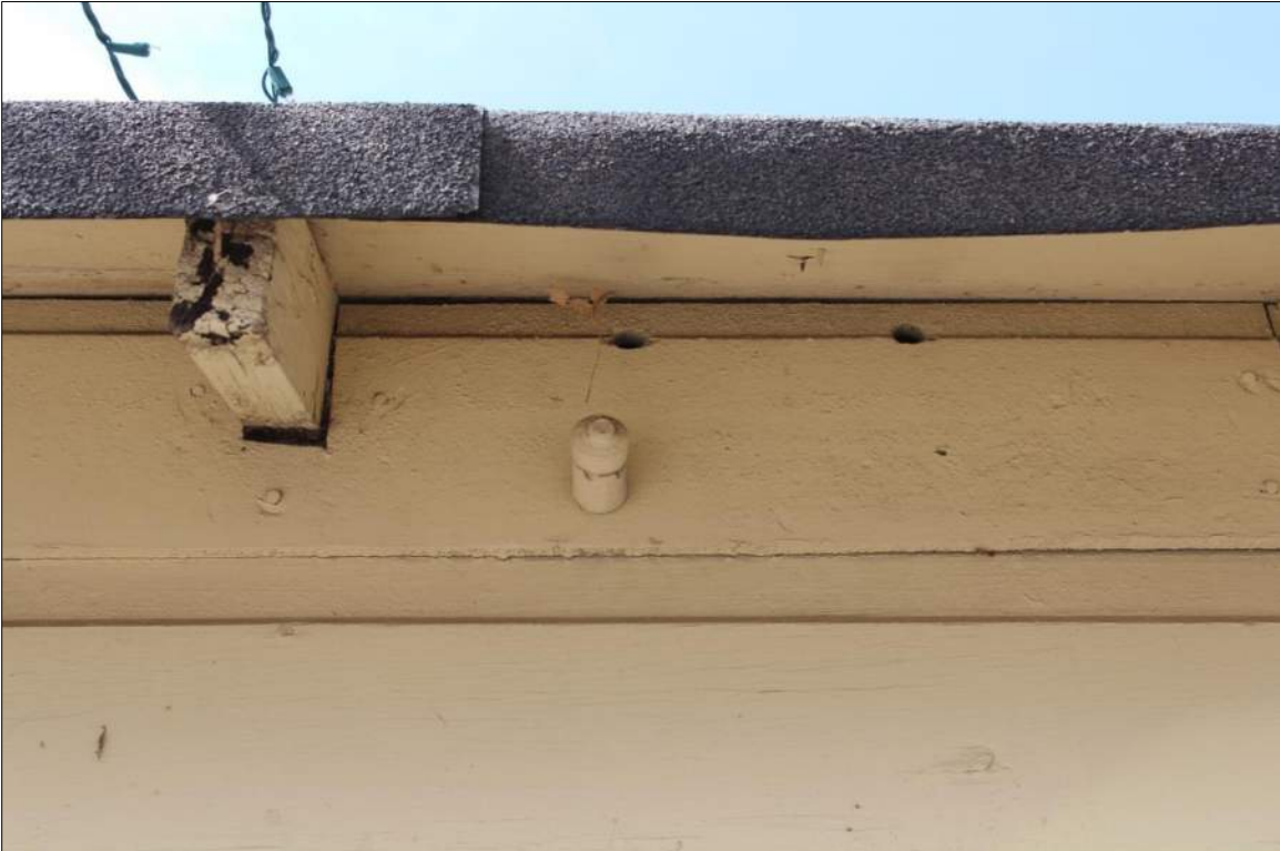
Figure 8. Porcelain knob under east eave of garage at 1503 Park Avenue, 2018, view facing west.
