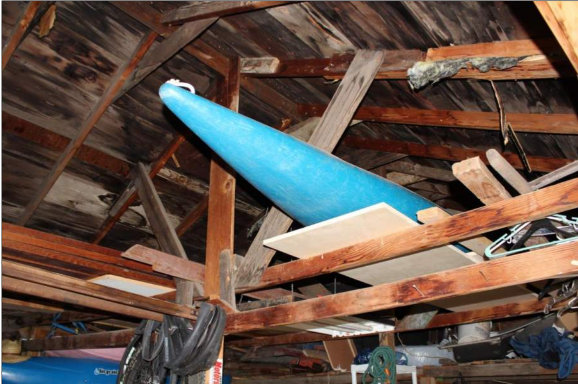
Figure 10. Roof framing system of garage at 1503 Park Avenue, 2018, view facing northwest.
