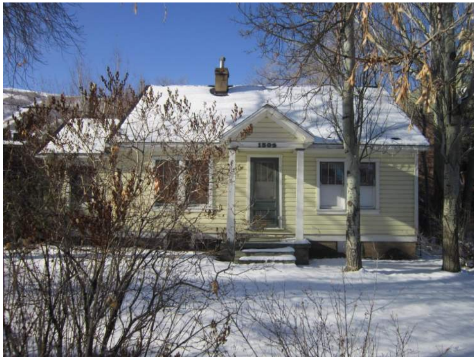
1503 Park Avenue. East elevation. November 2013.
