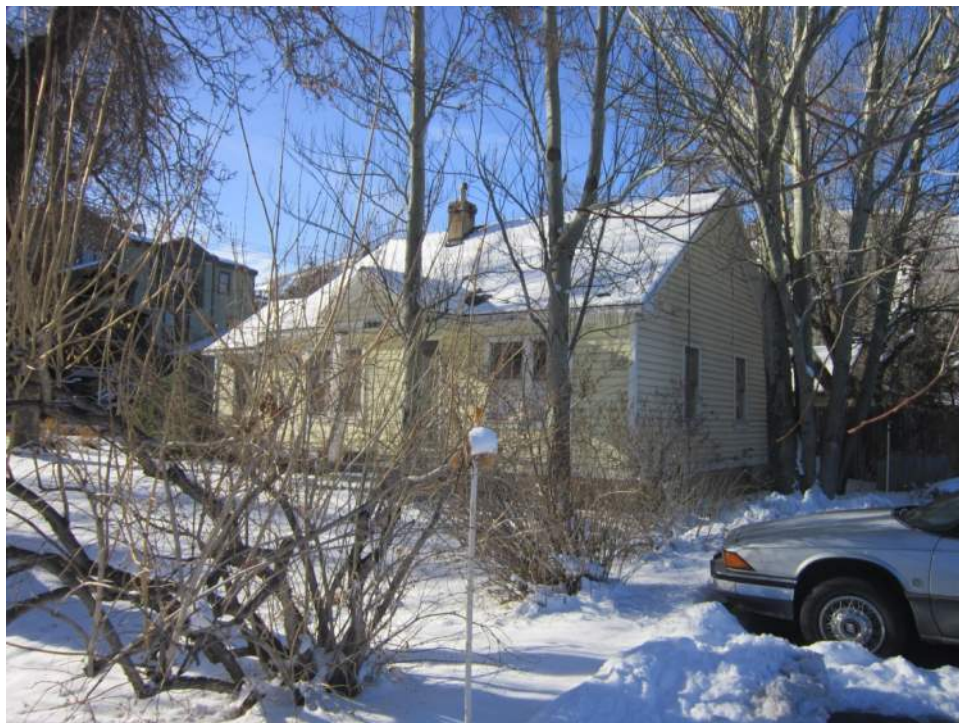
1503 Park Avenue. Northeast oblique. November 2013.
