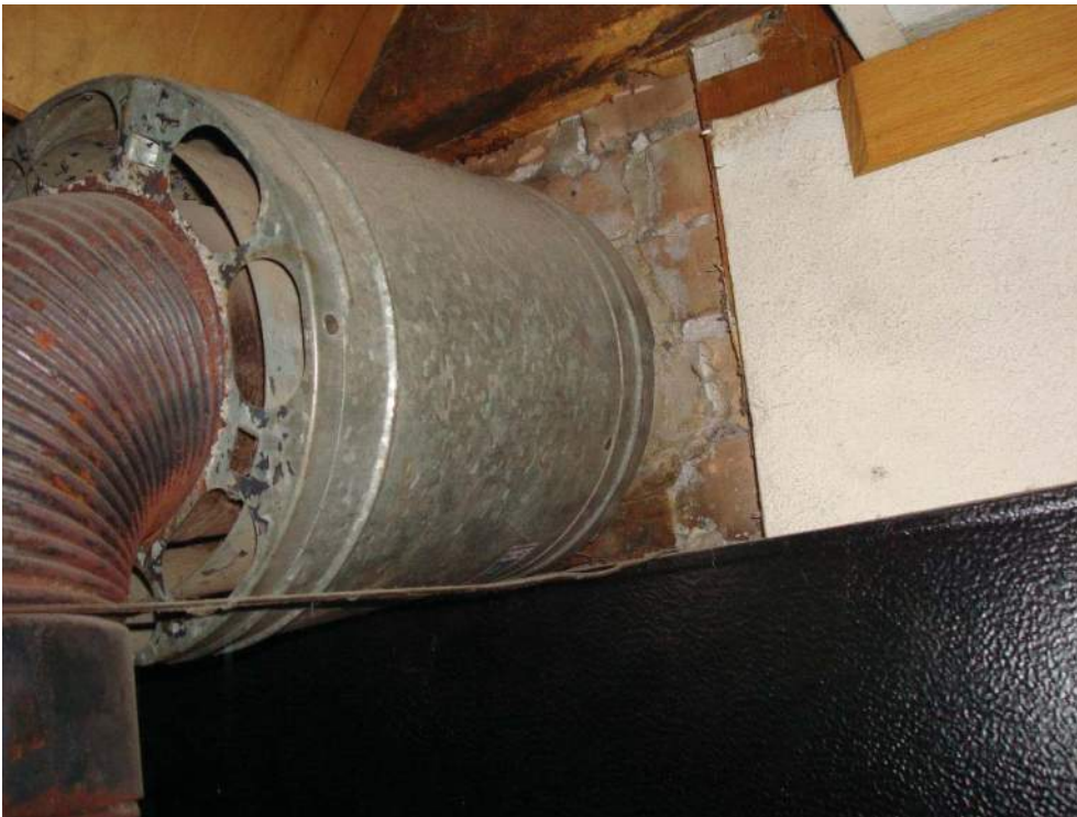
Photo 8j: Stove pipe to masonry chimney
