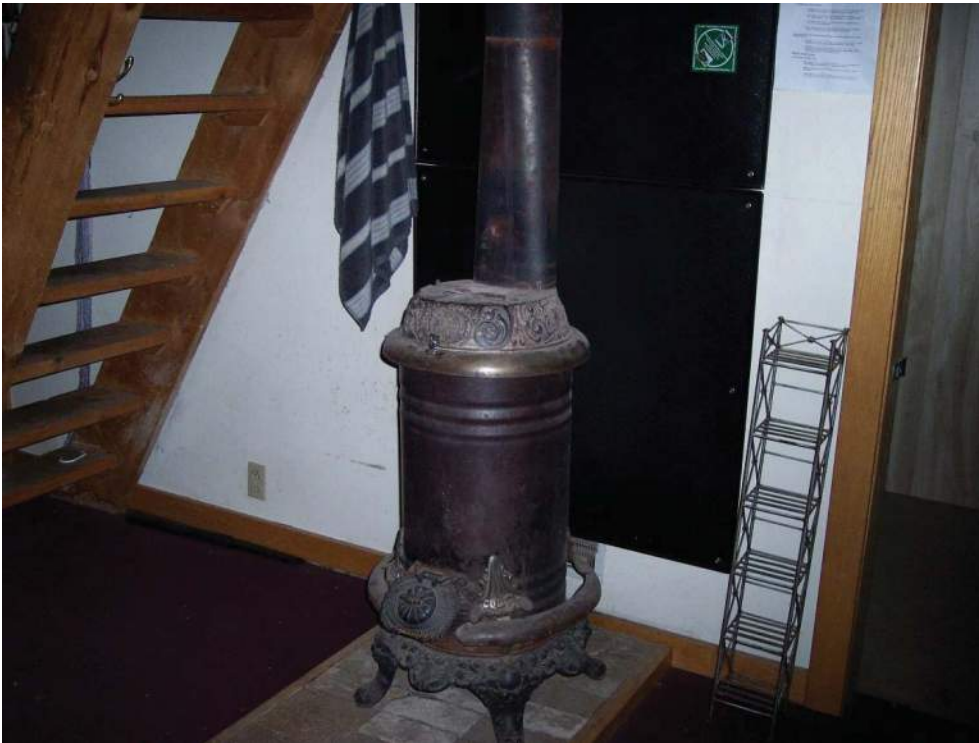
Photo 8j: Stove pipe to masonry chimney
