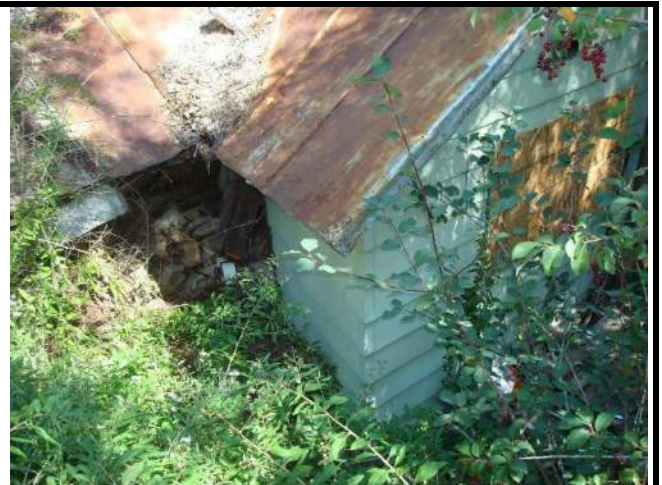
Addition buried in the hillside, west side of the house.
