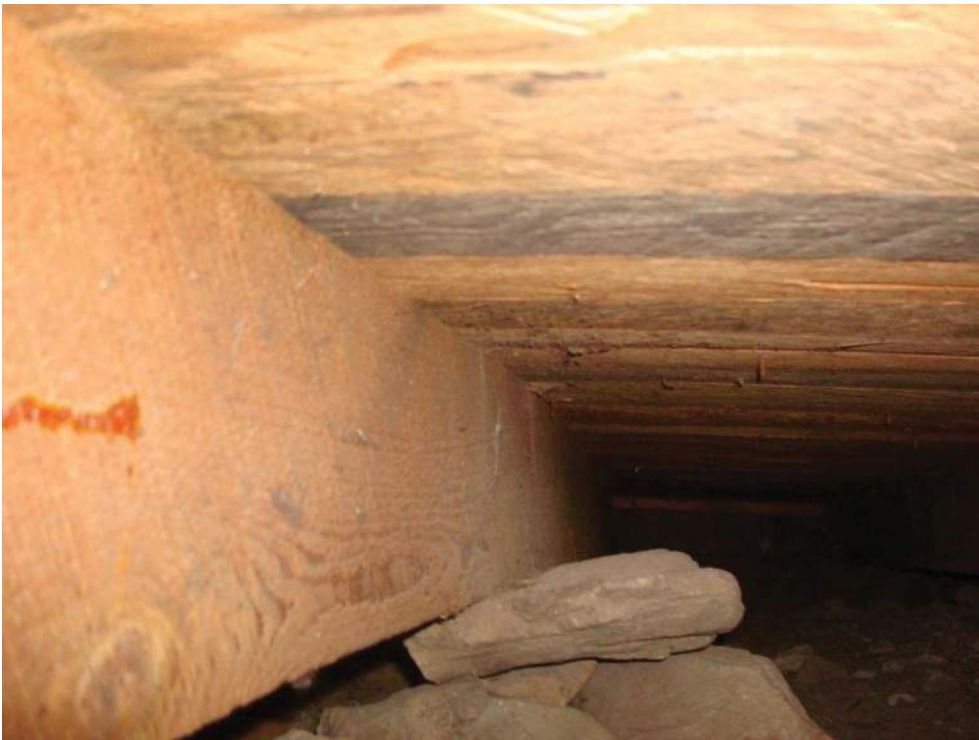
Photo 2c: Typical joist bearing on stone/soil
