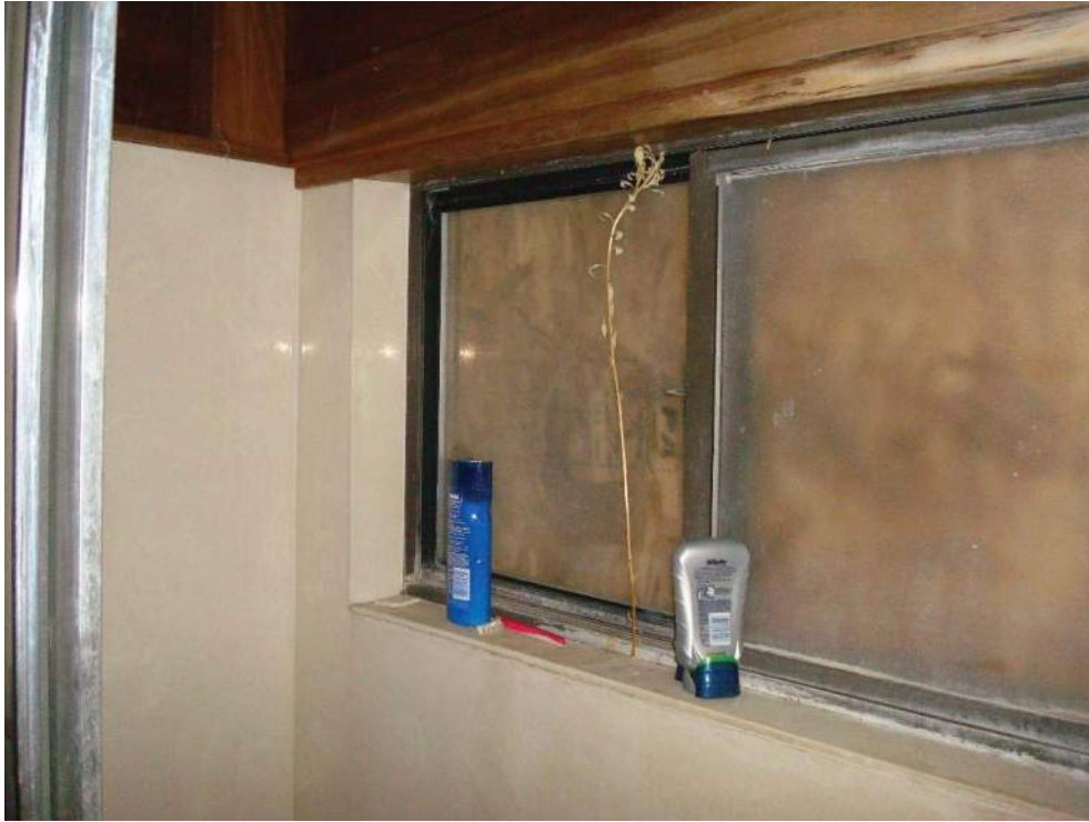
Photo 10g: Bathroom window W8
