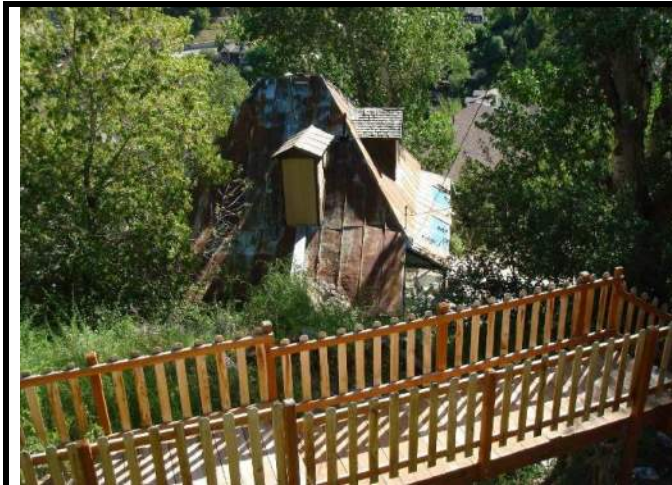
View of the house from the Sampson Avenue right-of-way.
