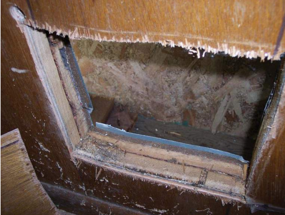
Photo 2c: Typical joist bearing on stone/soil
