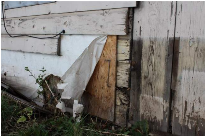
Layers of siding present at the time of the deconstruction in 2013
