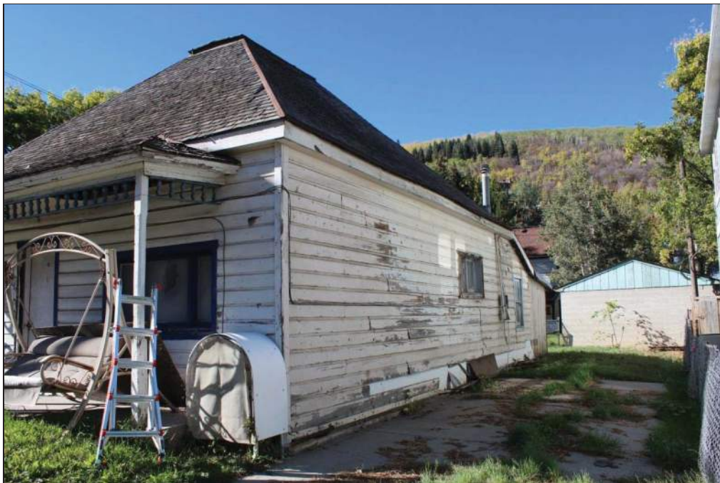
A.2. LANDSCAPING: Concrete parking pad on north side, facing southwest
