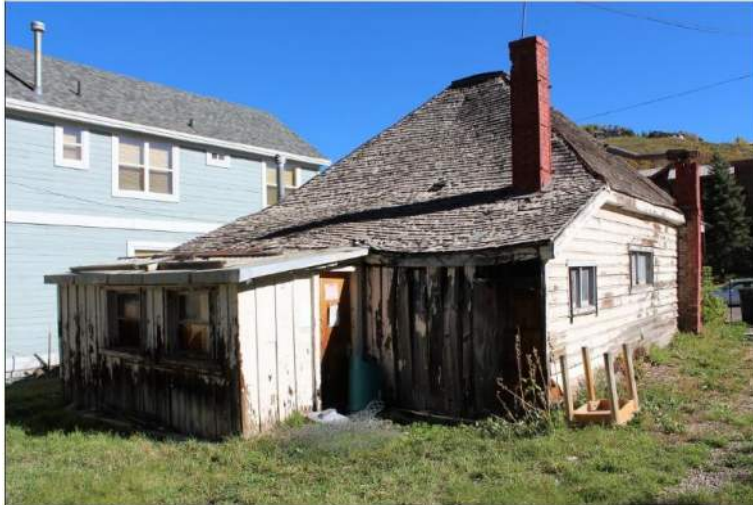
This photograph shows the condition of the two additions in 2014. The additions had begun to pull away from the original pyramid-shaped roof and had significantly deteriorated due to inadequate foundations.
