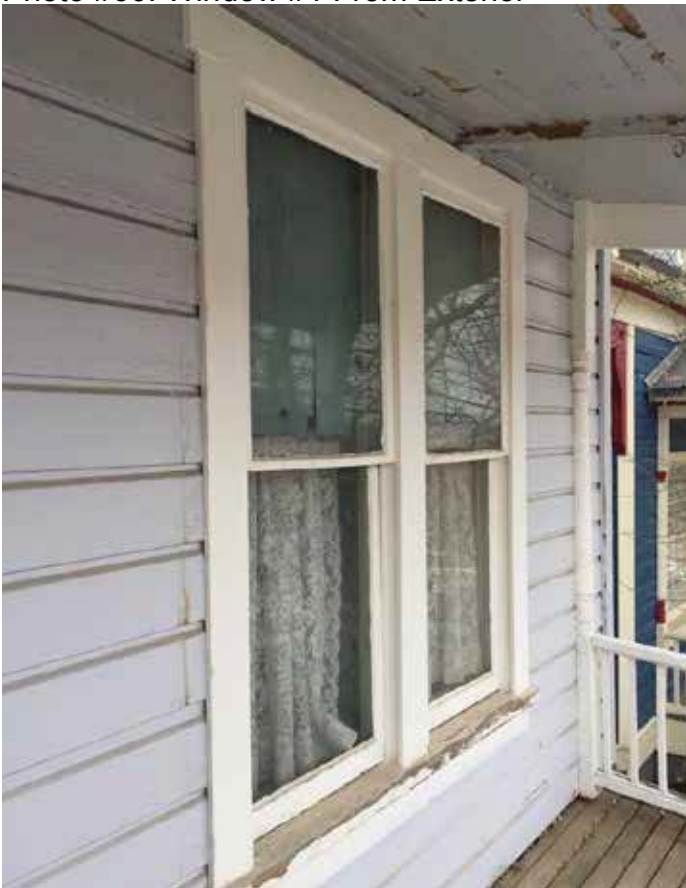
Photo #60: Window #1 From Exterior
