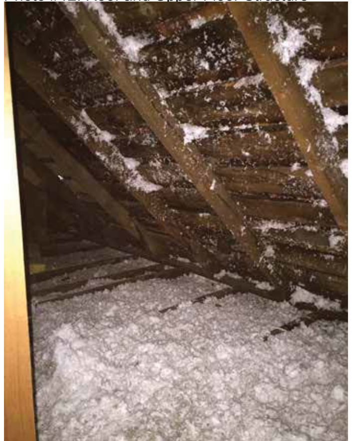
Photo #12: Roof and Upper Floor Structure
