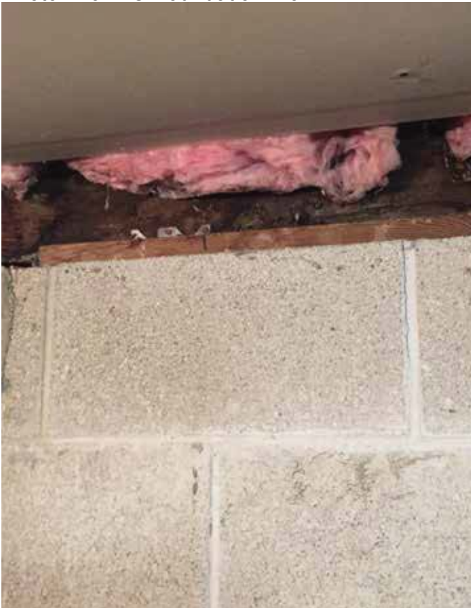
Photo #40: T.O Foundation Wall
