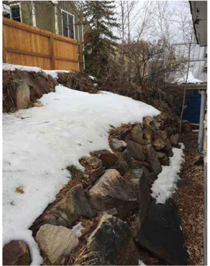
Photo #5: Southeast Corner
