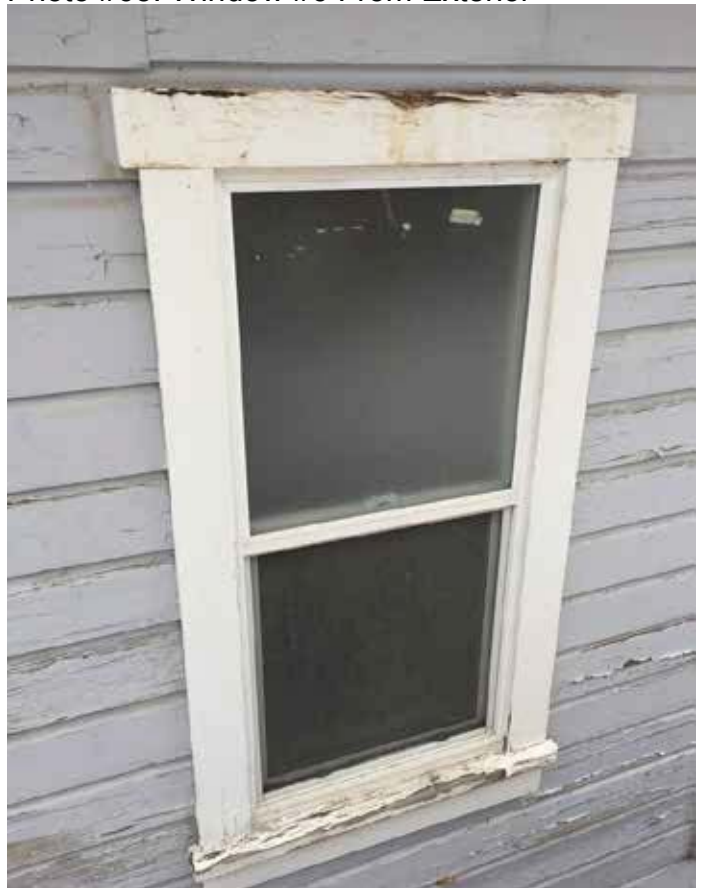
Photo #65: Window #6 From Exterior
