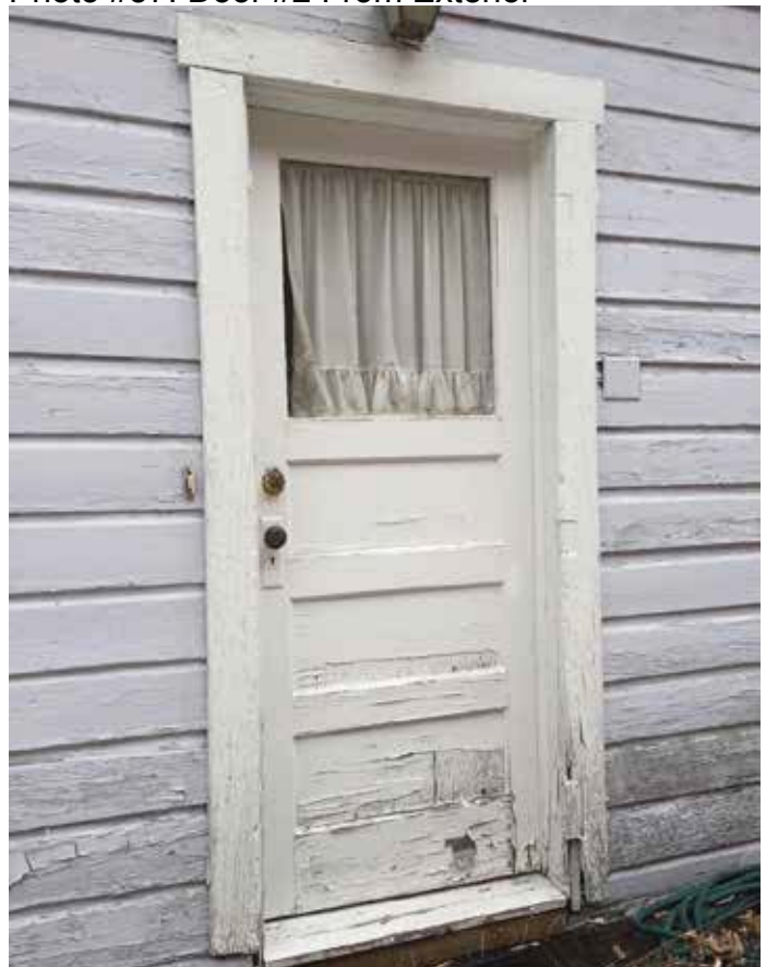
Photo #57: Door #2 From Exterior
