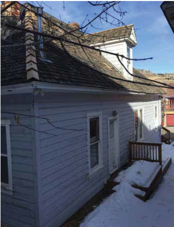
Photo #29: Southwest Facade
