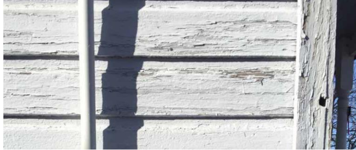
Close-up of siding condition.
