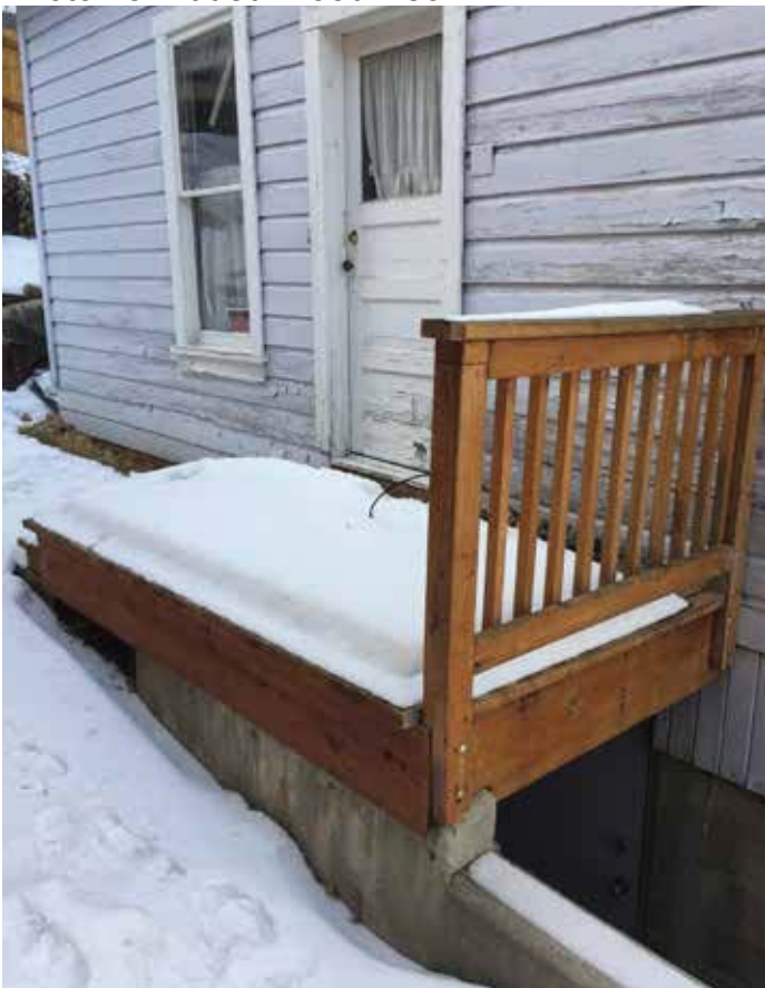
Photo #8: Added Wood Deck
