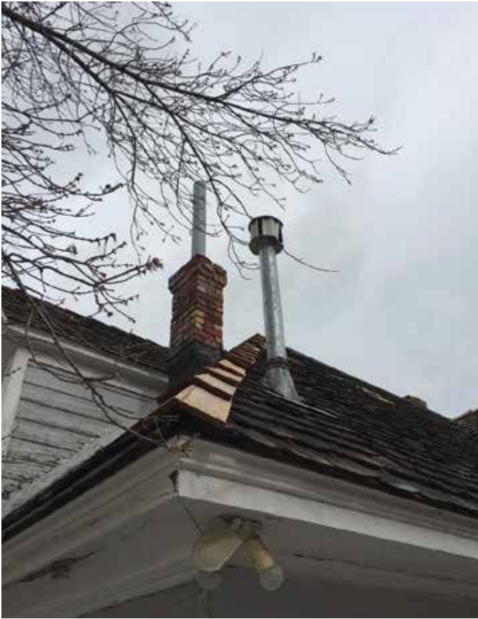
Photo #23: Rear Chimney From Southeast
