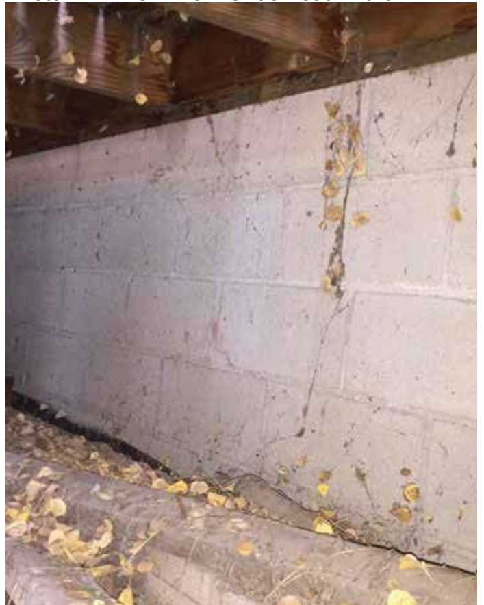
Photo #41: View From Underneath Porch
