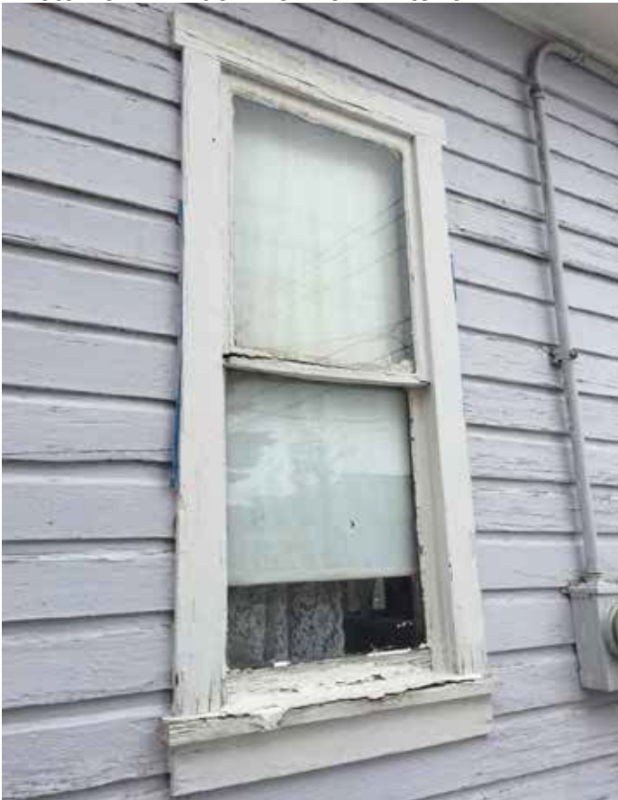
Photo #62: Window #3 From Exterior
