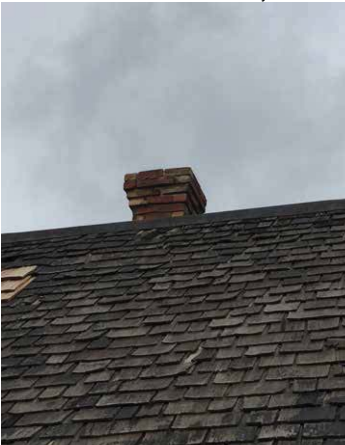
Photo #20: Exterior w/ Front Chimney
