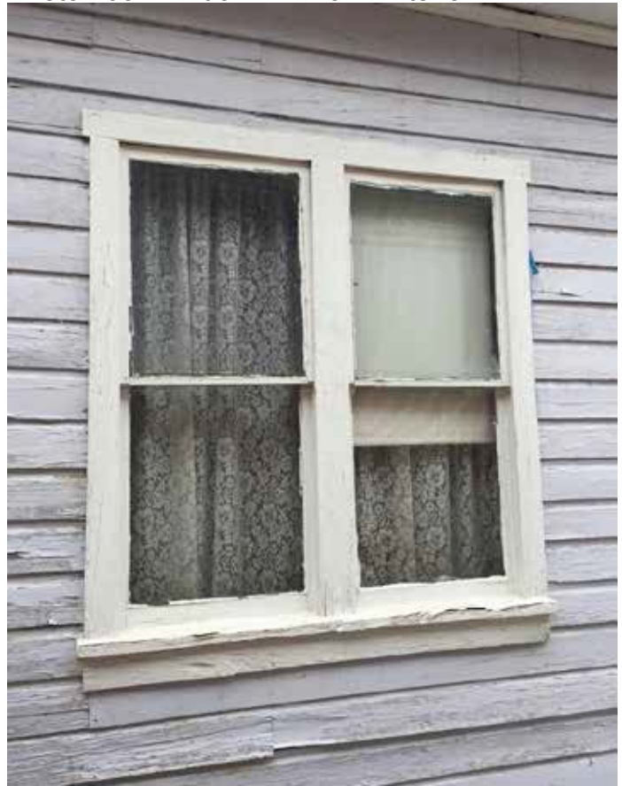
Photo #63: Window #4 From Exterior
