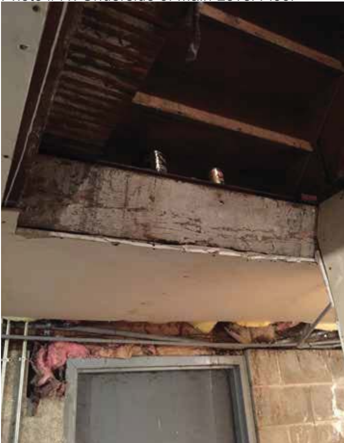
Photo #11: Underside of Main Level Floor
