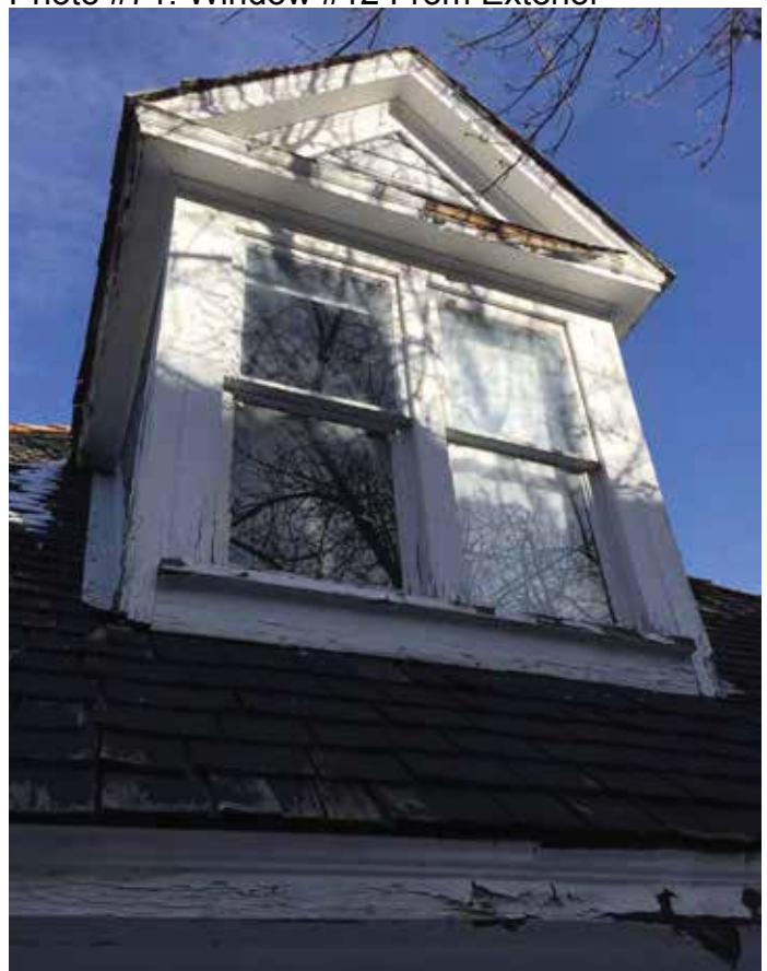
Photo #71: Window #12 From Exterior
