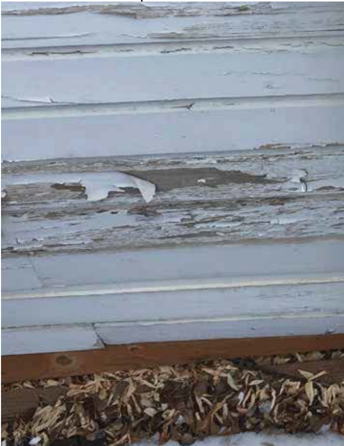
Photo #34: Close Up At Bottom Of Wall
