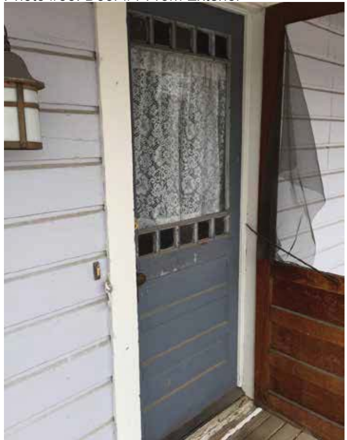
Photo #55: Door #1 From Exterior
