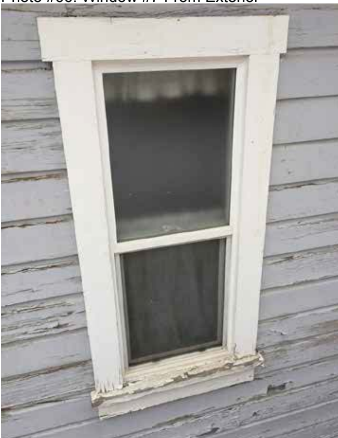
Photo #66: Window #7 From Exterior
