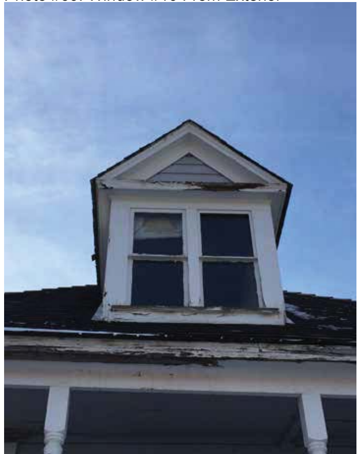
Photo #69: Window #10 From Exterior
