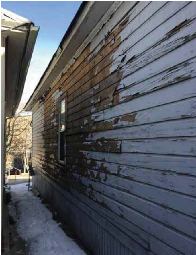
Photo #36: Northwest Facade
