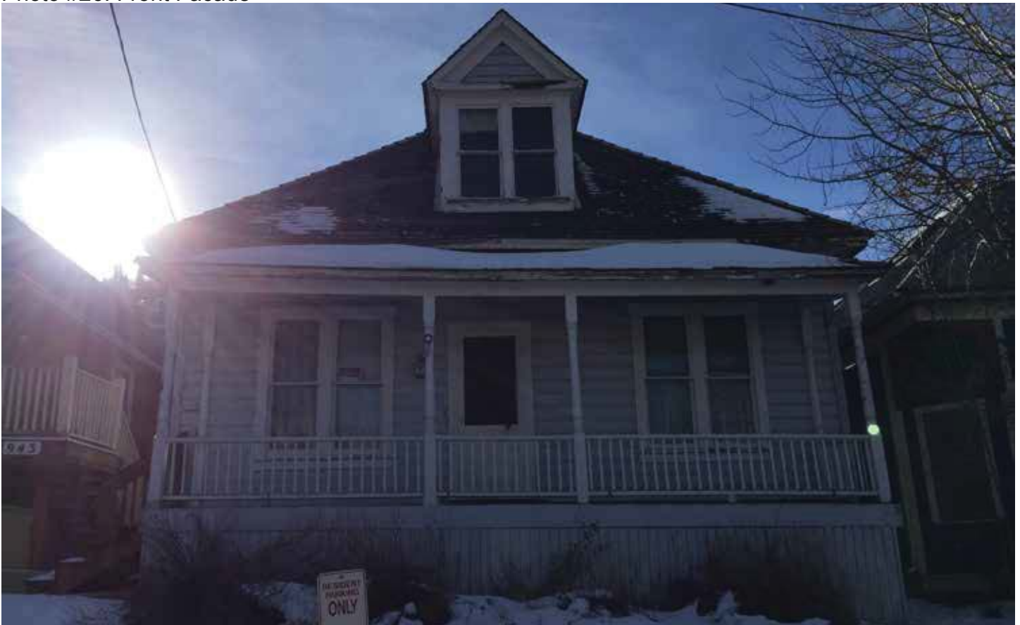
Photo #26: Front Facade
