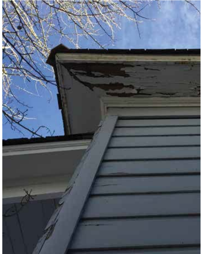
Photo #19: Underside of Soffit Molding
