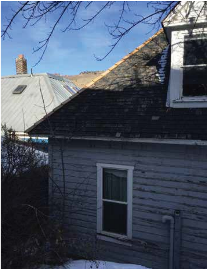
Photo #32: Rear Facade
