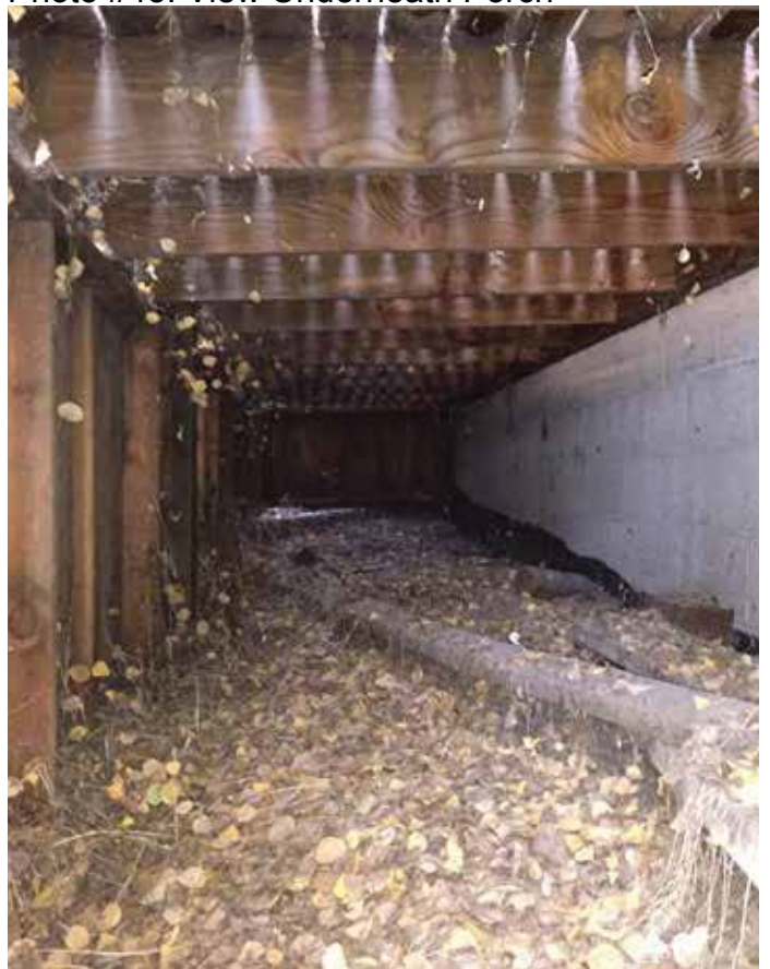
Photo #45: View Underneath Porch
