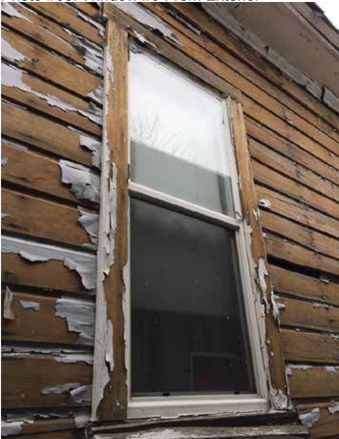
Photo #68: Window #9 From Exterior
