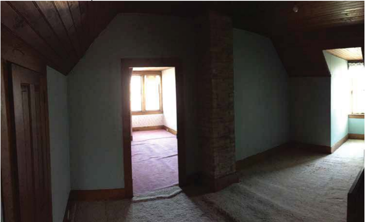
Photo #22: Front Chimney On 2nd Floor
