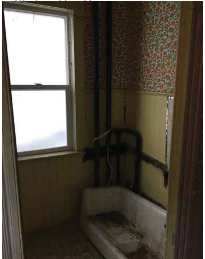
Photo #92: Wash Room - 2
