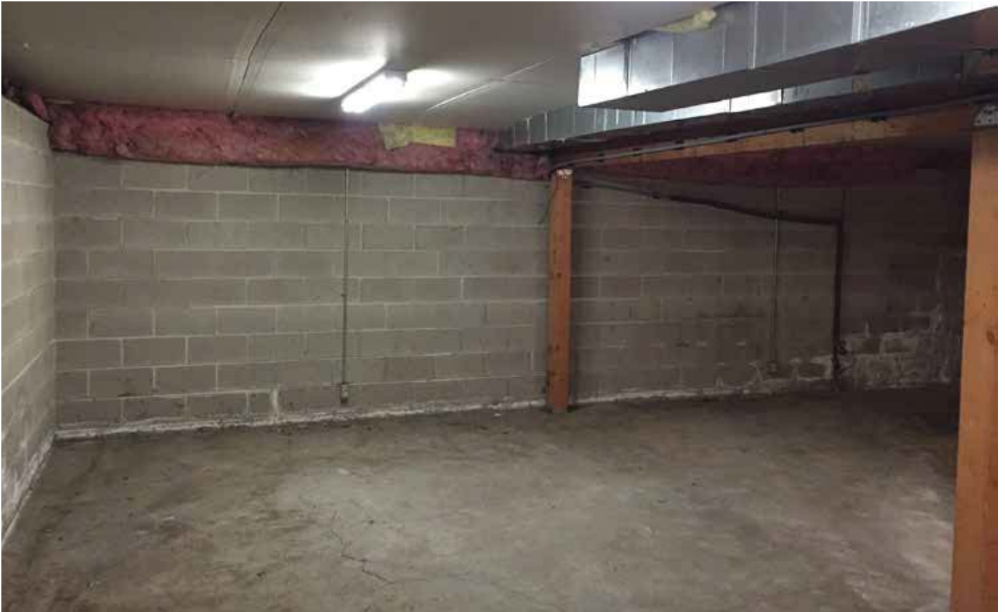
Photo #39: Foundation Wall From Basement
