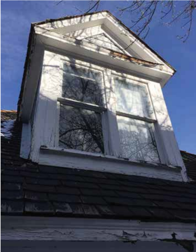
Photo #18: Rear Facade Dormer
