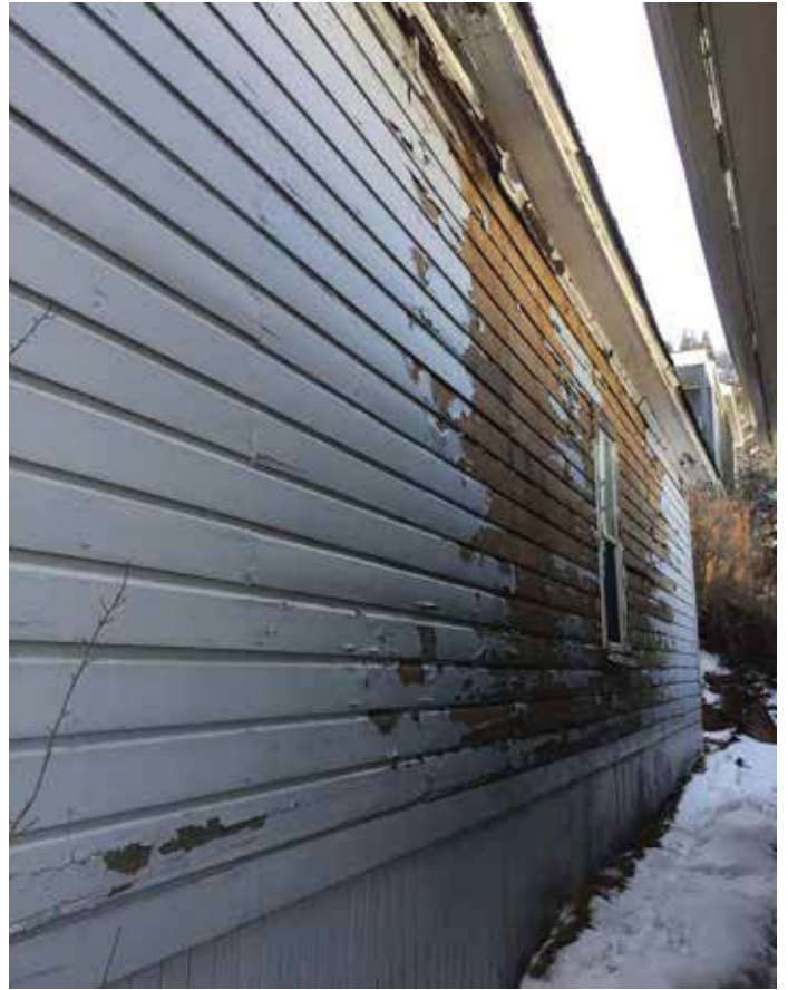
Photo #37: Northwest Facade
