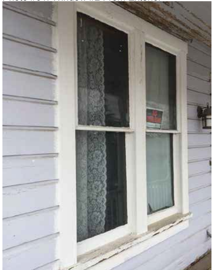
Photo #61: Window #2 From Exterior
