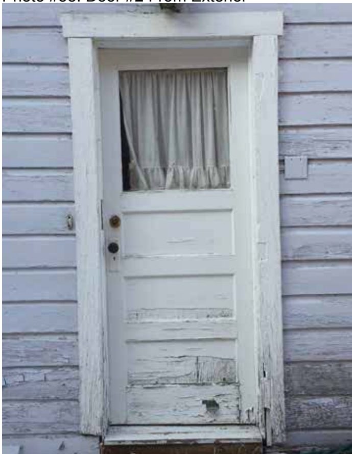
Photo #58: Door #2 From Exterior
