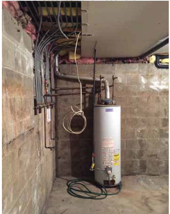
Photo #75: South Corner Of Basement
