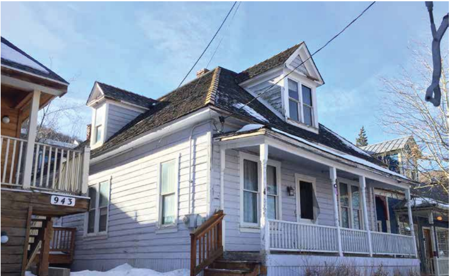
Photo #13: Roof From Northeast Corner
