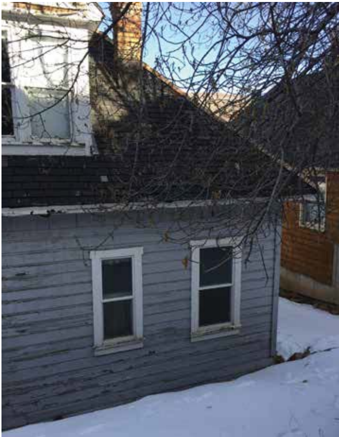
Photo #33: Rear Facade
