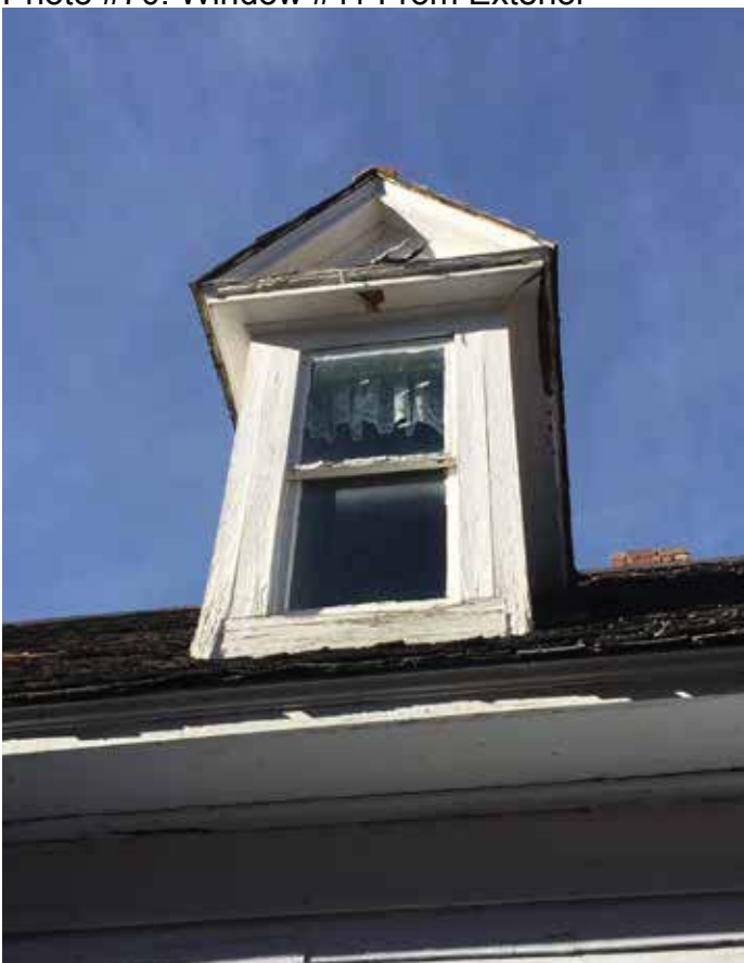
Photo #70: Window #11 From Exterior
