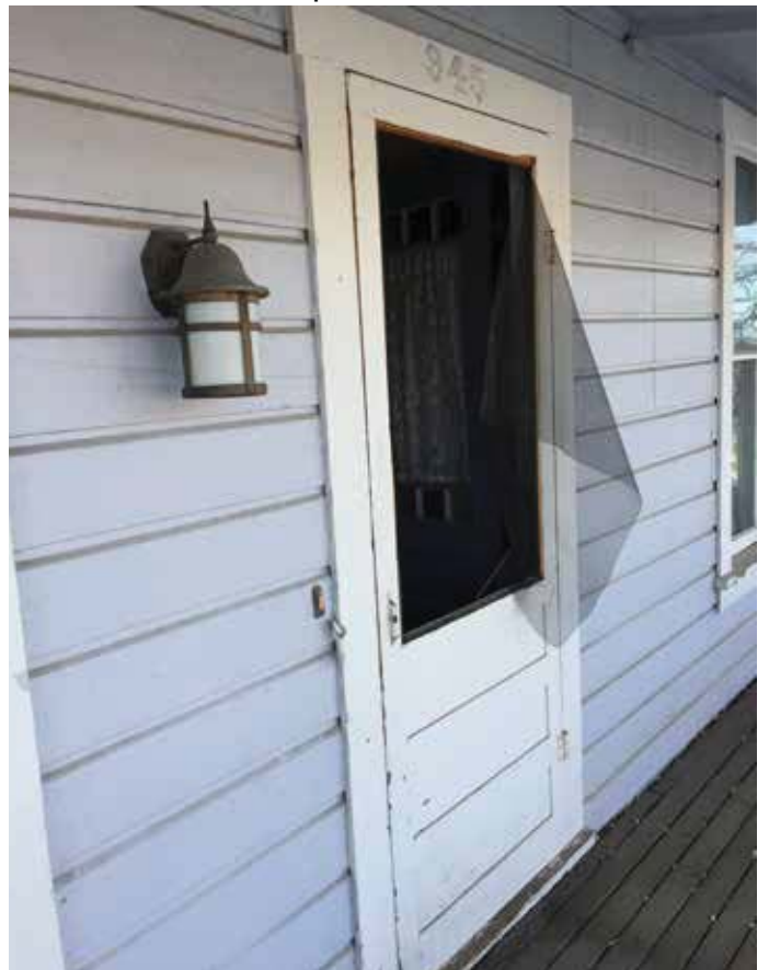
Photo #28: Close Up At Door
