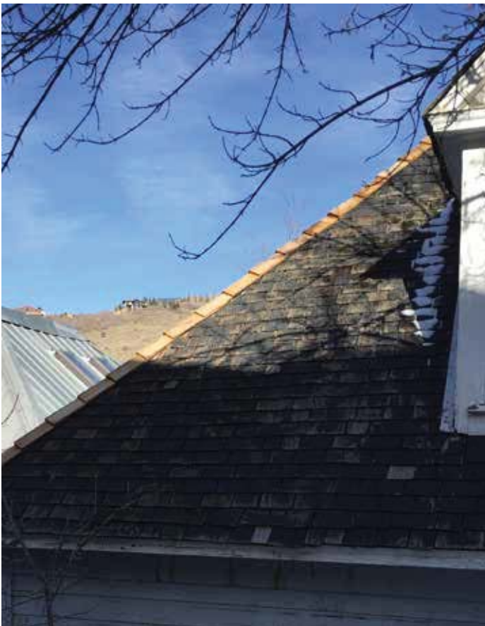
Photo #14: Roof From Rear
