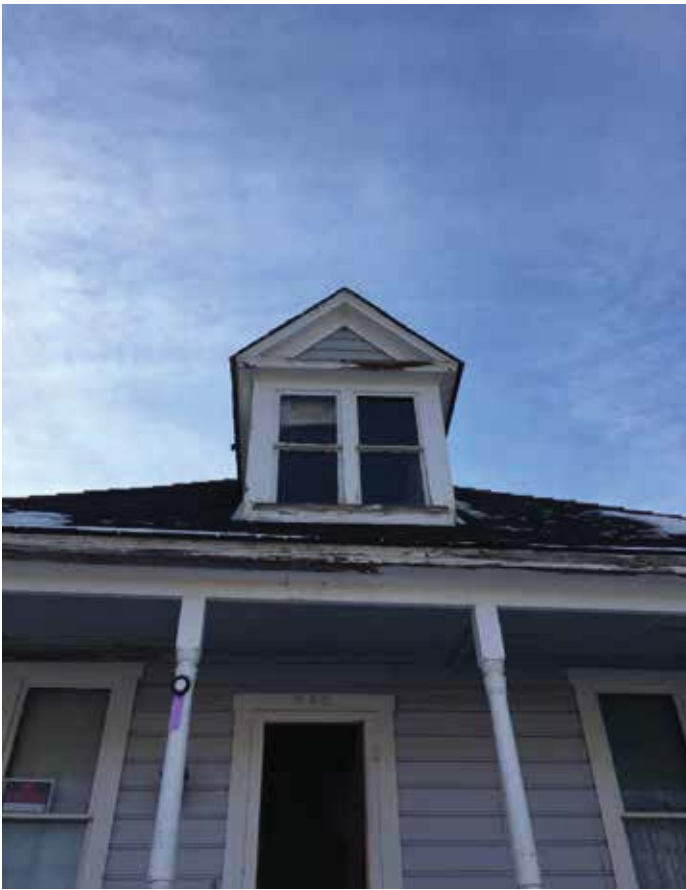
Photo #16: Front Facade Dormer
