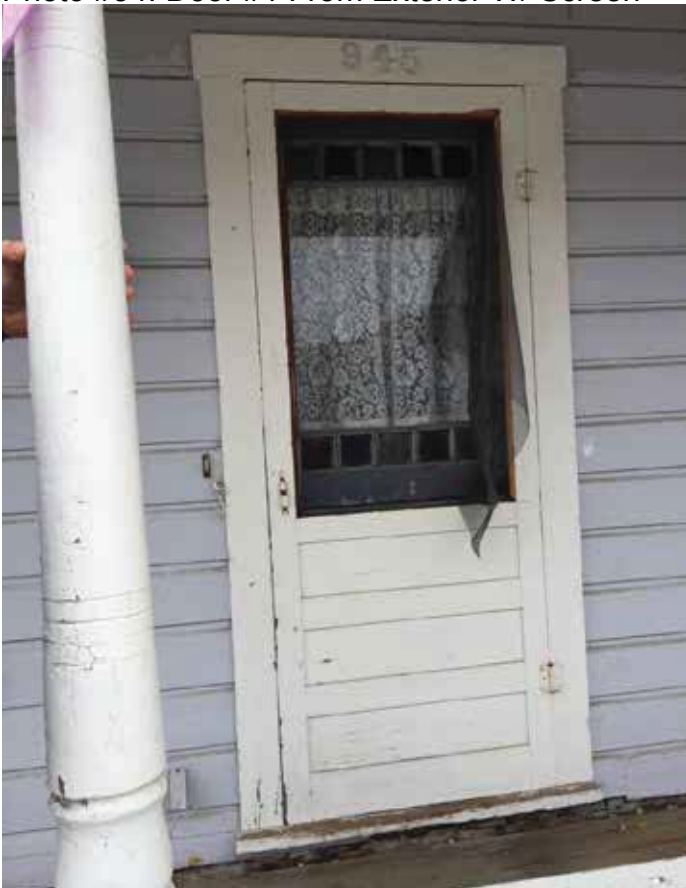
Photo #54: Door #1 From Exterior W/ Screen
