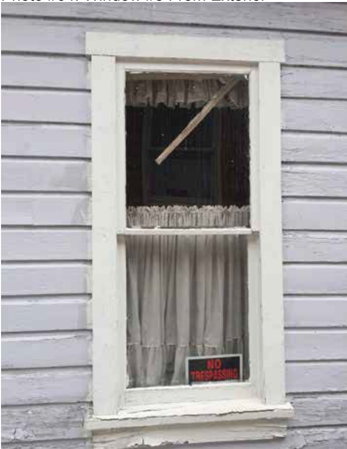
Photo #64: Window #5 From Exterior
