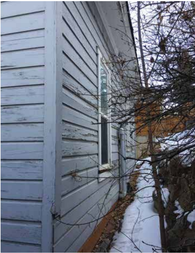
Photo #4: Southwest Corner
