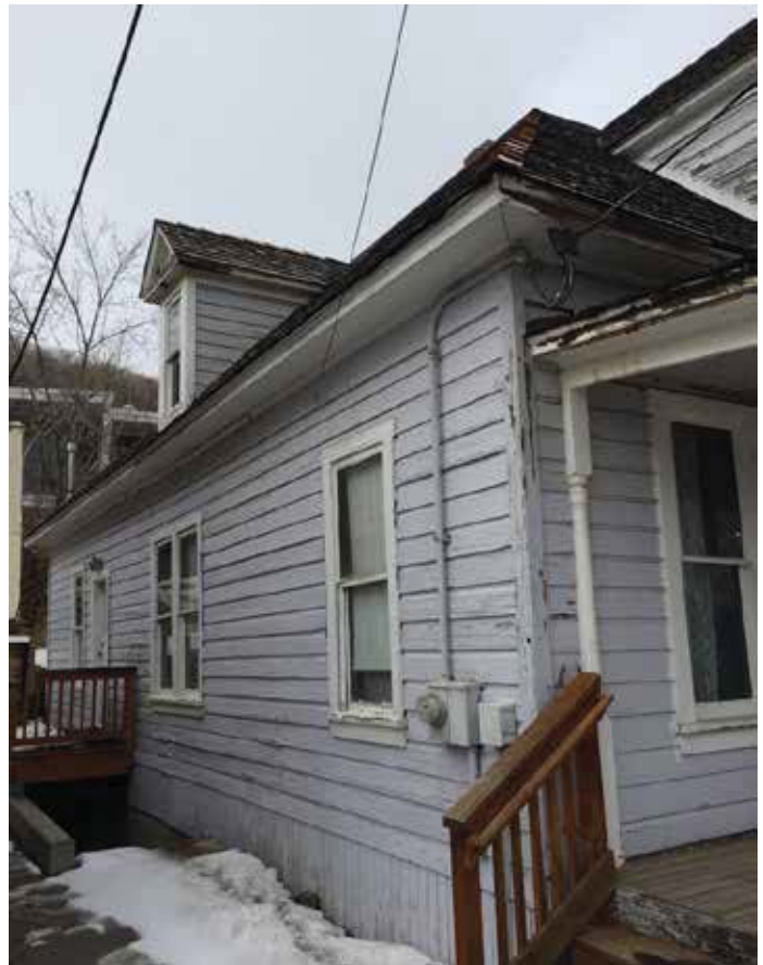
Photo #30: Southwest Facade
