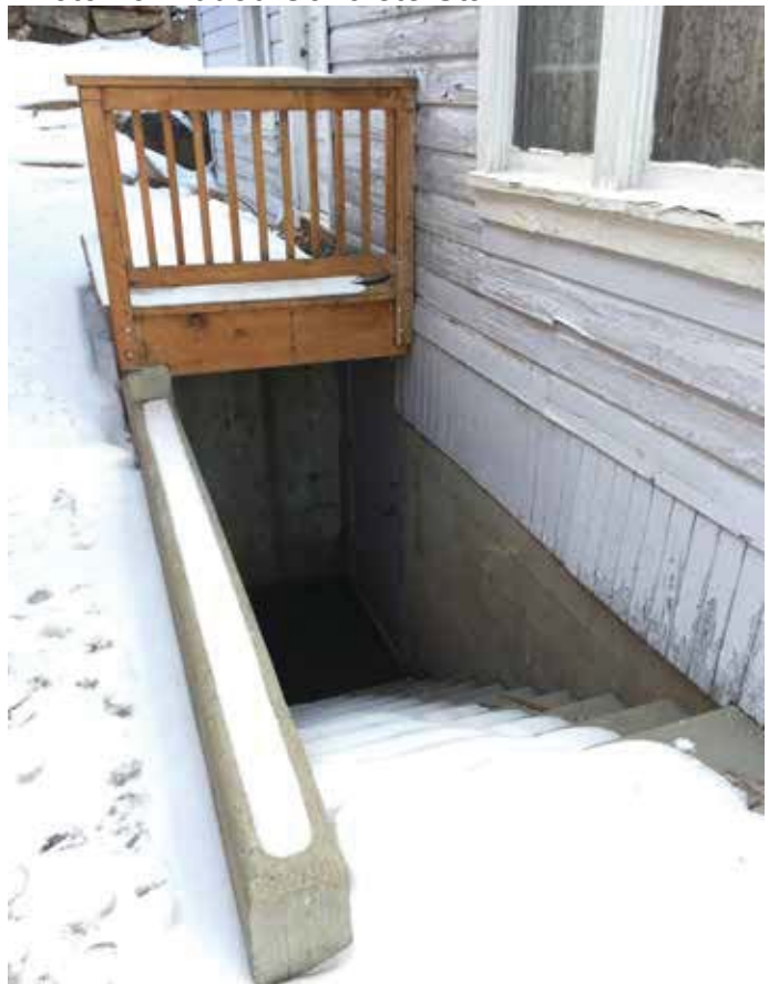
Photo #9: Added Concrete Stair
