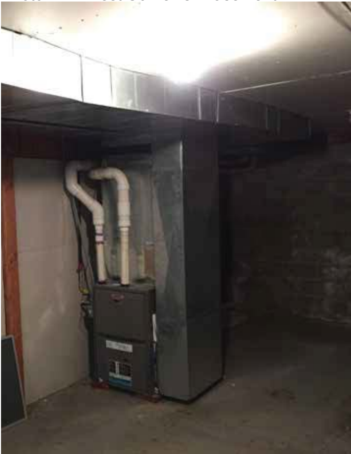
Photo #74: West Corner Of Basement
