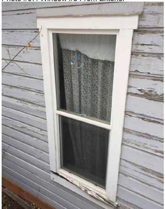
Photo #67: Window #8 From Exterior
