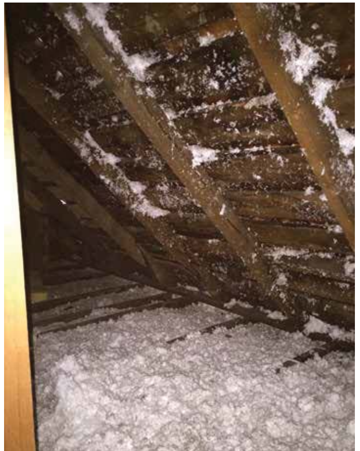
Photo #15: Attic Space Roof Construction
