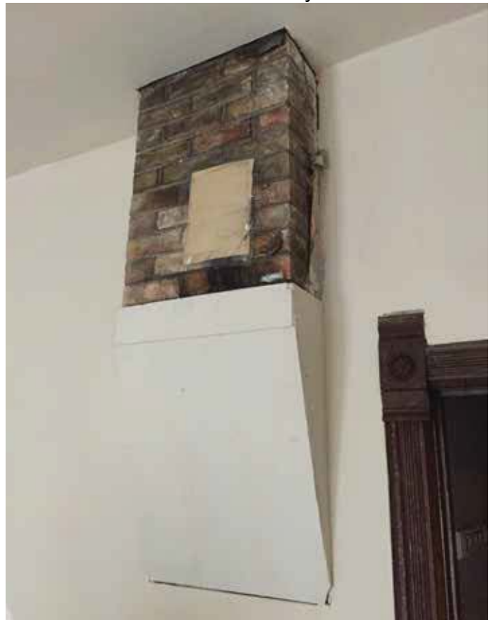
Photo #21: Bottom Of Chimney At Interior
