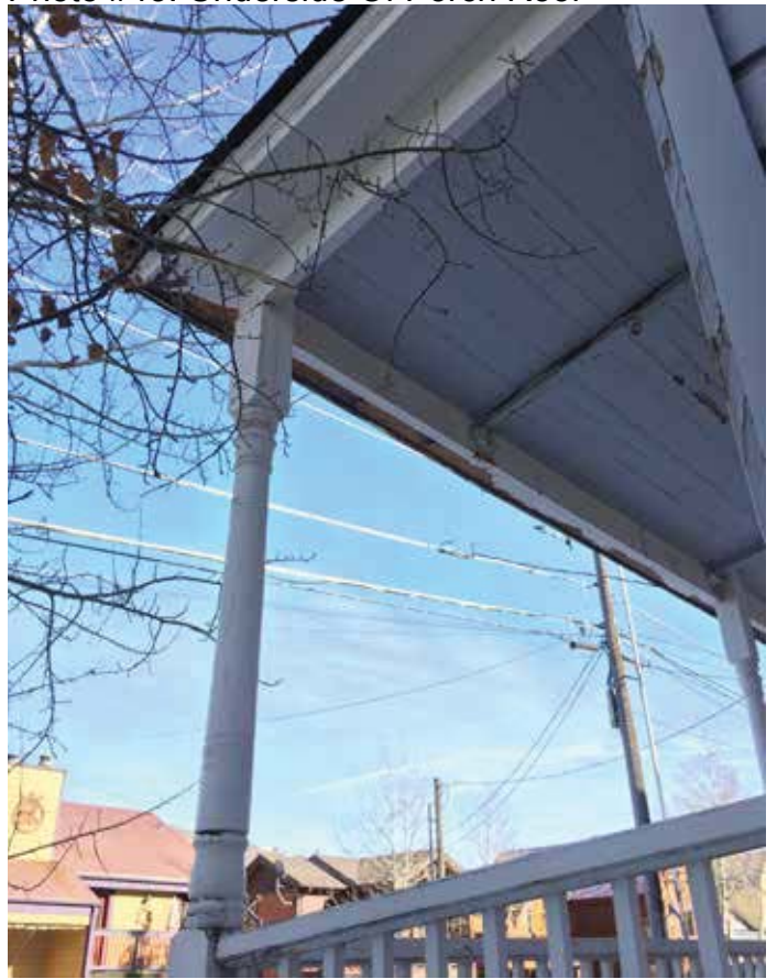
Photo #43: Underside Of Porch Roof
