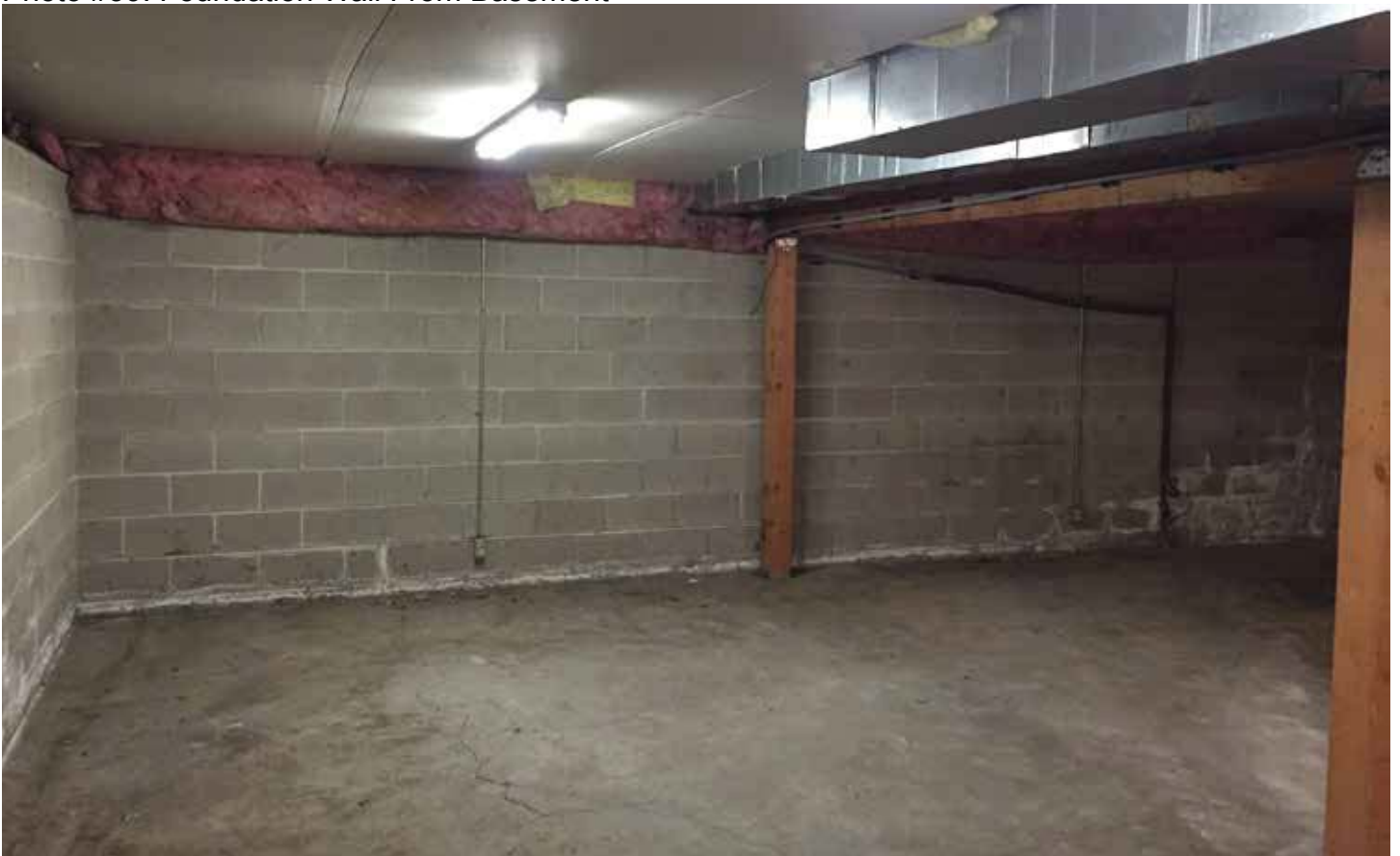
Photo #39: Foundation Wall From Basement
