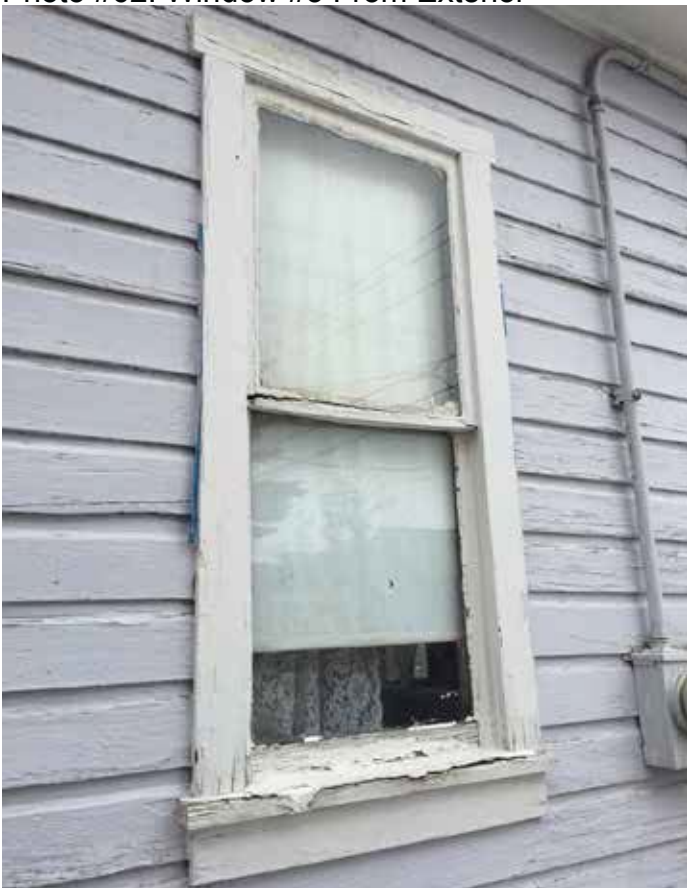
Photo #62: Window #3 From Exterior
