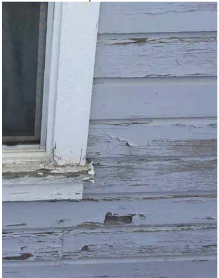
Photo #35: Close Up Near Window
