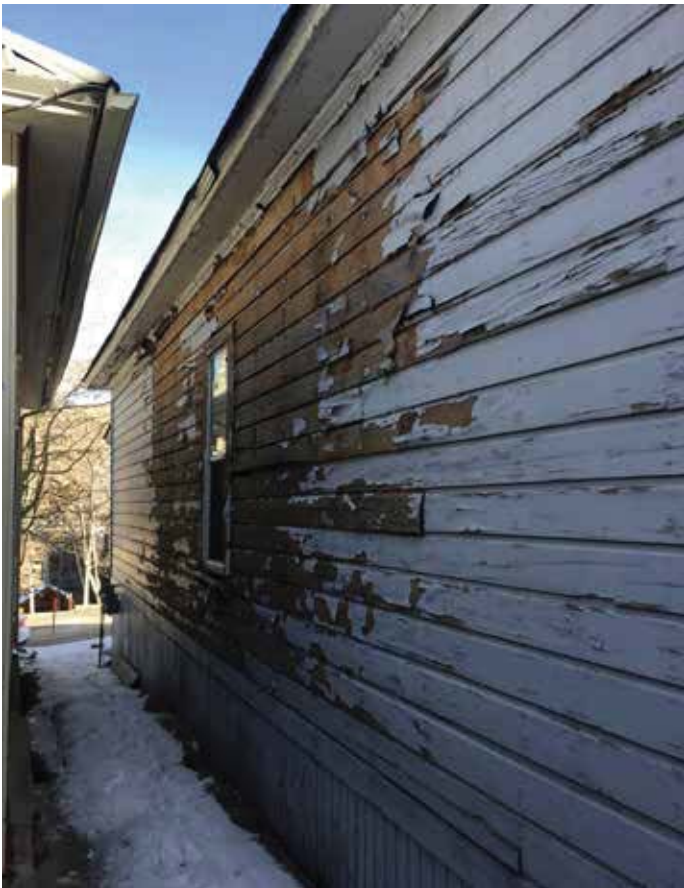
Photo #36: Northwest Facade
