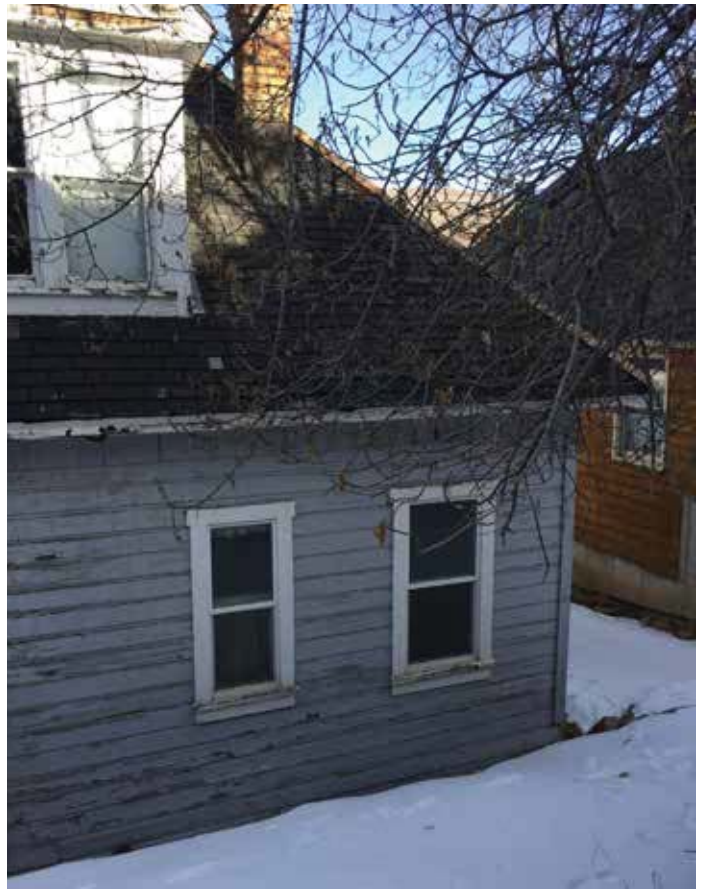
Photo #33: Rear Facade
