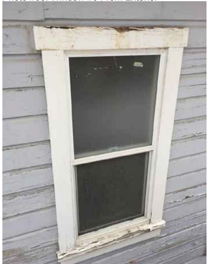
Photo #65: Window #6 From Exterior
