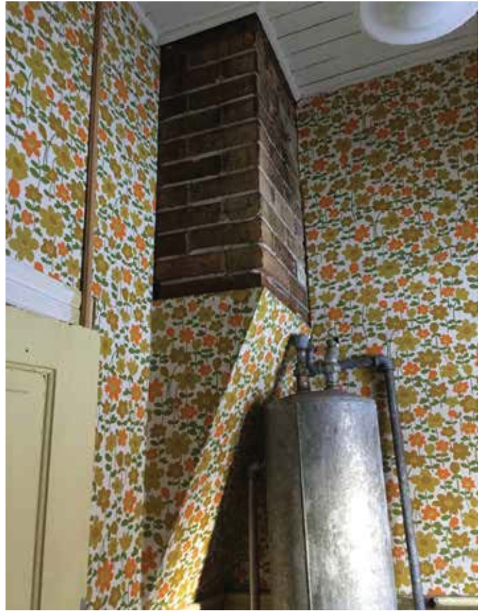
Photo #24: Chimney Within Bathroom
