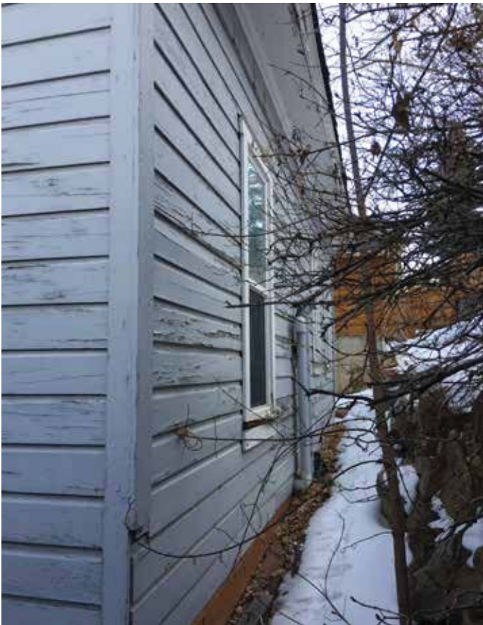
Photo #4: Southwest Corner
