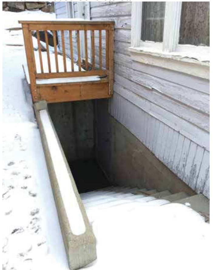
Photo #9: Added Concrete Stair
