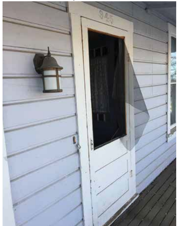
Photo #28: Close Up At Door
