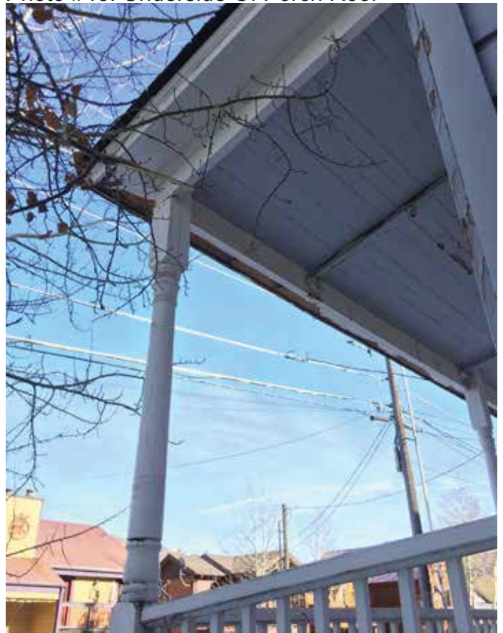
Photo #43: Underside Of Porch Roof
