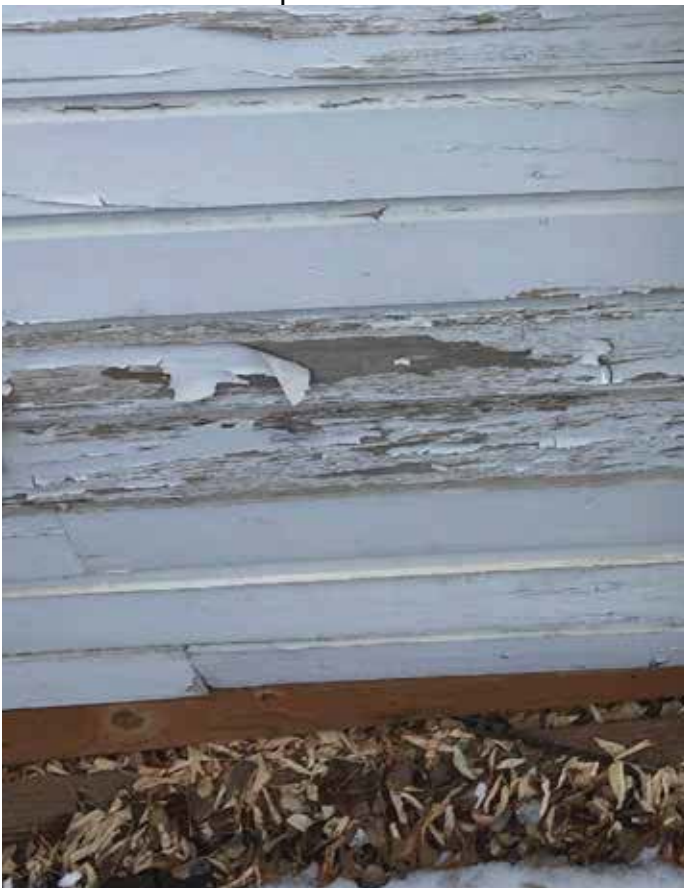
Photo #34: Close Up At Bottom Of Wall
