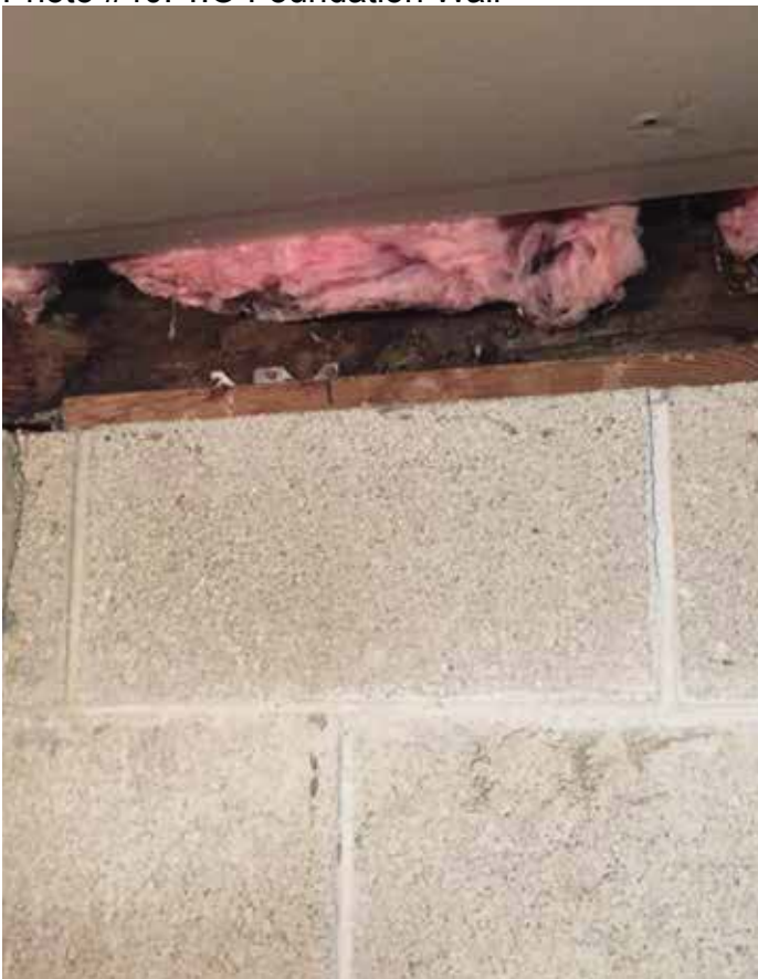
Photo #40: T.O Foundation Wall
