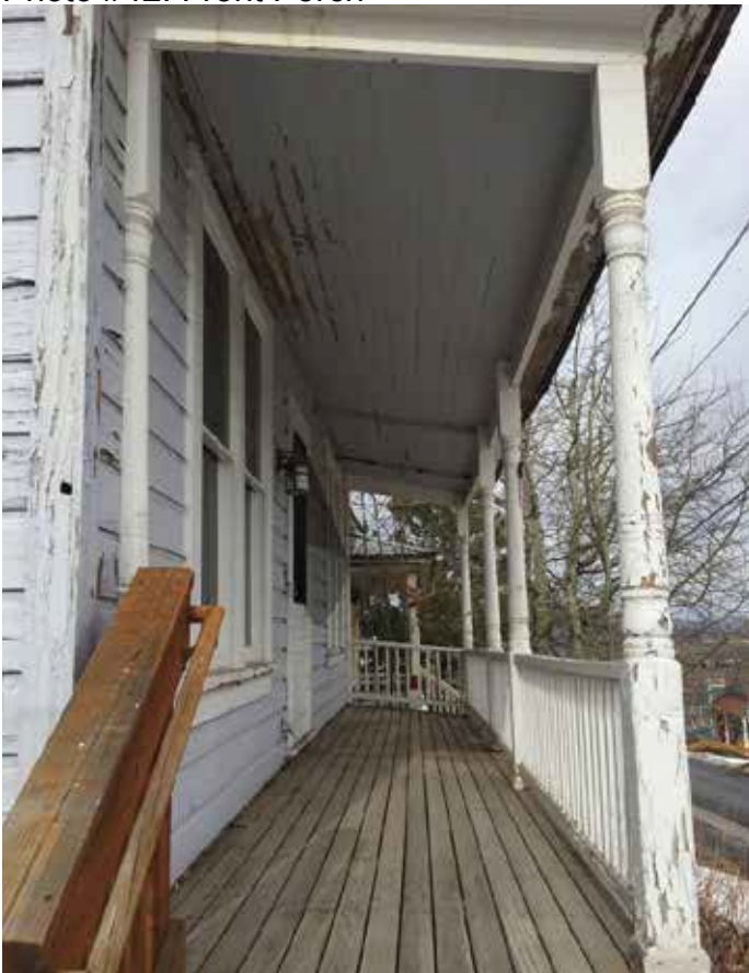
Photo #42: Front Porch
