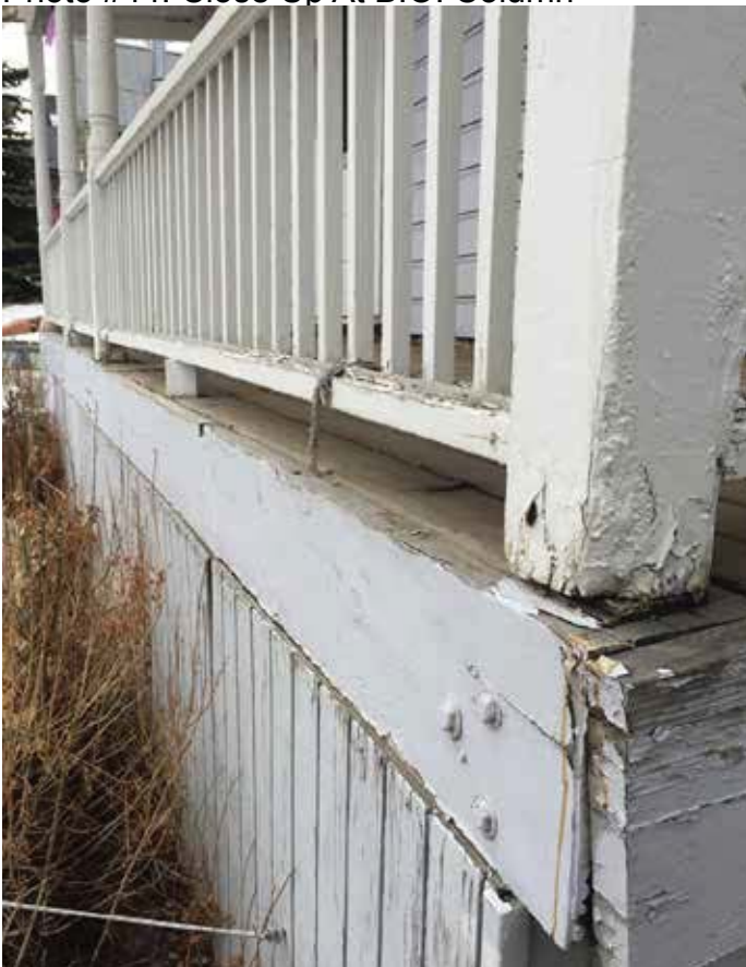
Photo #44: Close Up At B.O. Column
