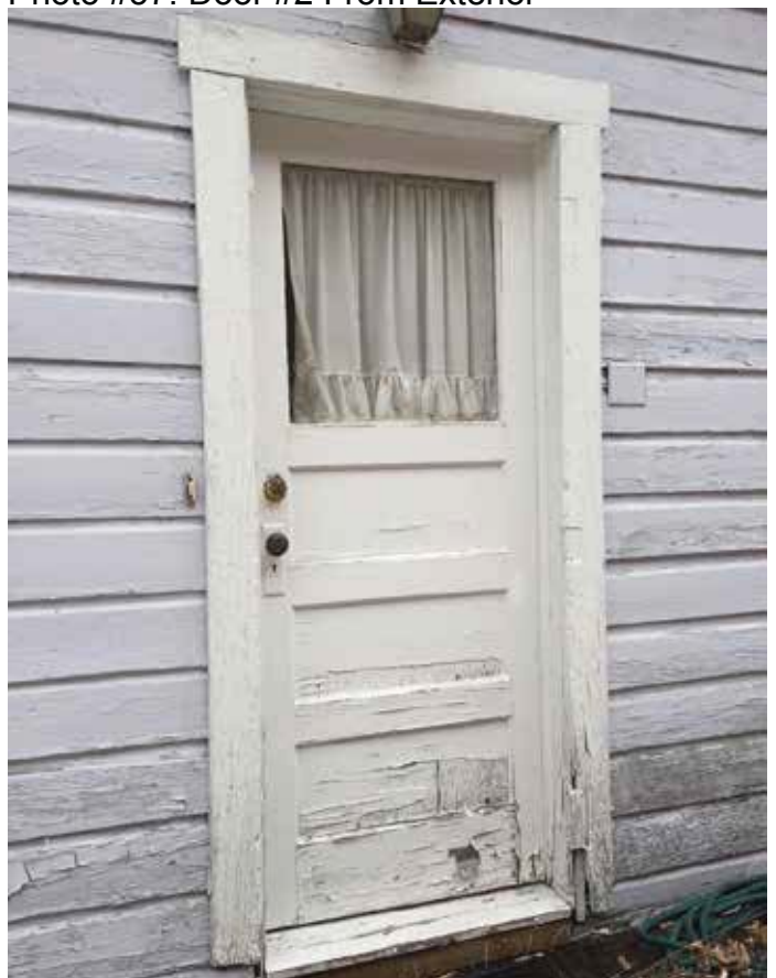
Photo #57: Door #2 From Exterior
