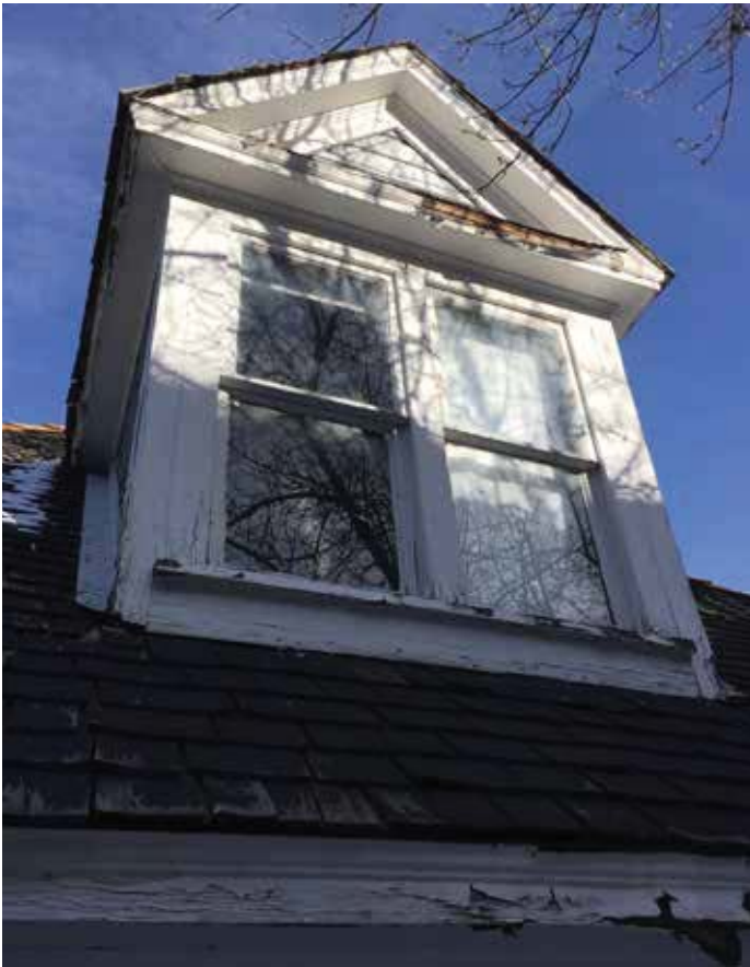
Photo #18: Rear Facade Dormer
