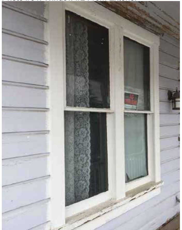
Photo #61: Window #2 From Exterior
