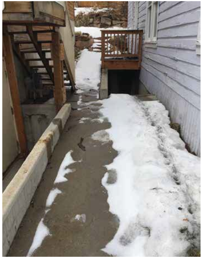
Photo #7: Southeast Side Yard
