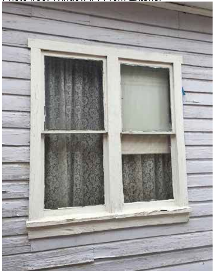
Photo #63: Window #4 From Exterior
