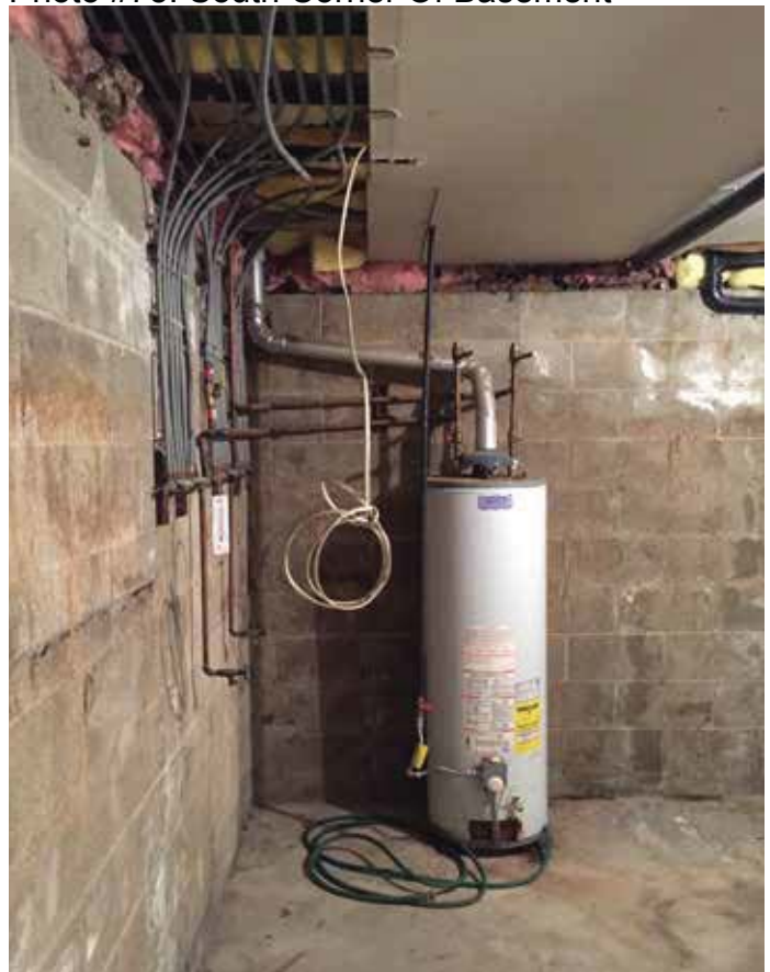
Photo #75: South Corner Of Basement
