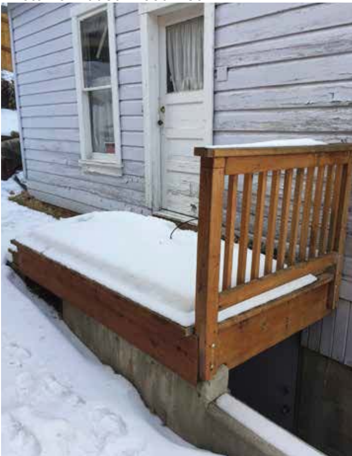
Photo #8: Added Wood Deck
