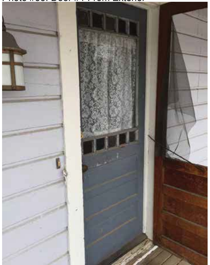
Photo #55: Door #1 From Exterior
