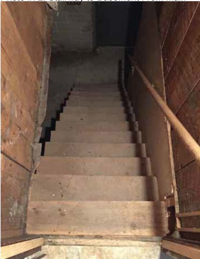
Photo #72: Stairway to Basement From Main
