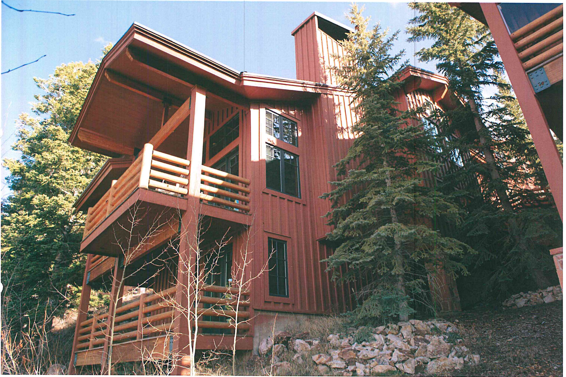
Stag Lodge Phase II Unit 49 - looking easterly
