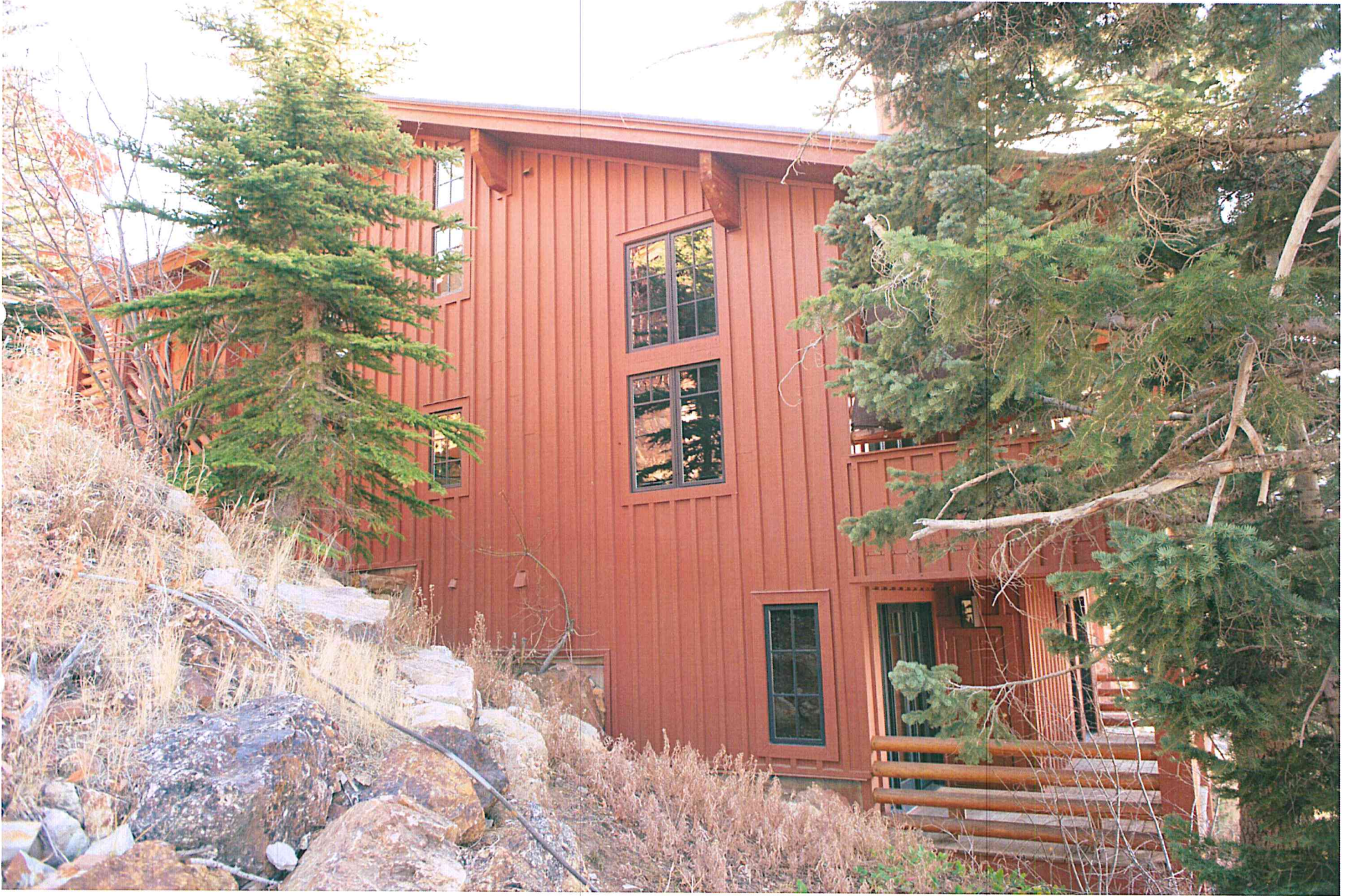
Stag Lodge Phase II Unit 49 - looking southerly
