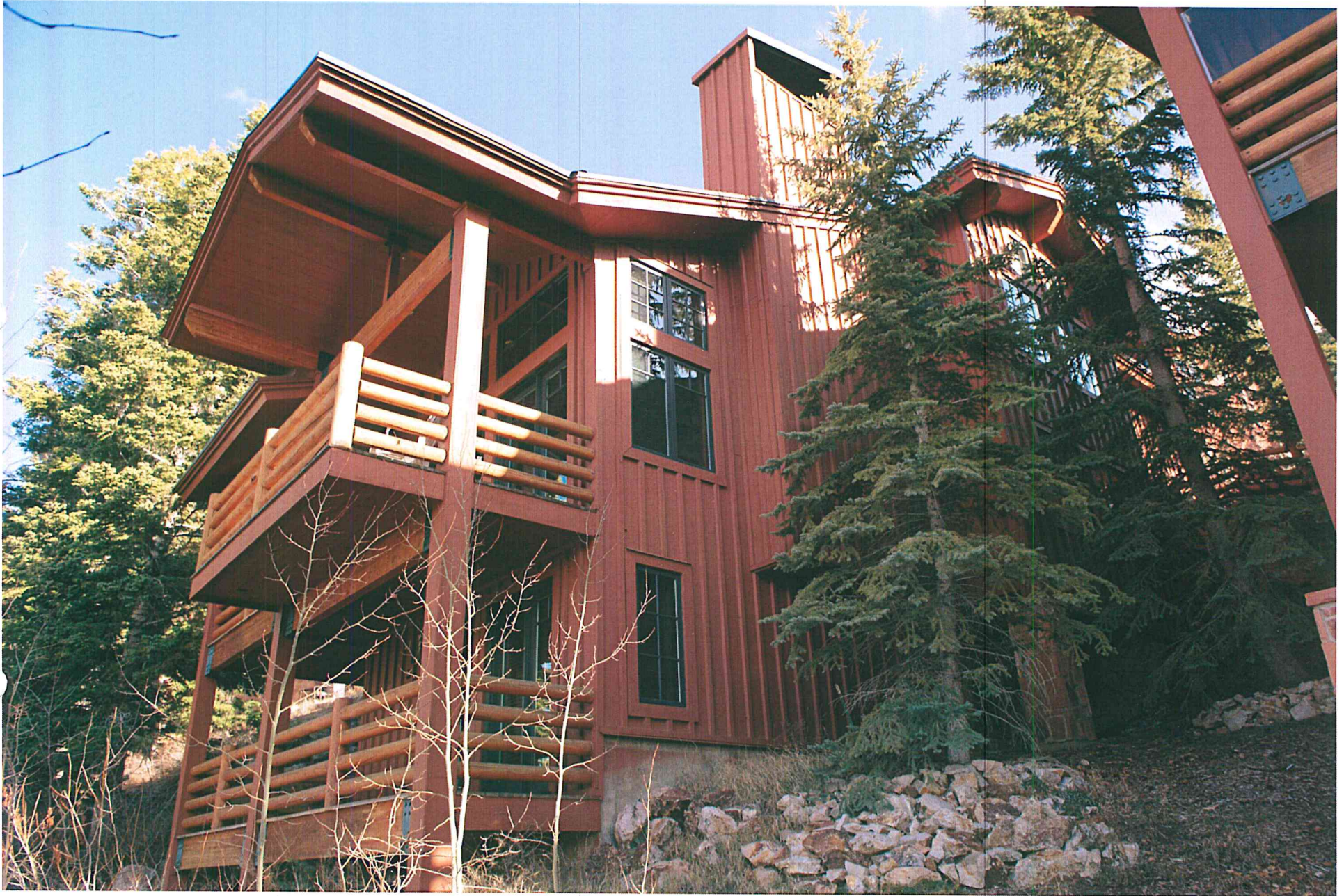
Stag Lodge Phase II Unit 49 - looking easterly
