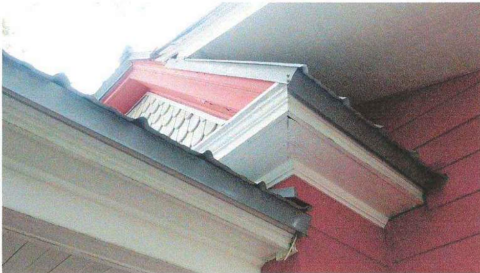
Photo 8: Soffit and Fascia
