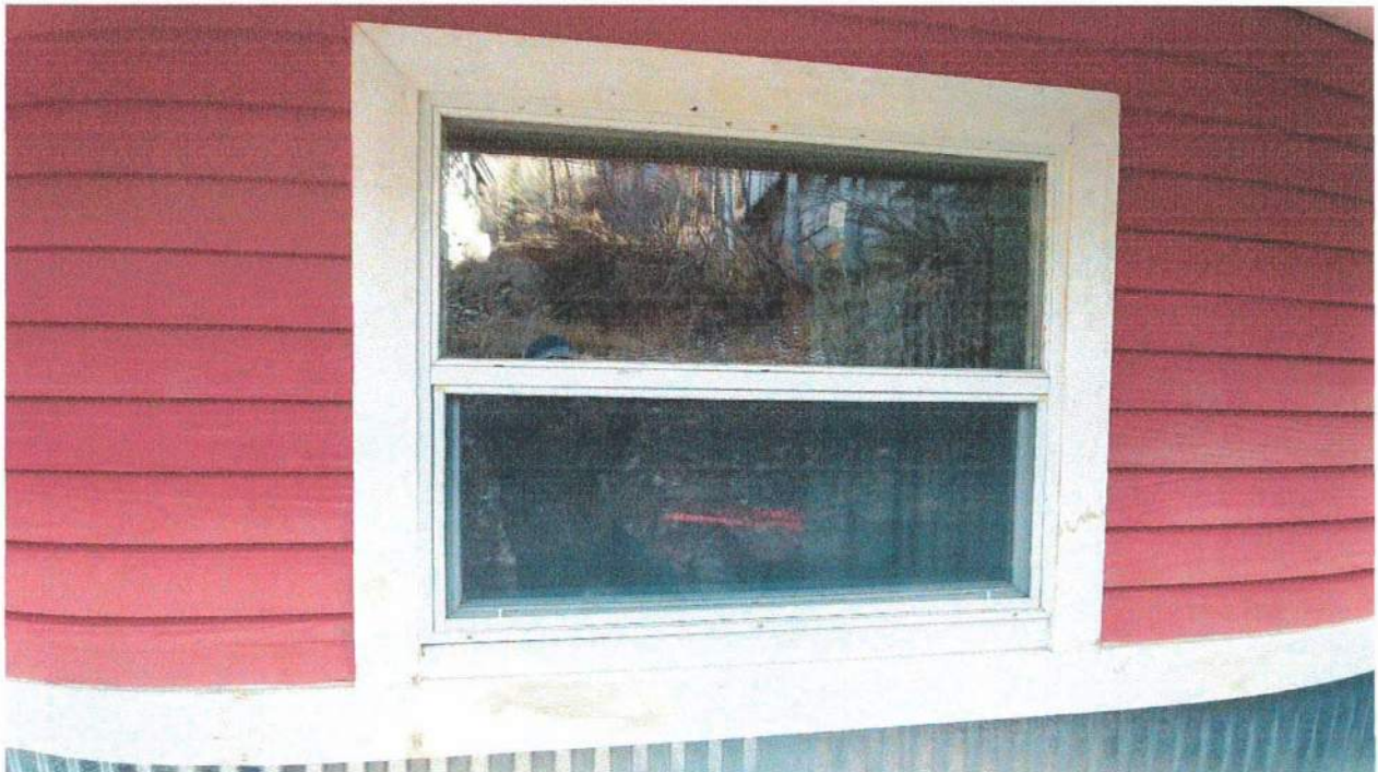
Photo 24: Rear (Window E-206) Non-Historic Addition
