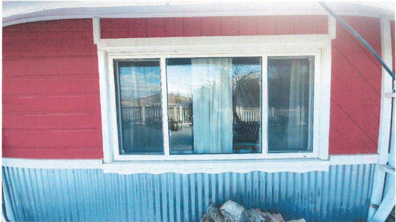
Photo 20: Front Porch Right Window (Window E-210) Non-Historic Addition
