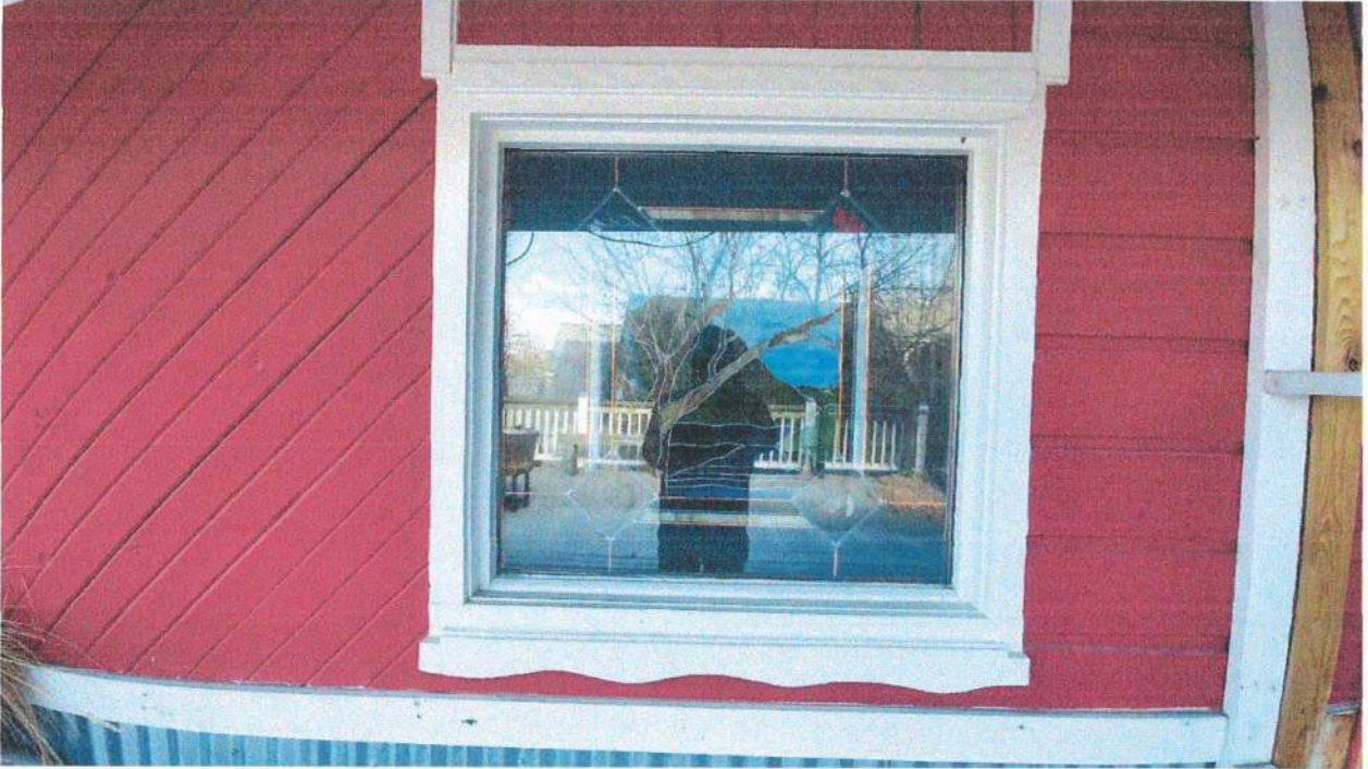
Photo 21: Deck Right Side (Window E-211) Non-Historic Addition
