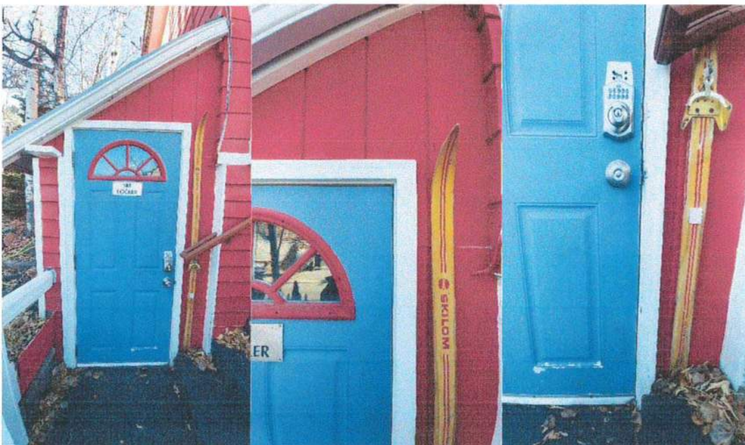
Photo 16: Basement Entrance Door (Door E3) Non-Historic Addition
