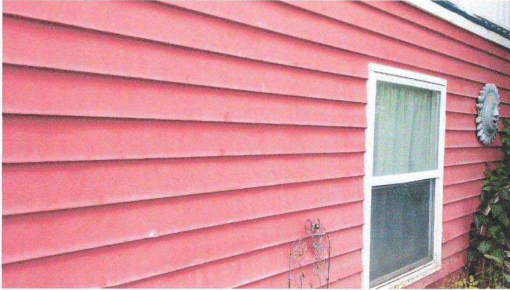
Photo 5: Siding and Window Trim
