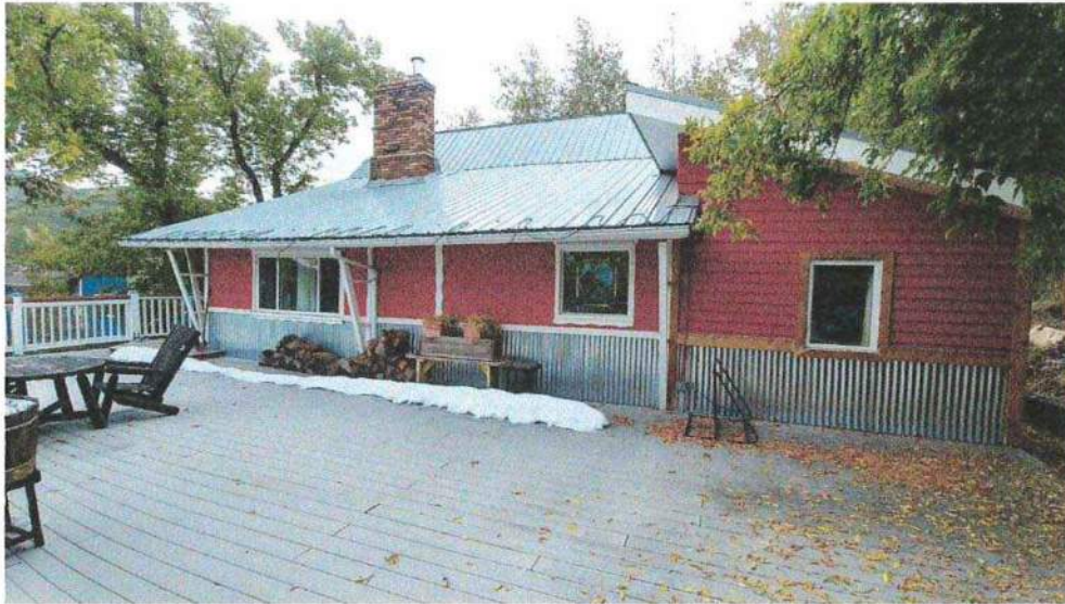
Photo 7: Roof and Non Historic Addition
