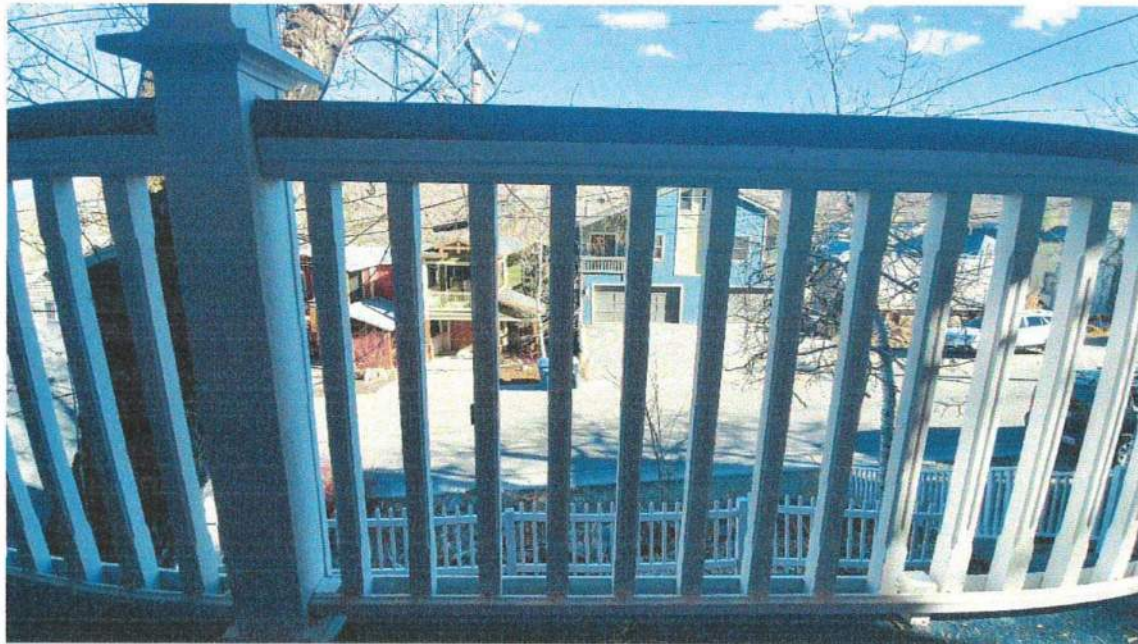
Photo 14: Front Porch Railing
