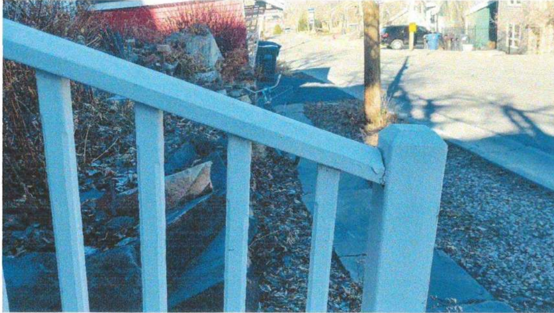
Photo 11: Front Railing Steps
