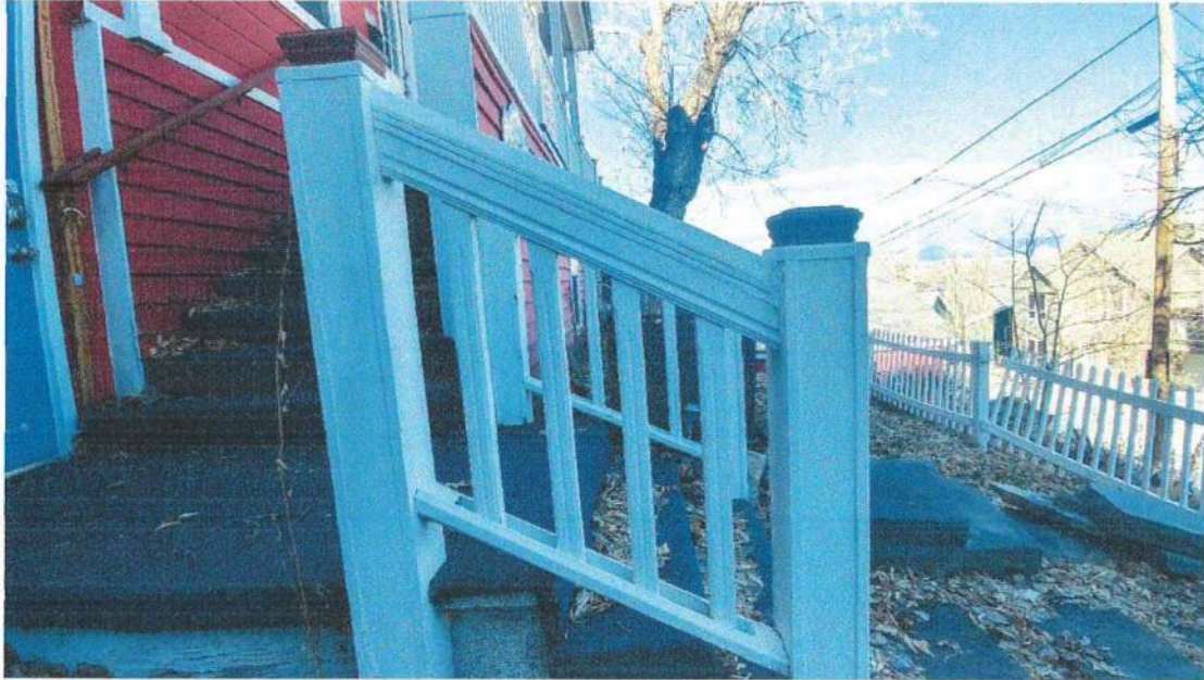
Photo 13: Railing to Front Porch
