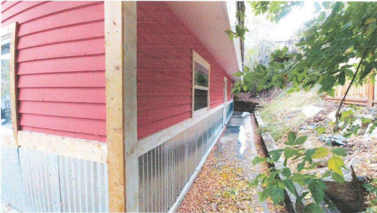
Photo 6: Rear View of Existing Home Non-Historic Addition
