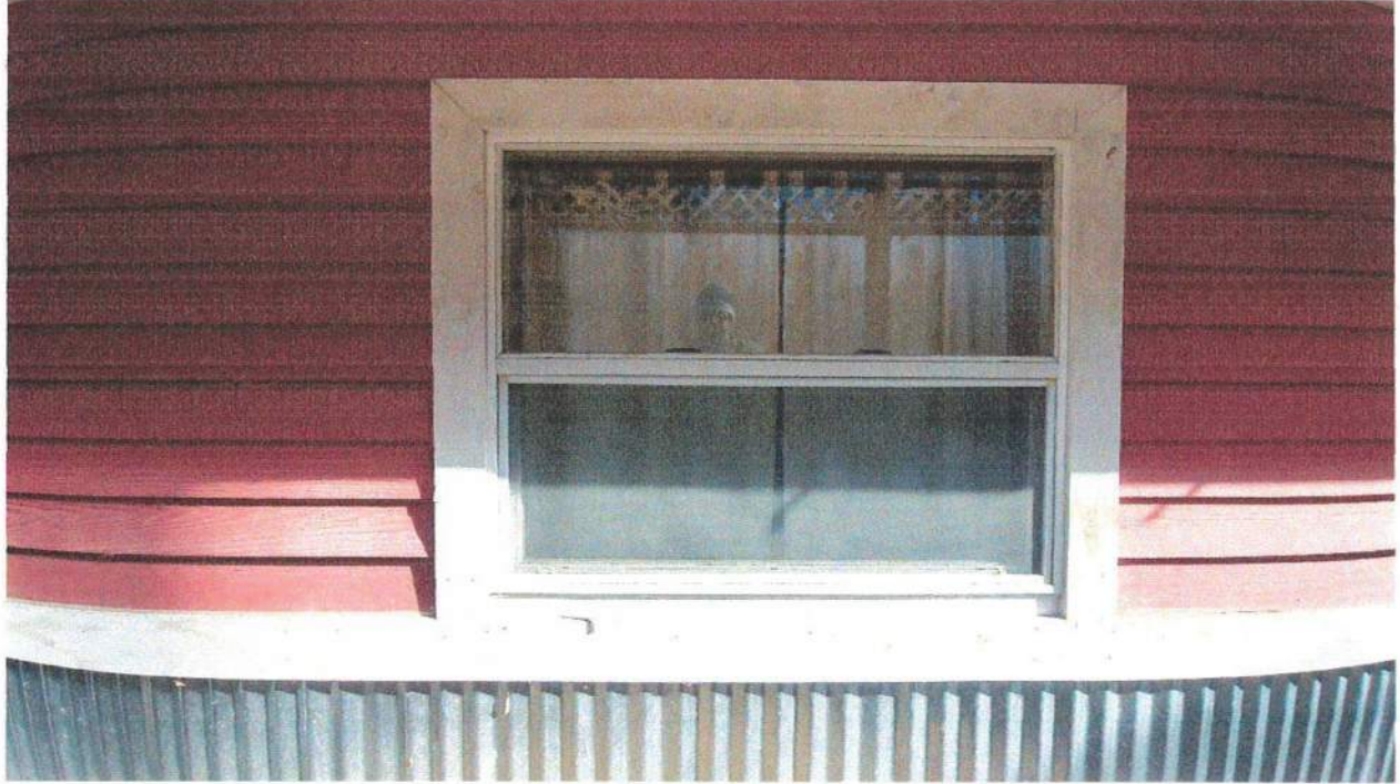
Photo 23: Rear (Window E-207) Non-Historic Addition
