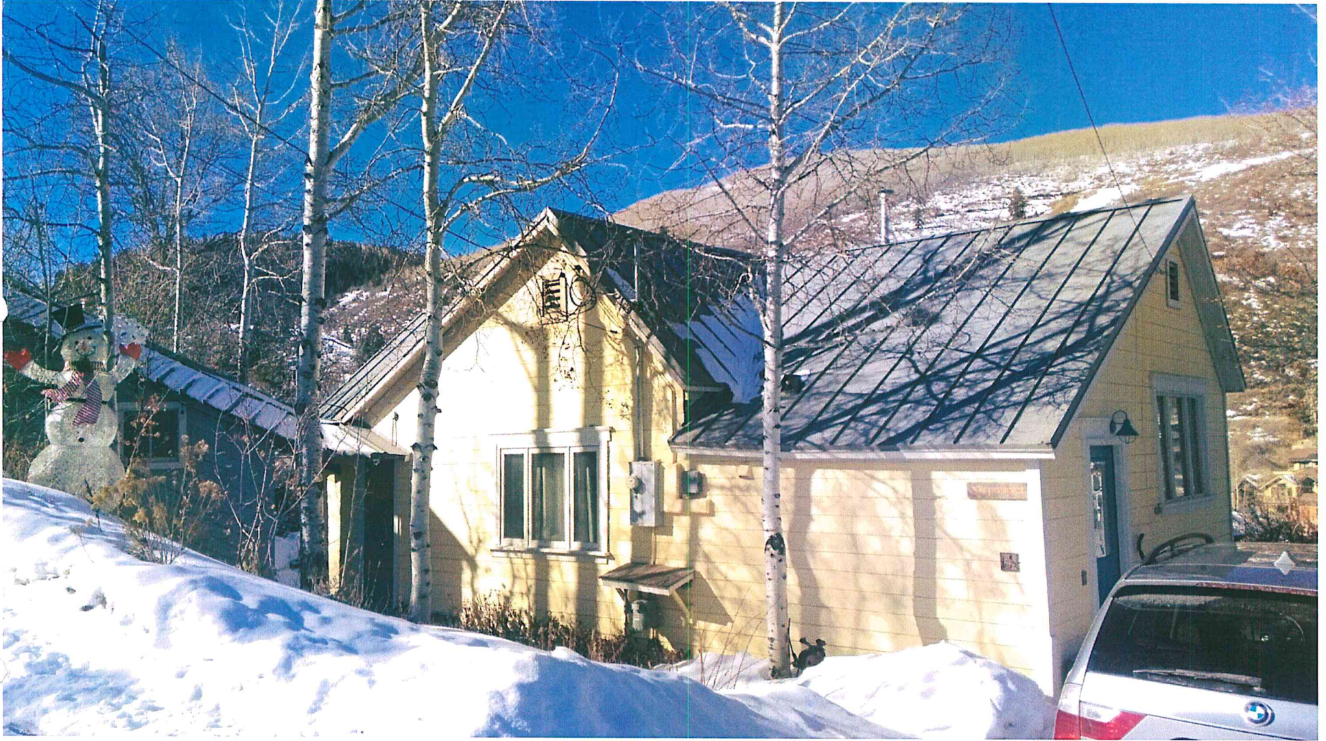
86 Prospect Street - Looking southwesterly
