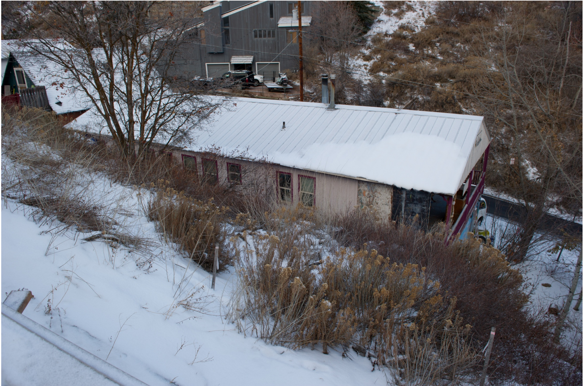
89 King Road - looking westerly
