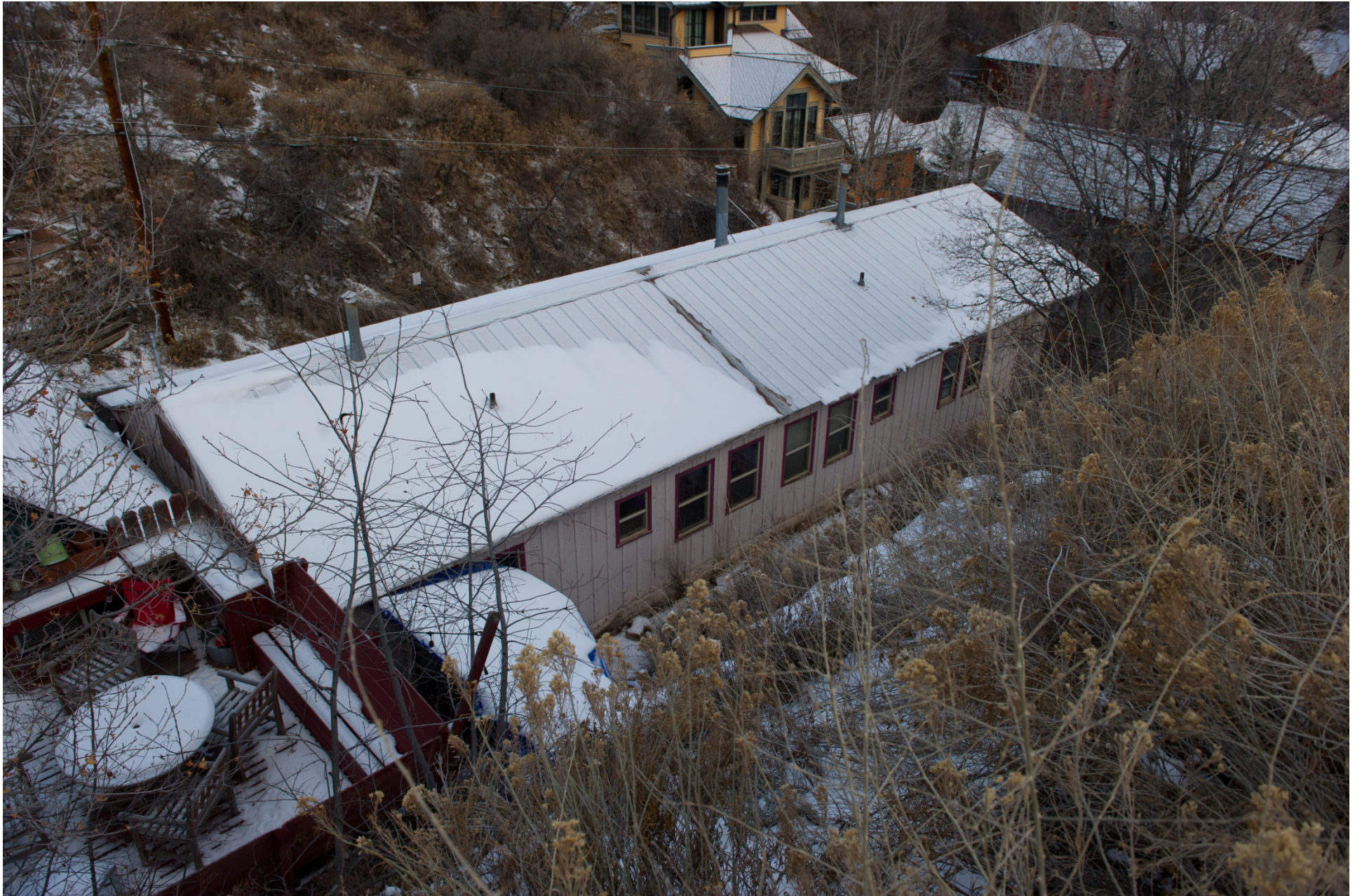
89 King Road - looking northwesterly
