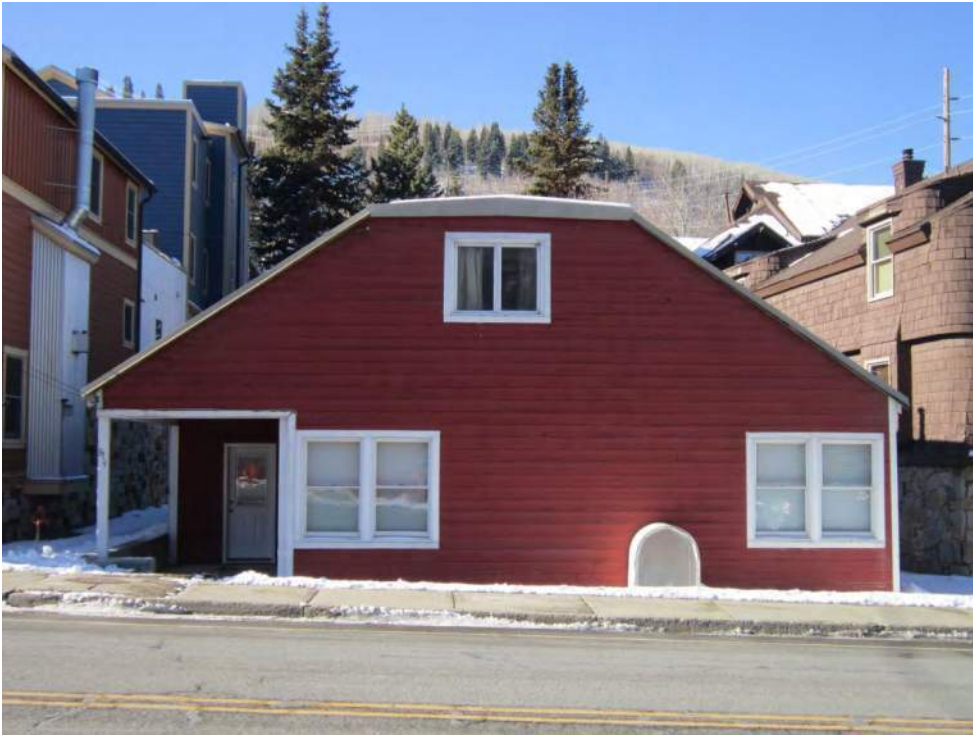
819 Park Avenue. East elevation. November 2013.
