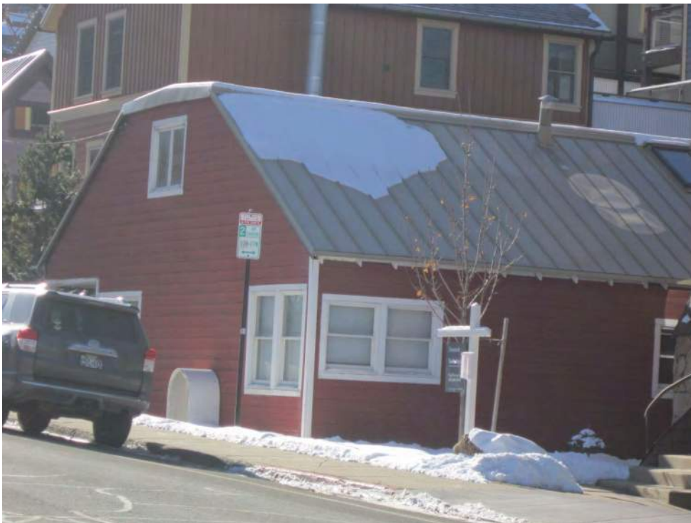
819 Park Avenue. Northeast oblique. November 2013.
