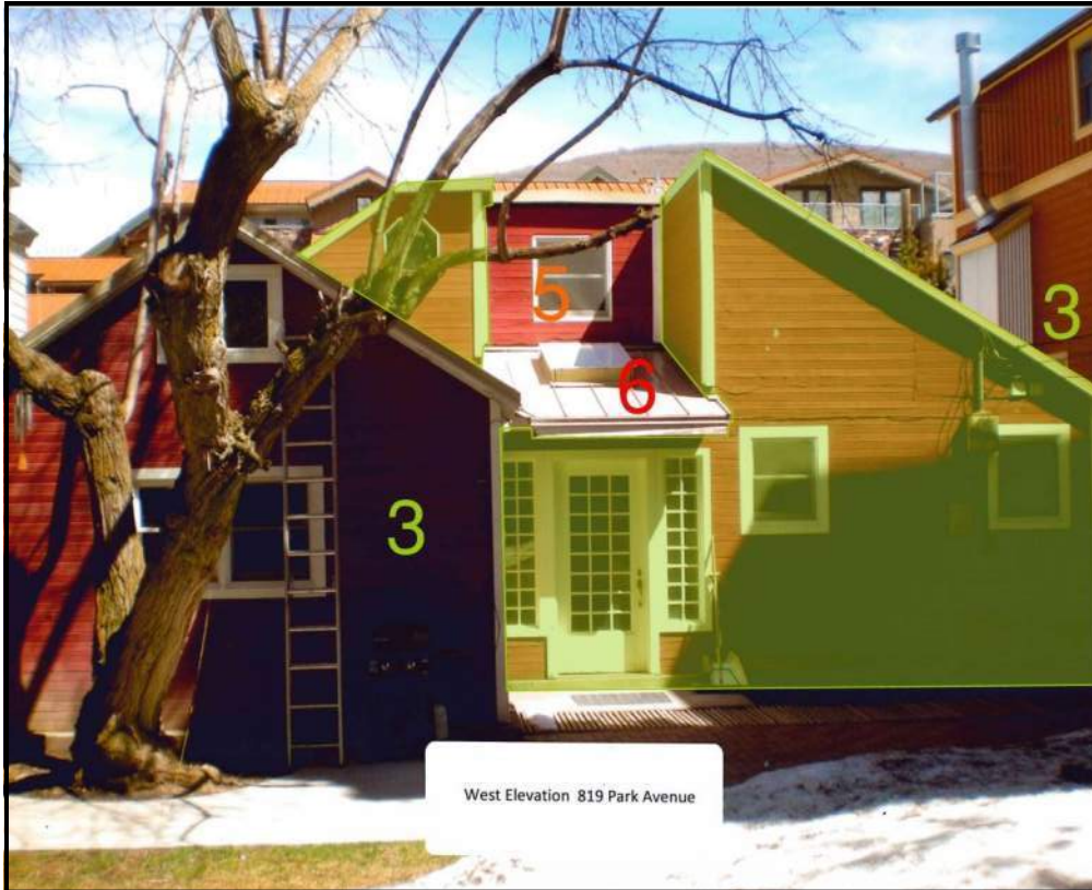
3. In-line addition to the rear of the building, 1974; 5. Asphalt shingle siding replaced with new wood siding, 1990s; 6. New roof and skylights, 2003.
