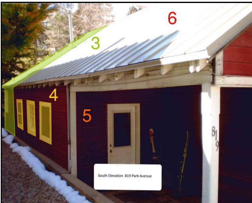
3. Rear addition to the house and storage shed remodeled as habitable space, 1974; 4. Window changes, 1984; 5. Asphalt shingle siding replaced with new wood siding, 1990s; 6. Skylights and new roof, 2003.
