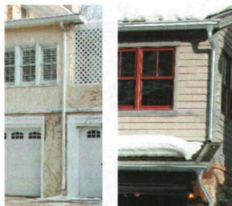
Gutters match trim or are appropriate for the architectural style
