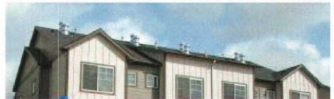
Mechanical vents reflect architectural style
