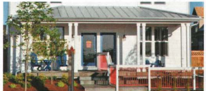
Properly detailed porch elements
