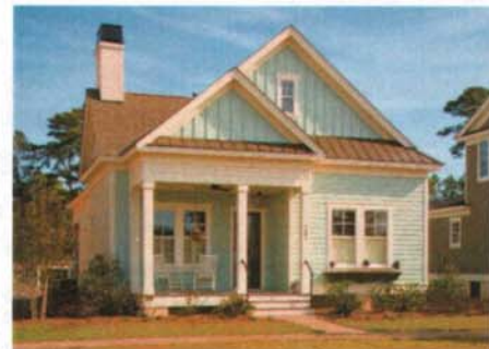
Porch roof forms are consistent with home
