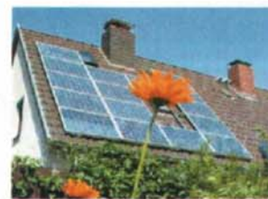
Solar panels visual impacts are minimized
