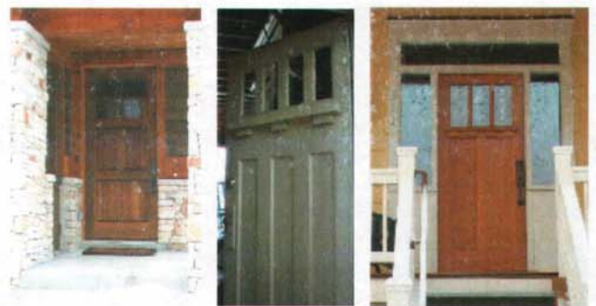
Doors should be significant architectural features of the Homestead homes
