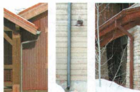
Gutters must complement the homes style
