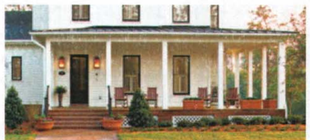
Porch raised above finished grade
