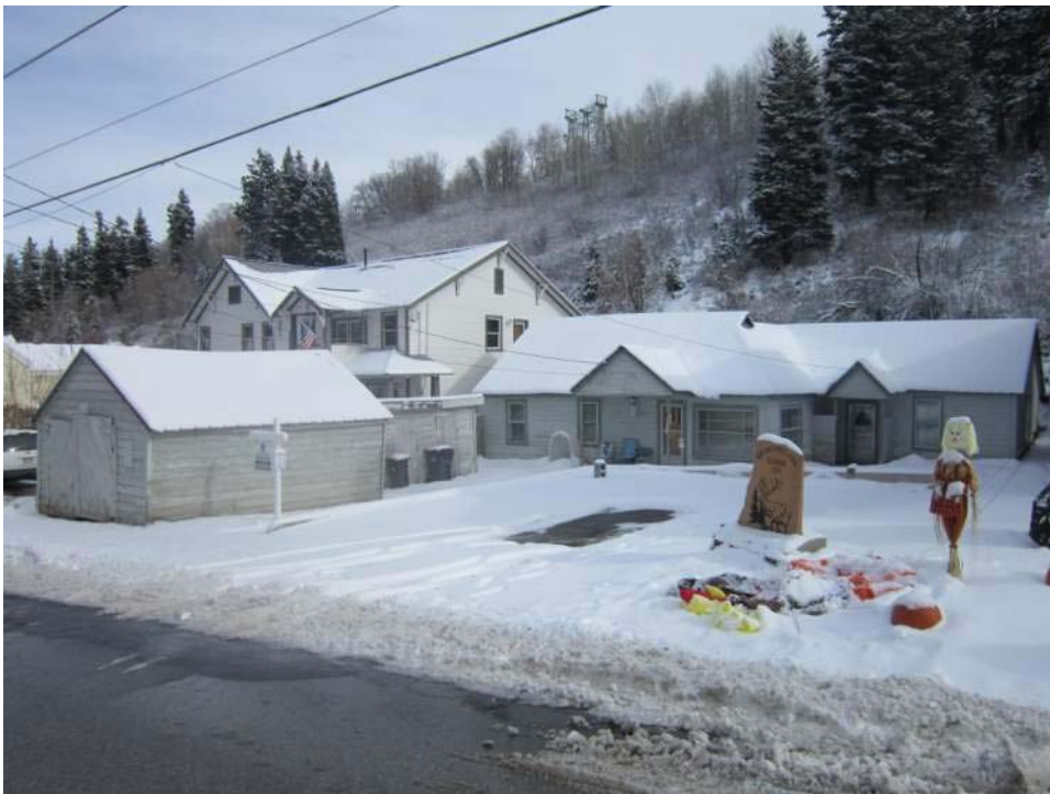
173 Daly Avenue. Southwest oblique. November 2013.
