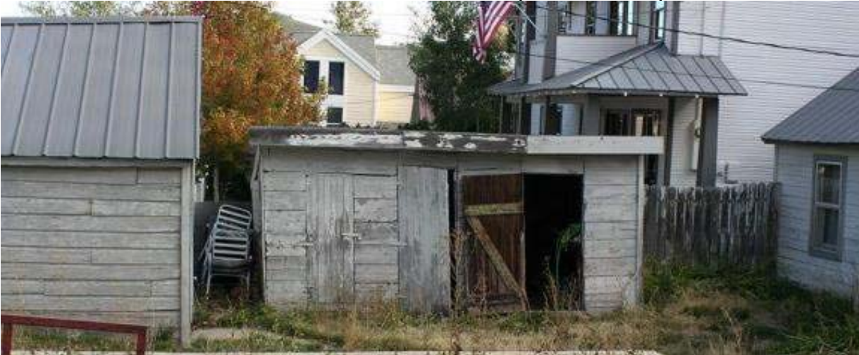
Historic Shed: North Elevation
