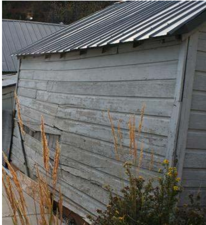
Figure 9: Detailed photograph of the non-historic siding that is to be removed from the Historic House.
