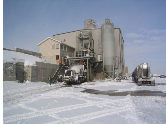
Loading Concrete Mixer Truck
