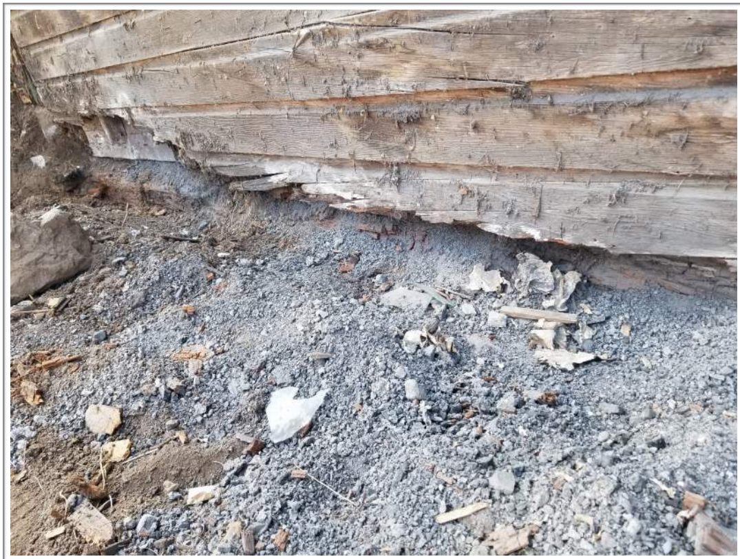
Photo #13: Deteriorated Foundation and Ash Mixture
