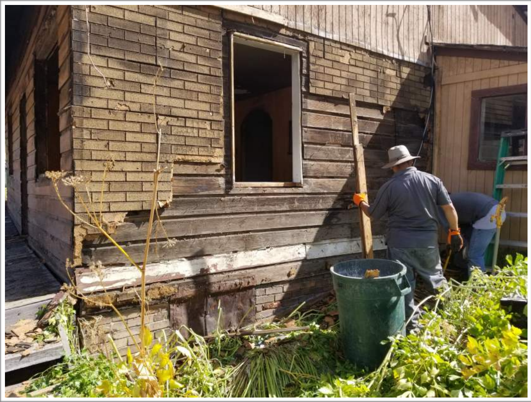
Photo #24 East Elevation Siding Removal
