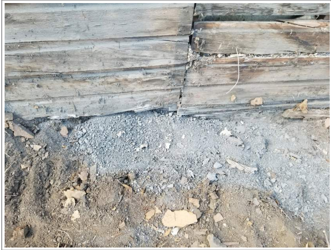
Photo #13: Deteriorated Foundation and Ash Mixture
