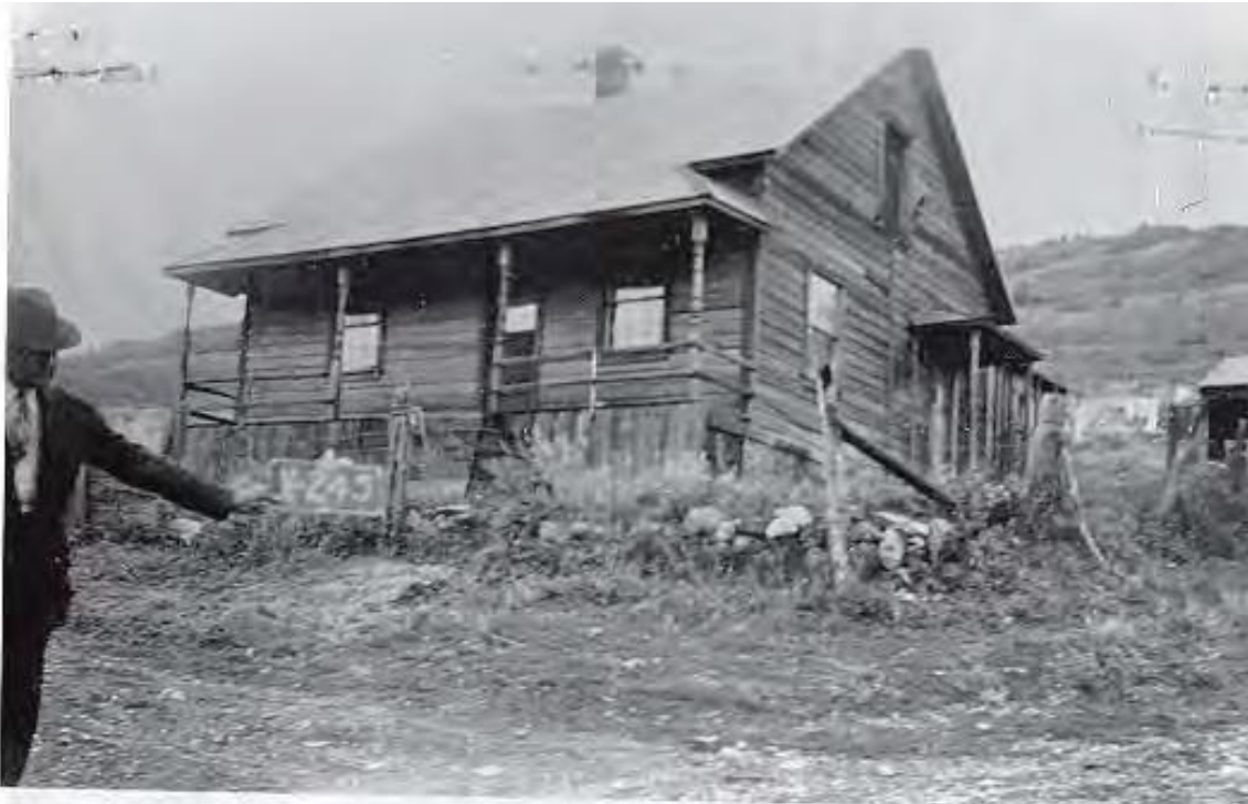
Above: The c.1941 tax photograph of the building.
