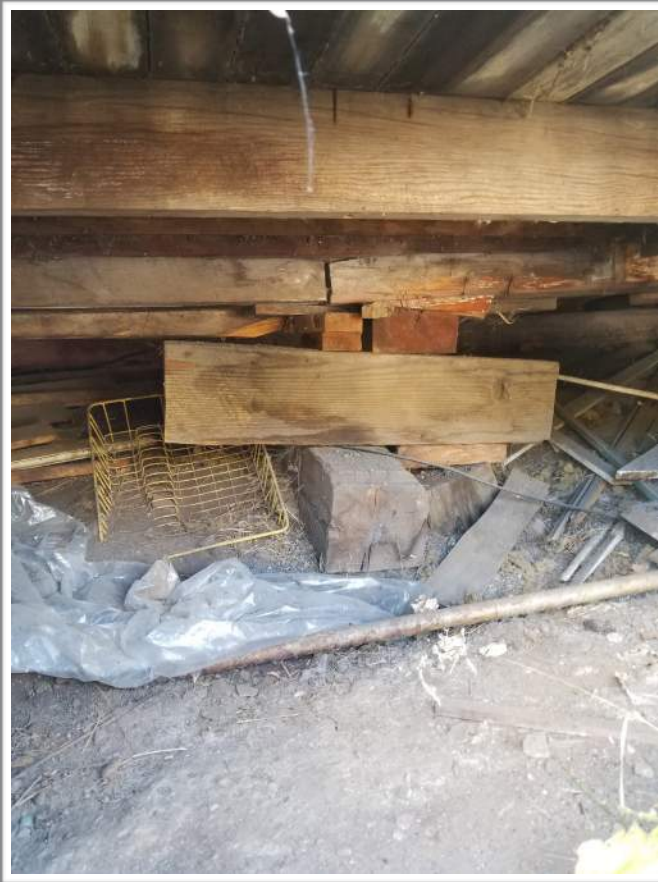
Photo #12 Ash Mixture Exiting Structure
