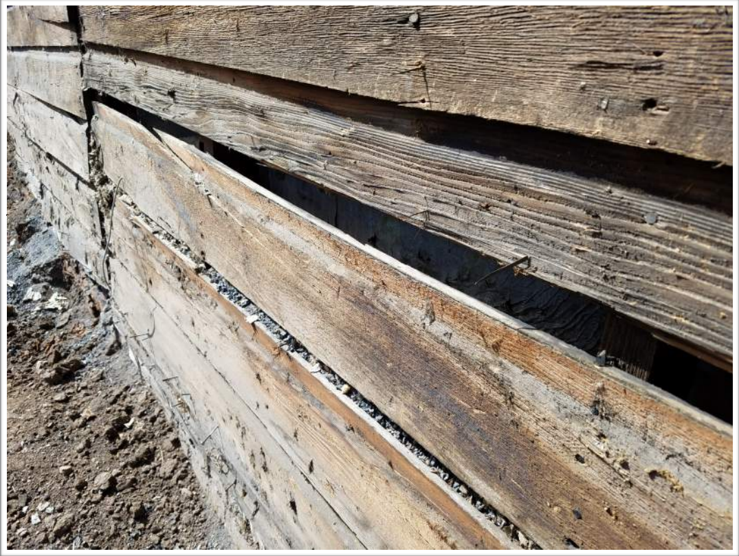
Photo #25 East Facade Siding Condition
