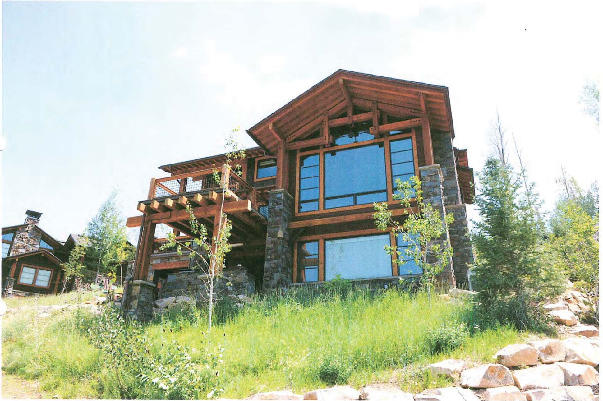
Unit 8 (11 Nakoma Terrace) – looking southeasterly
