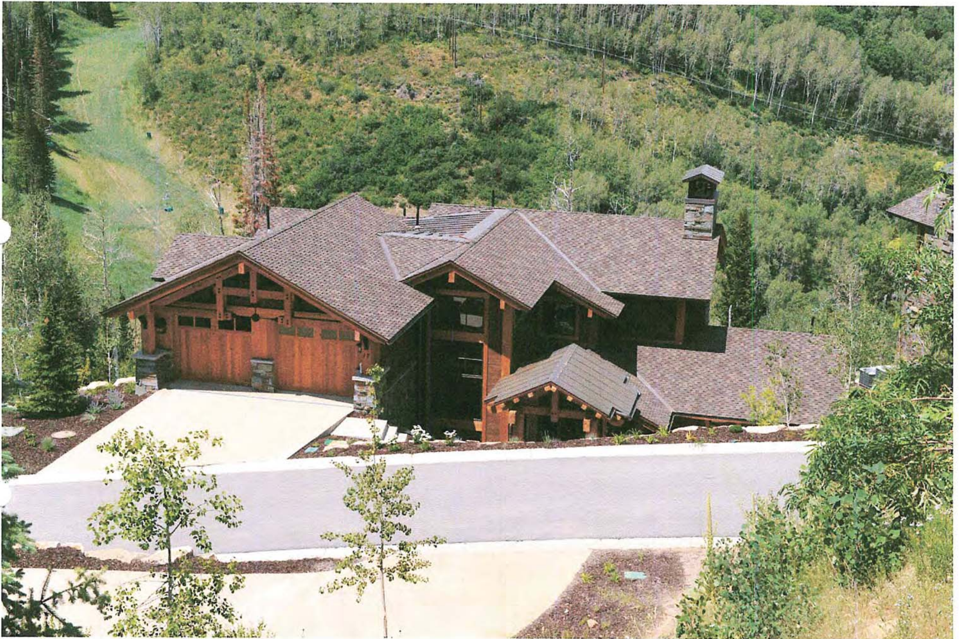
Unit 7 (17 Nakoma Terrace) – looking northwesterly
