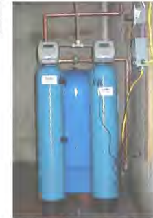
Use of E33 media in typical point-of-entry system installation. Picture courtesy of Aquamech, Inc.
