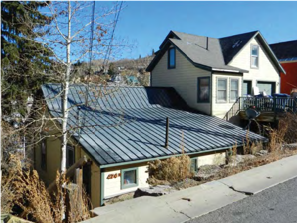
424 Woodside Avenue. Northwest oblique. November 2013.
