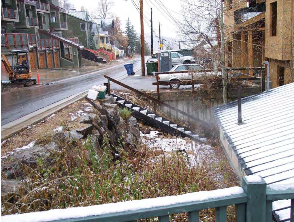
Rock retaining wall and entry stairs along west elevation
