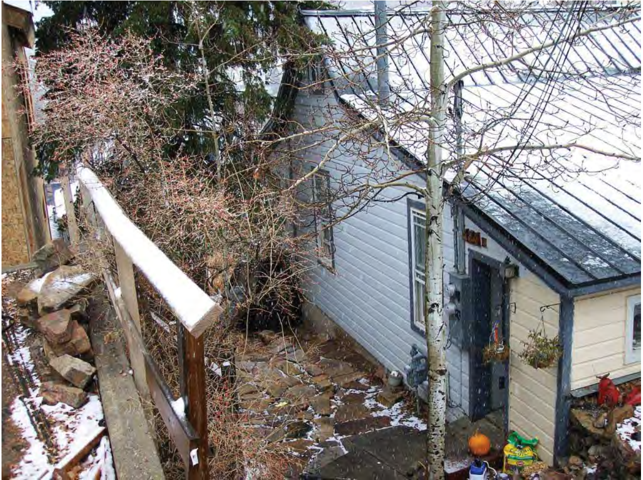
Roof looking southeast
