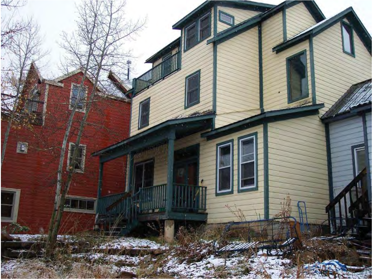
Addition on the south elevation built after 1993
