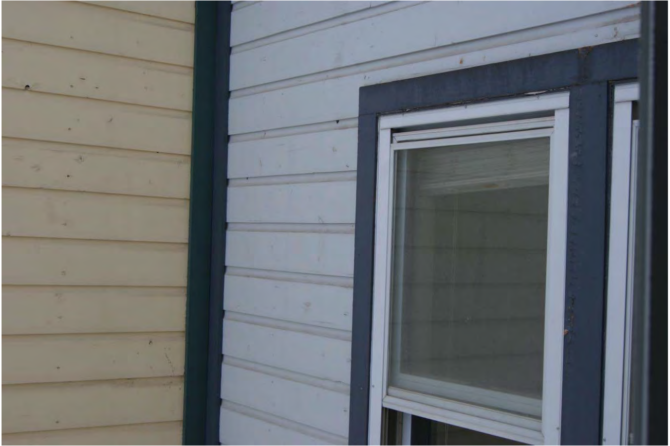
Wood aluminum clad window- typical
