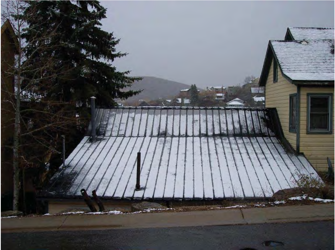
Roof looking east
