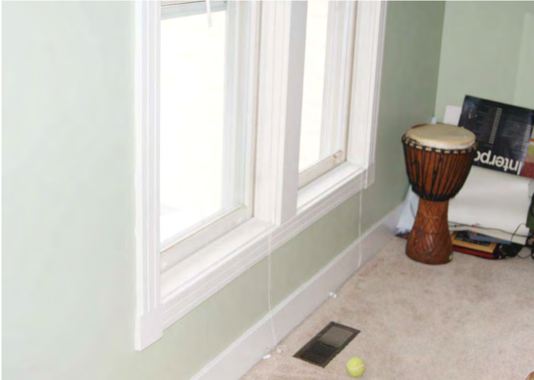
Typical base and window casing
