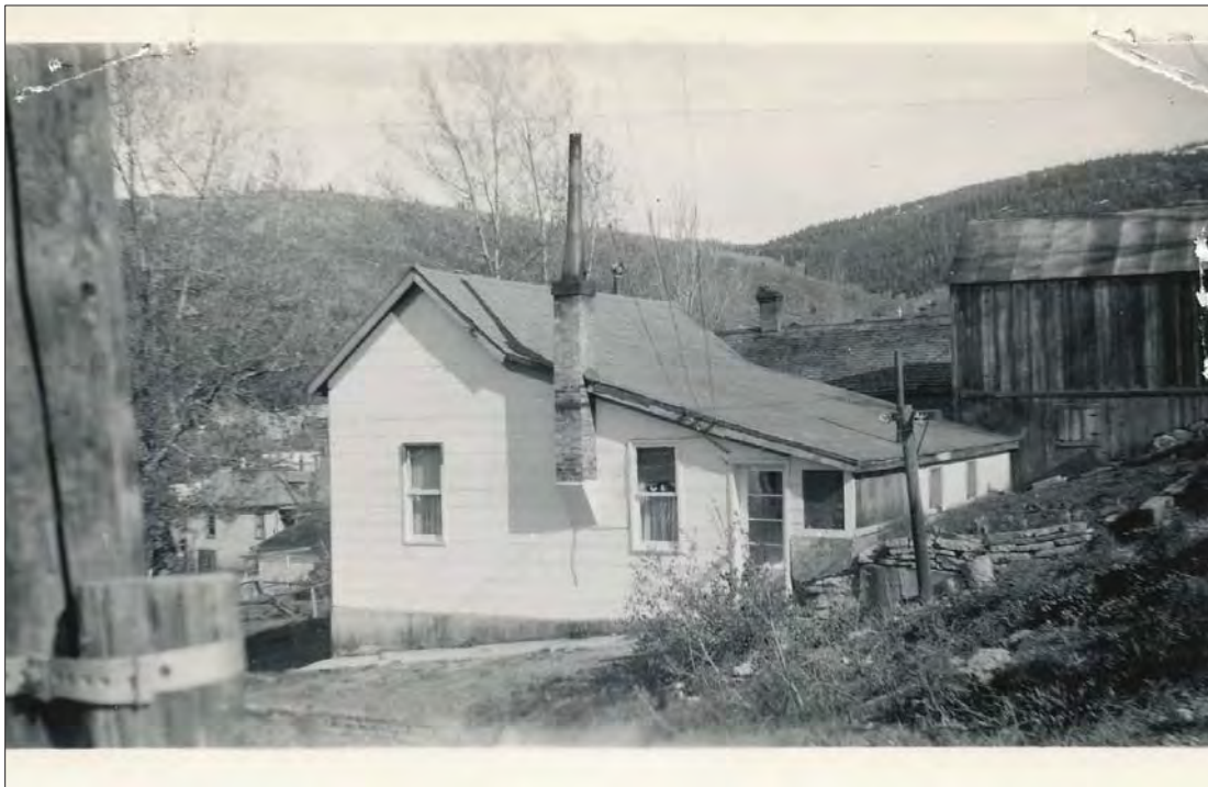
Figure 5. Tax appraisal photograph of property at 424 Woodside dating to ca. 1941, facing southeast.
