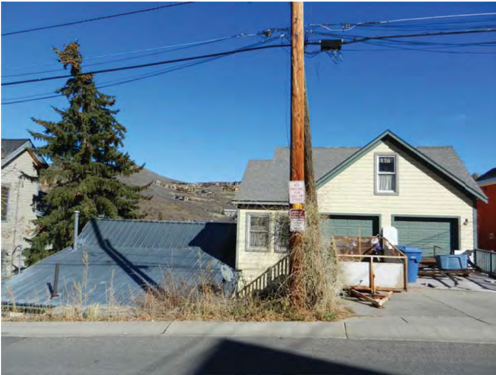
424 Woodside Avenue. West elevation. November 2013.
