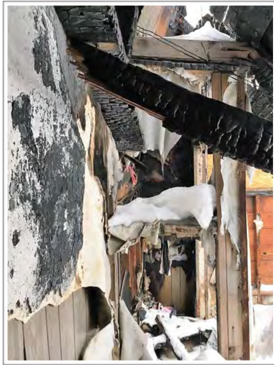
Photo #14: Fire Damage @ Rear Addition
