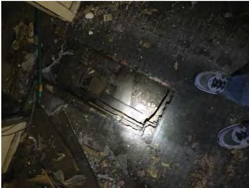
Figure 2- Existing floor framing conditions
