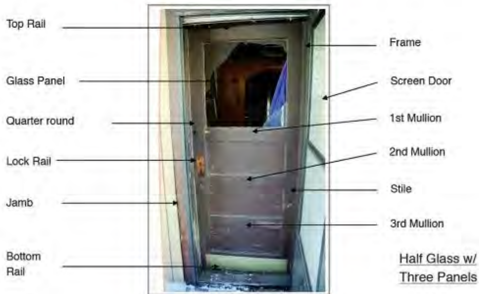
Historic front door proposed to be salvaged and reused.
