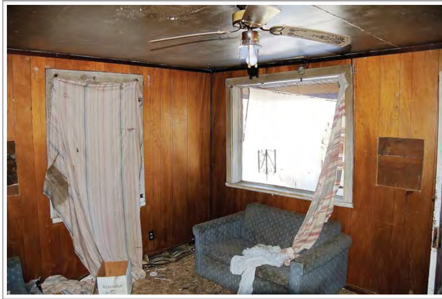
Photo #35: Interior Main Room (2)
