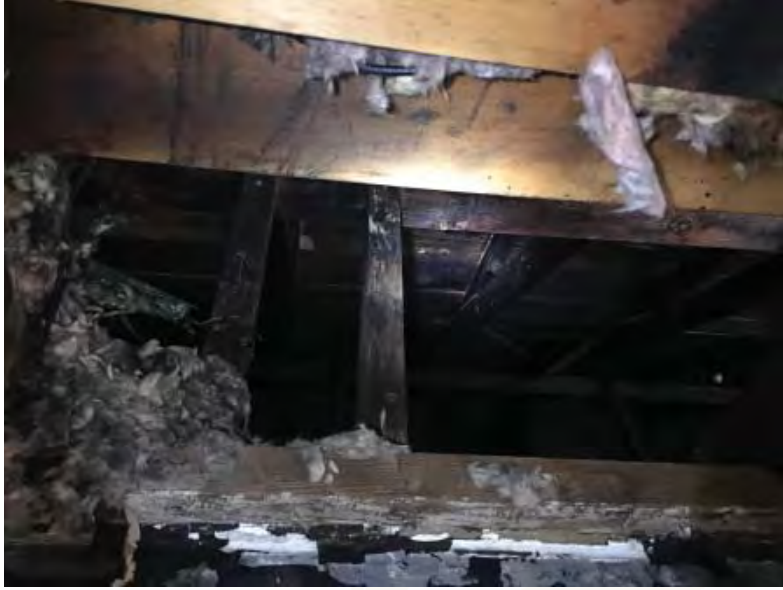
Figure 3 - South Perimeter Wall looking into Attic
