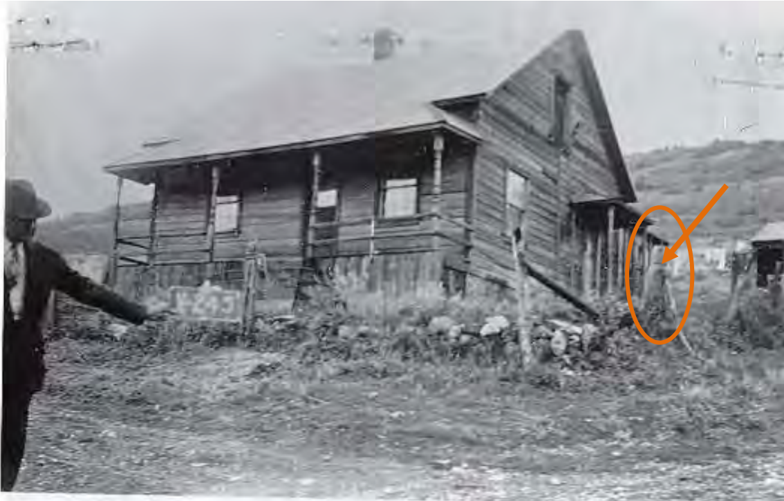
Above: The arrow denotes the structure to the back of the building c.1941. It is unclear if this is a short-lived addition or an unidentified outbuilding.
