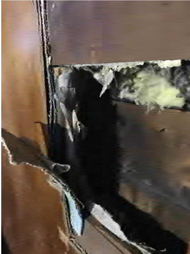
Figure 5 - Existing wall framing with lap board siding
