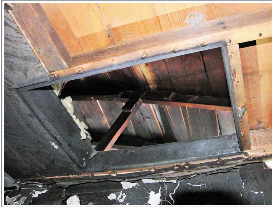
Photo #12: Chimney Flue @ Attic
