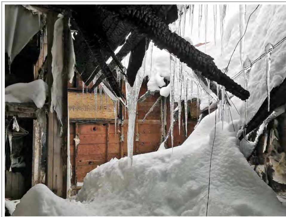
Photo #14: Fire Damage @ Rear Addition
