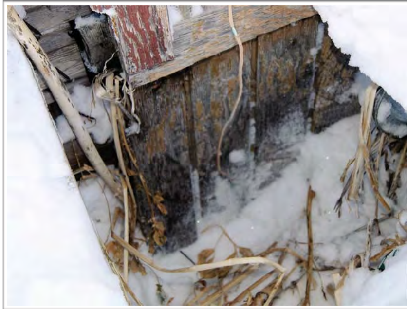
Photo #10: Floor Construction on Grade
