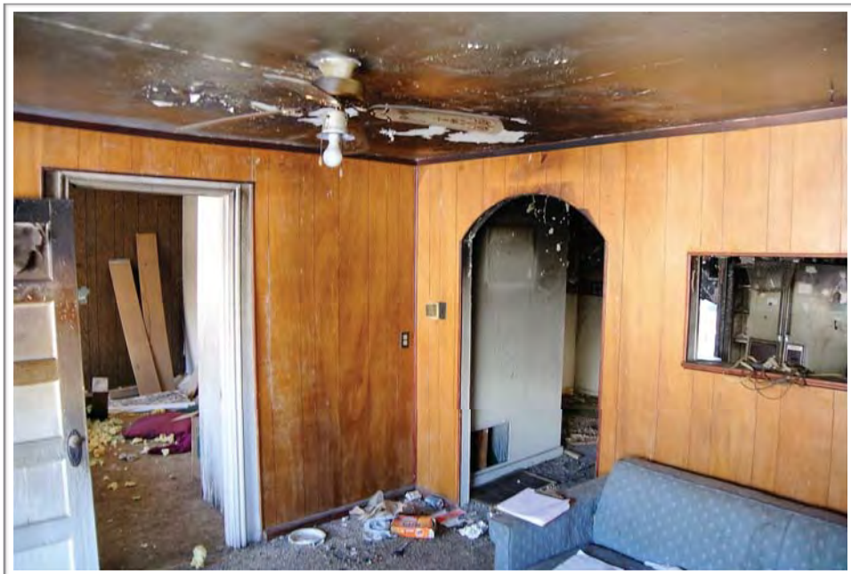
Photo #34: Interior Main Room (1)
