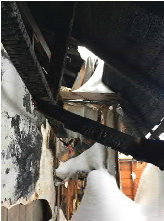
Figure 4 - South Area of roof
