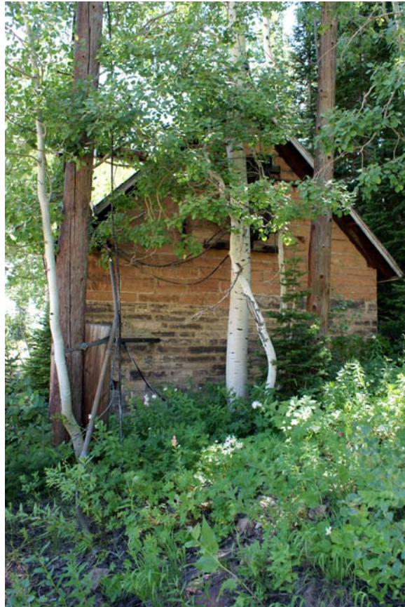
Transformer House (west elevation), 2009
