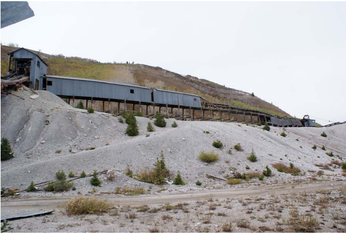
Conveyor Gallery extension, 2009
