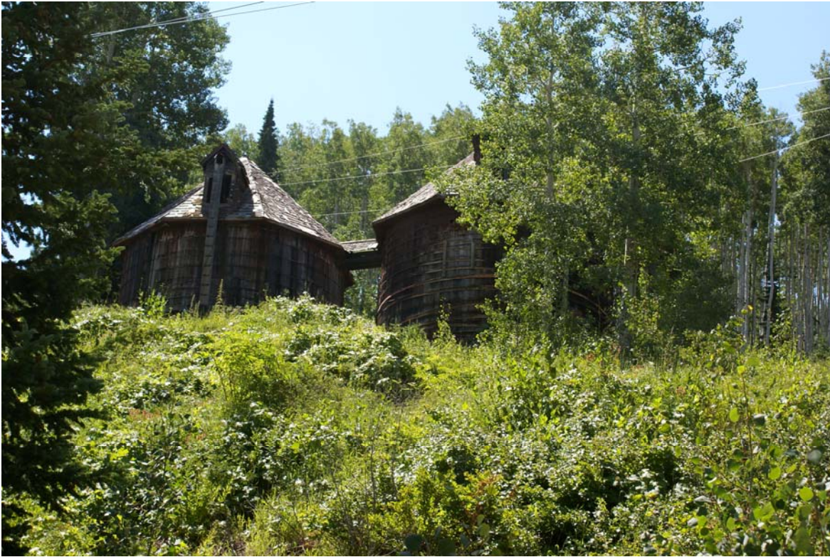
Water Tanks D & E (north elevation), 2009
