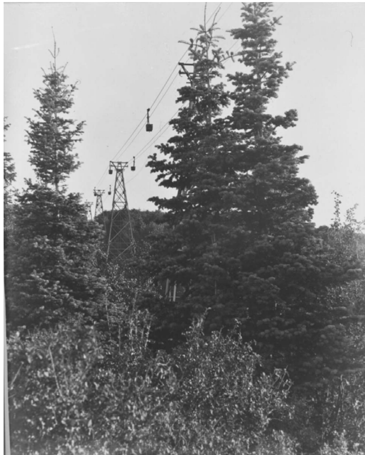
Silver King Aerial Tramway . N.d. Bea Kummer Collection . Hal Compton Research Library . Park City Historical Society & Museum. 10 Oct. 2009 Photo #1990.31.21. Electronic.
