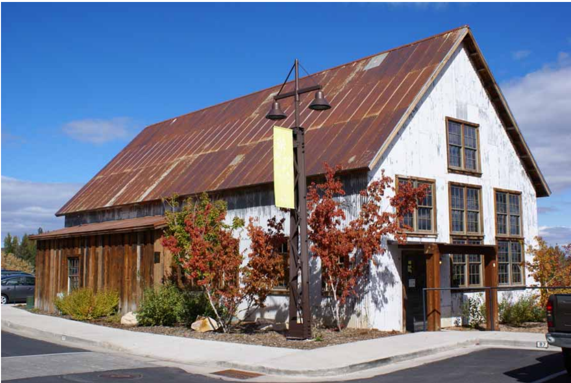
Silver King Consolidated Mine - Spiro Tunnel Site, Sawmill Building, 2006
