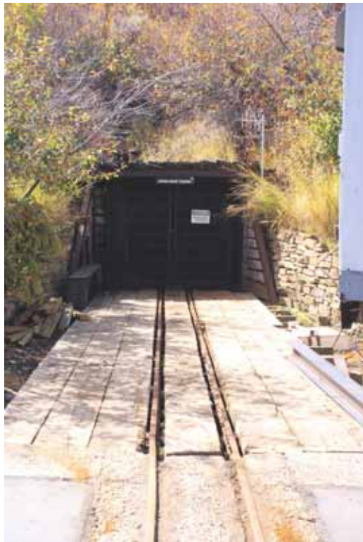
Silver King Consolidated Mine - Spiro Tunnel Site, Spiro Tunnel Portal, 2006
