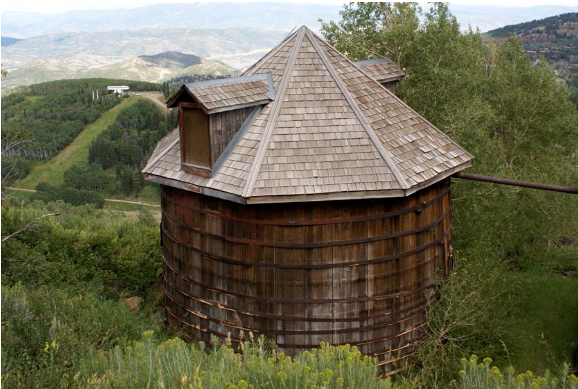
Water Tank A (southwest elevation), 2009
