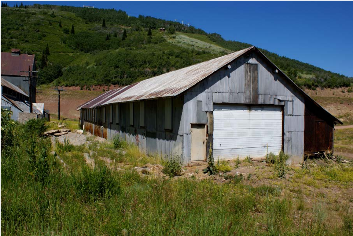
Stores Dept Building (southeast oblique), 2009
