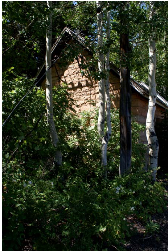
Transformer House (east elevation), 2009
