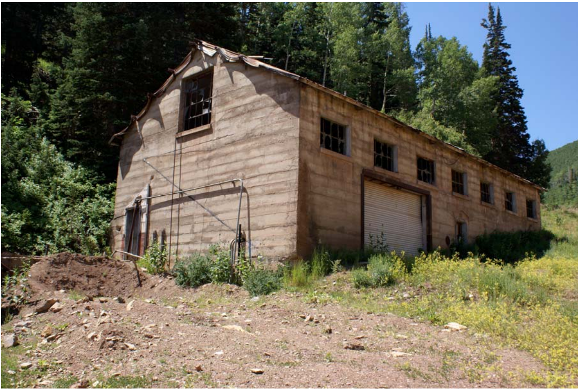
Change House (northeast oblique), 2009
