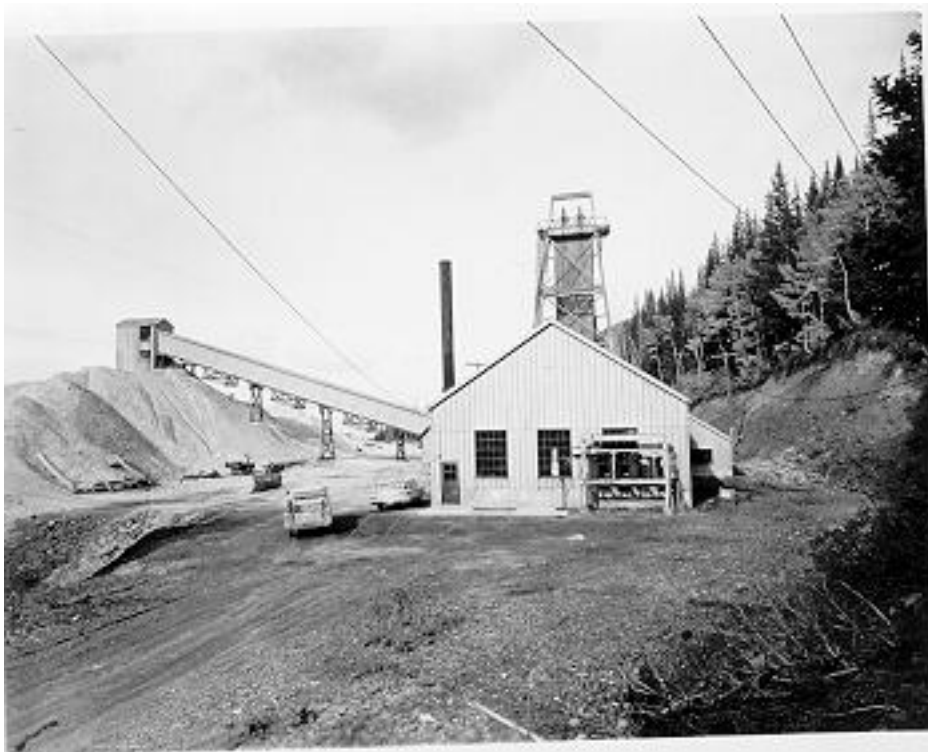
Thaynes Shaft Surface Plant - Silver King Coalition Mines Company. [c.1970?] Leon Stanley Collection. Hal Compton Research Library. Park City Historical Society & Museum. 10 Oct. 2009. Photo #1990.5.27. Electronic.
