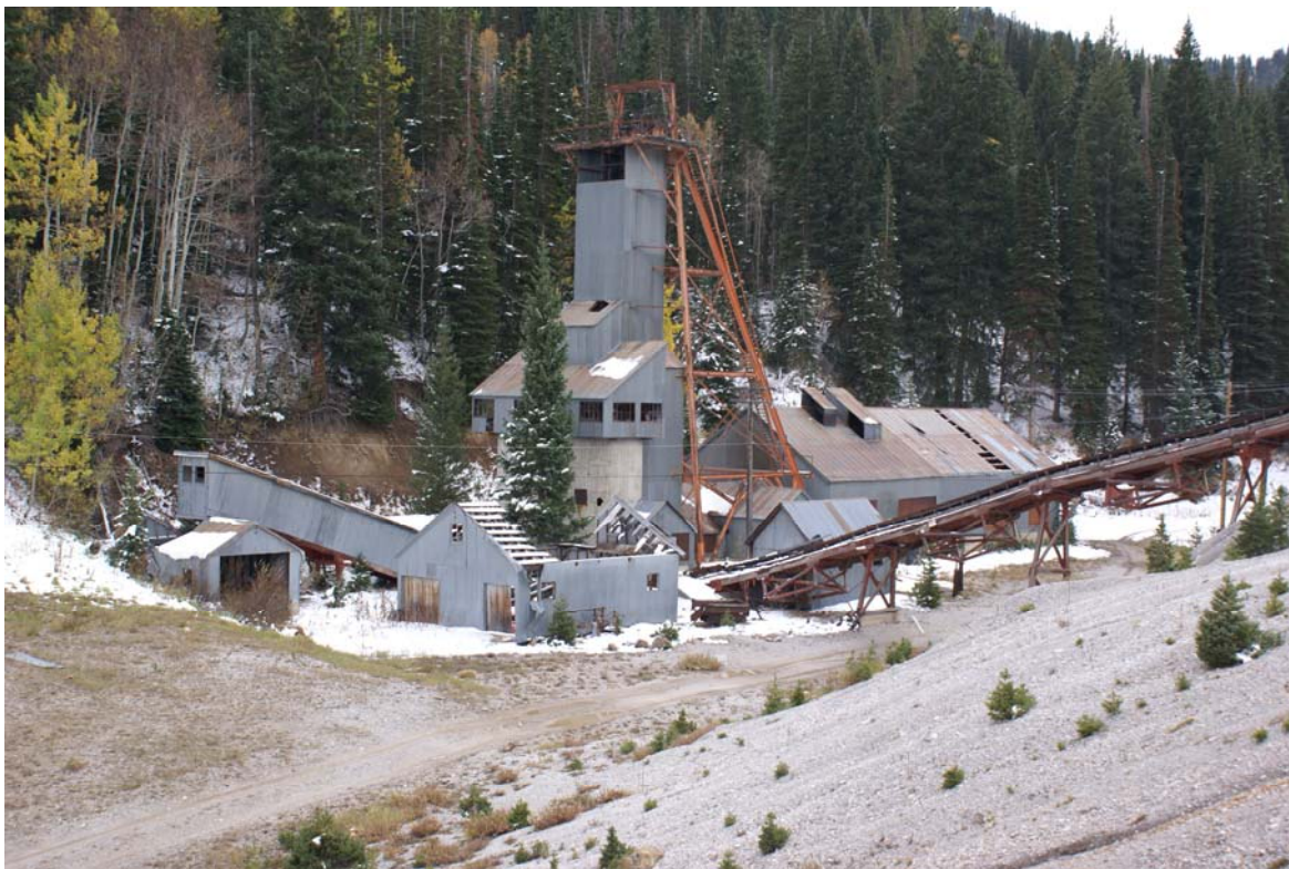
Hoist House (north oblique), 2009
