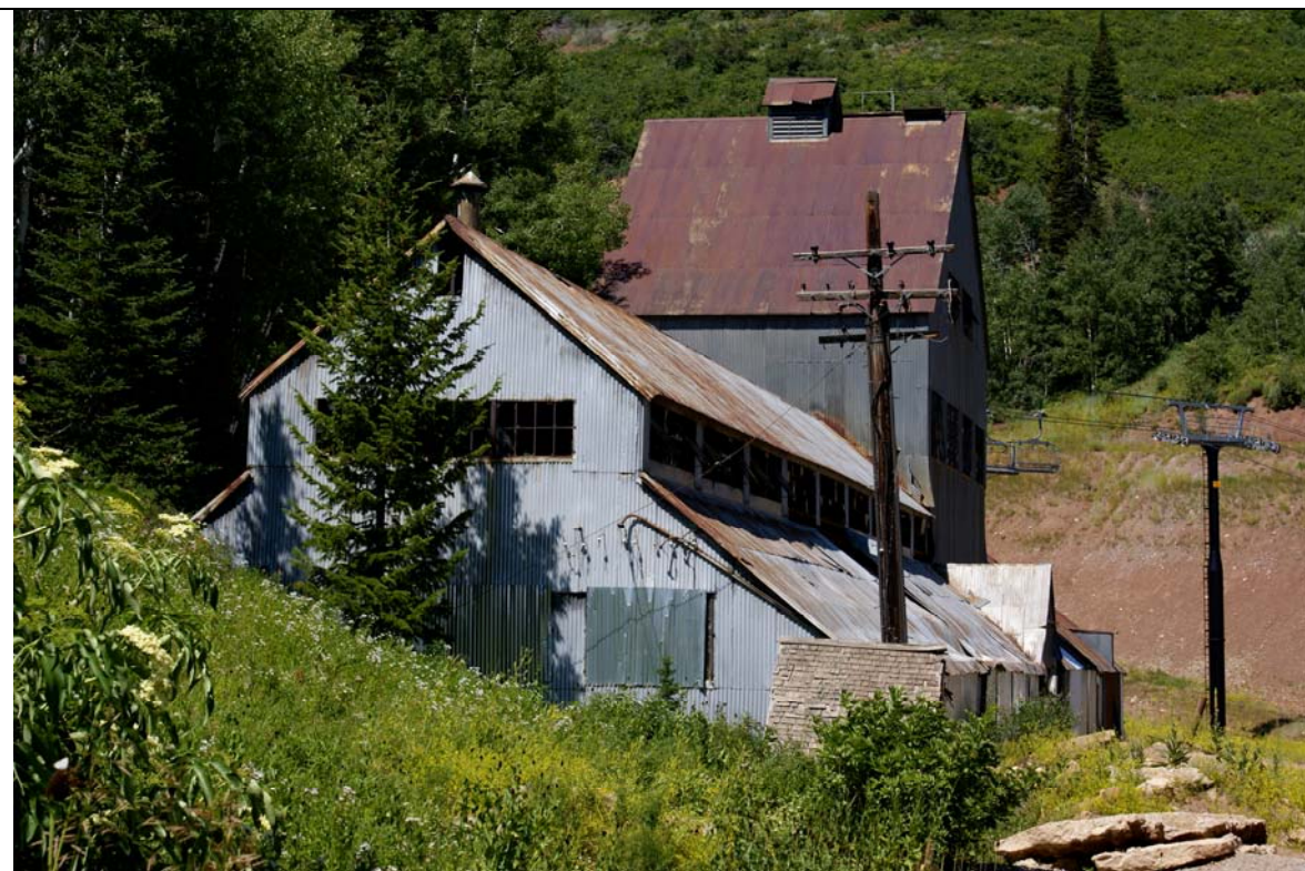
Hoist House (east elevation), 2009
