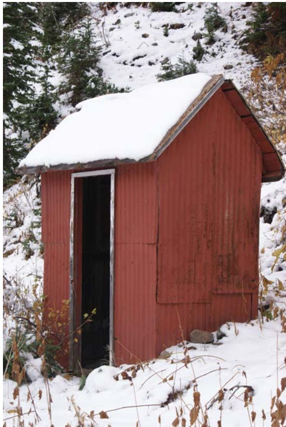
Fire Hydrant Shack (west oblique), 2009
