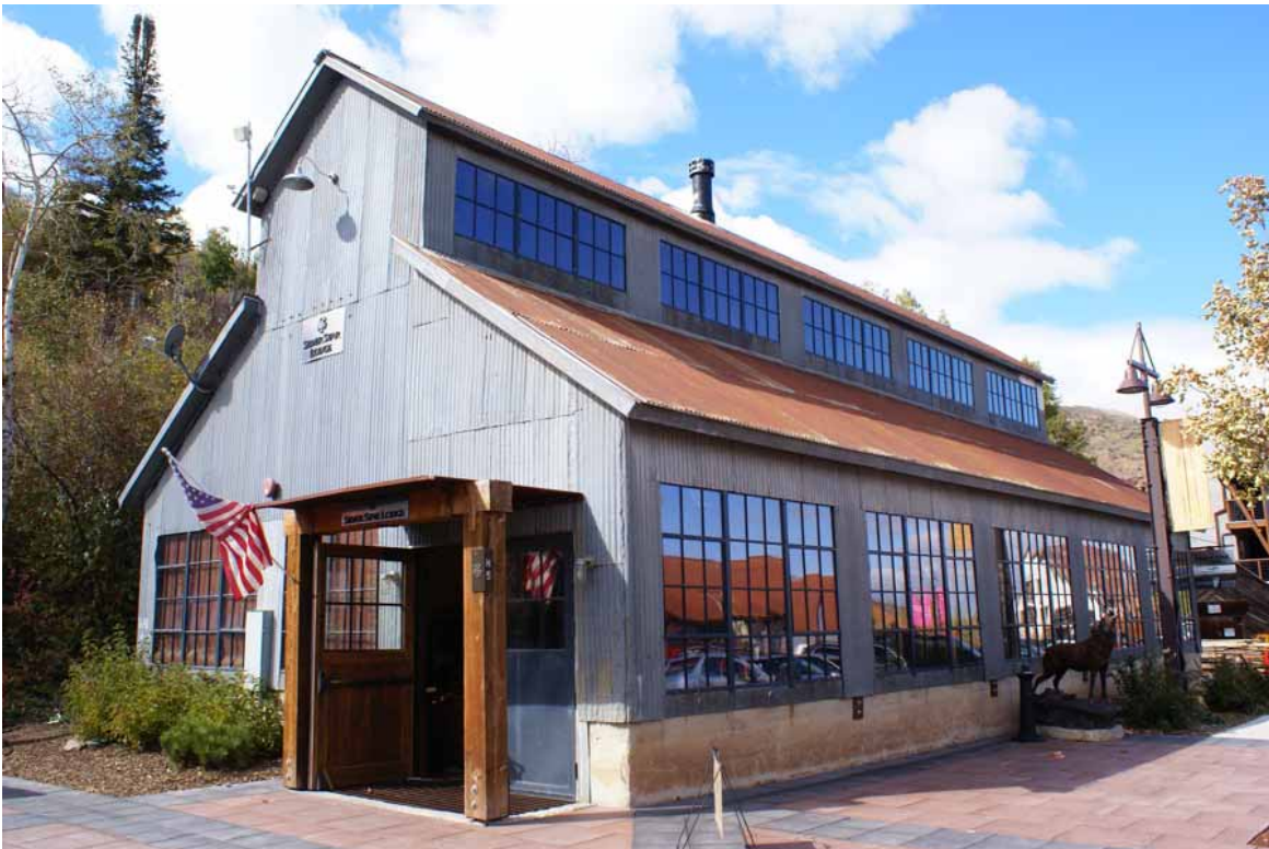
Silver King Consolidated Mine - Spiro Tunnel Site, Compressor House A, 2006
