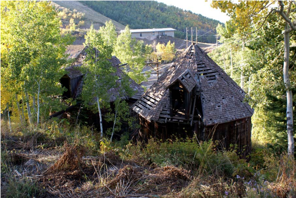
Water Tanks D & E (south elevation), 2009
