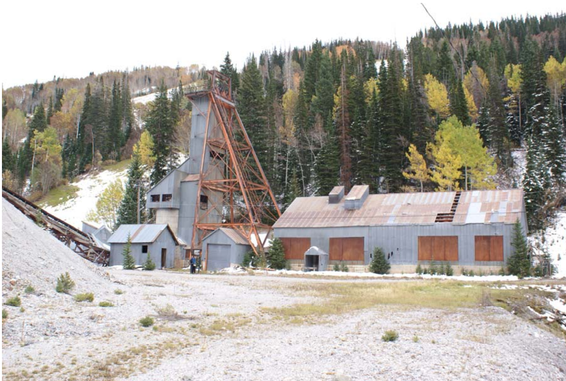
Hoist House (west oblique), 2009
