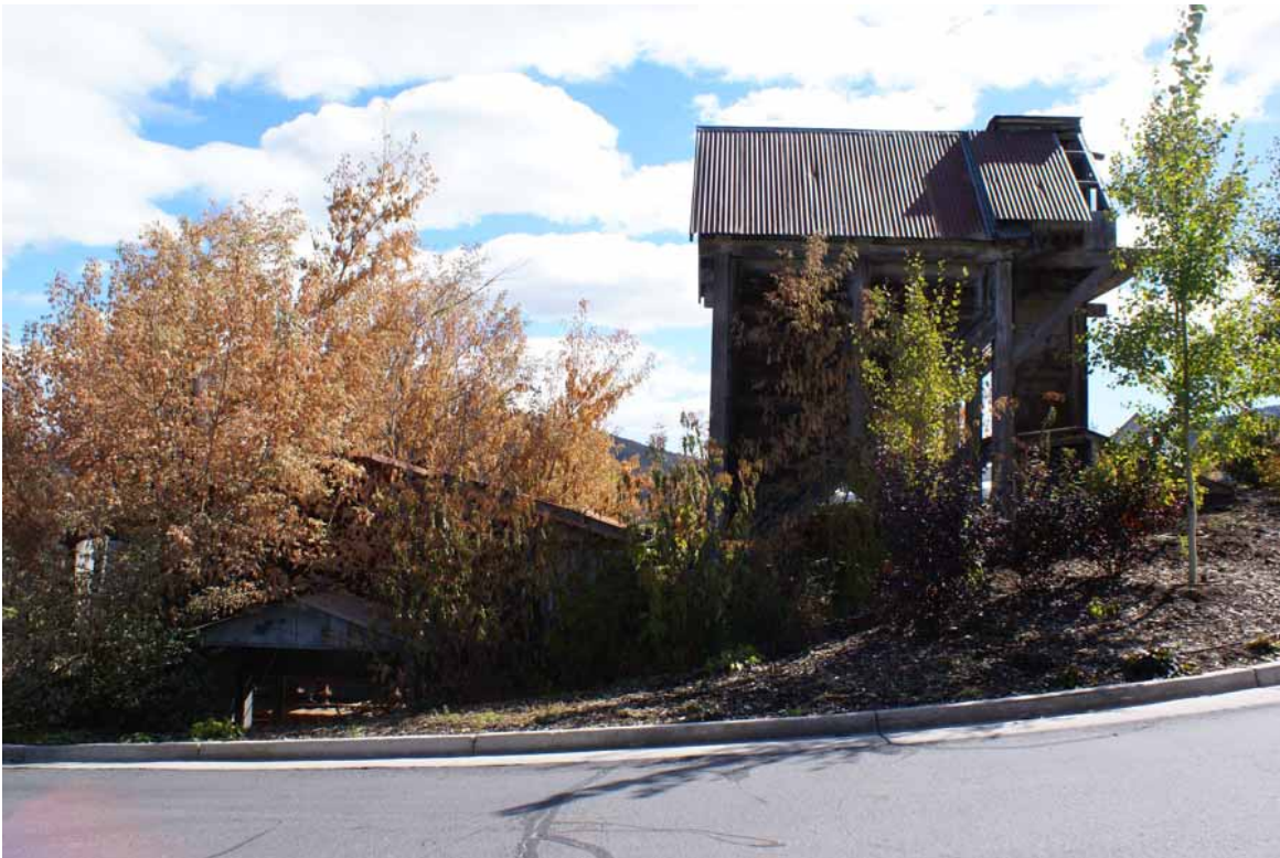
Silver King Consolidated Mine - Spiro Tunnel Site, Heating Plant-Coal Bin, 2006
