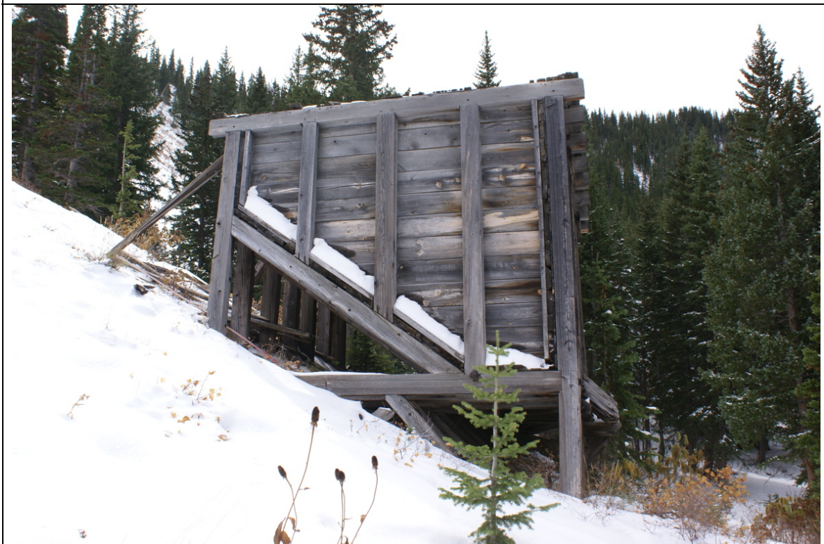
Jupiter Mine Ore Bin (northeast elevation), 2009
