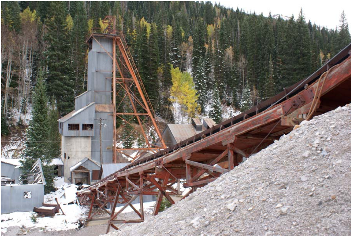
Conveyor Gallery detail (northwest elevation), 2009
