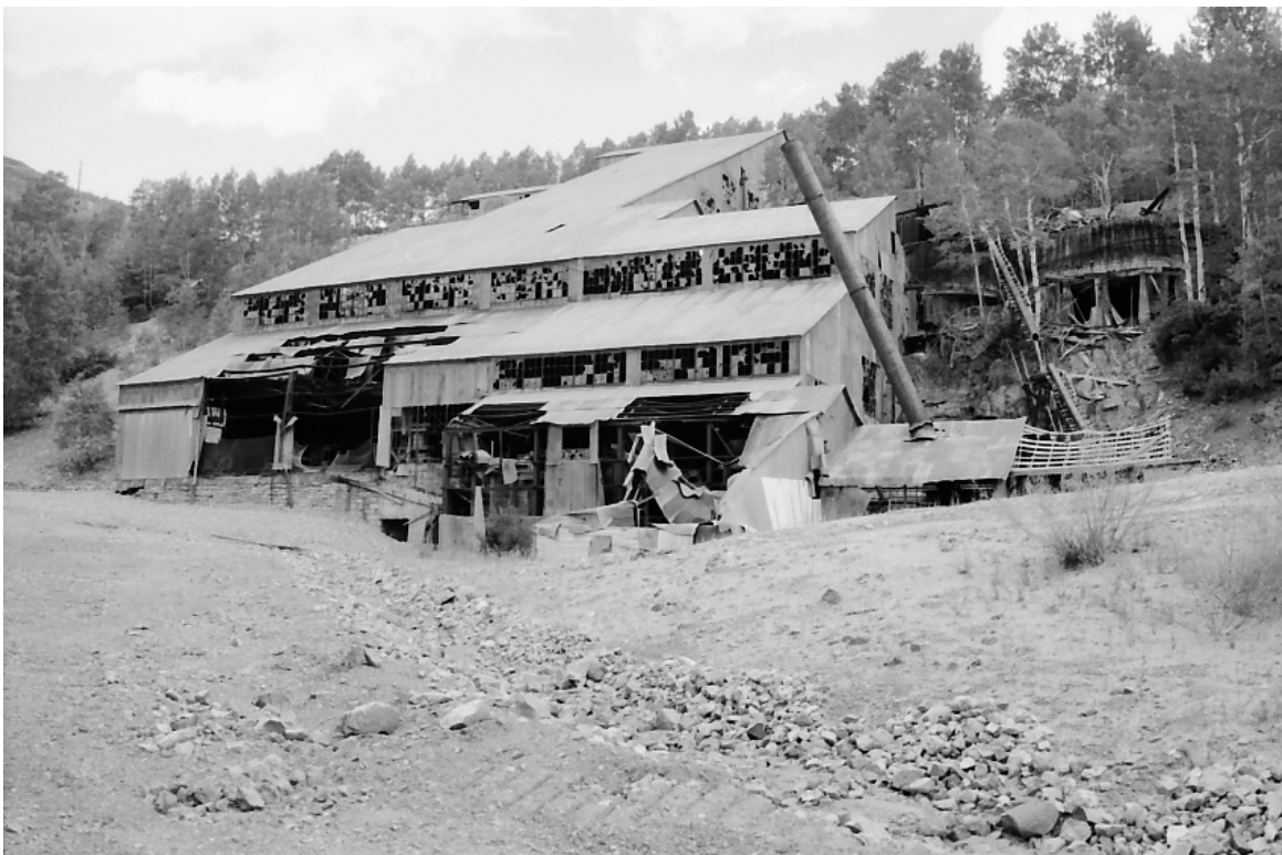
Mill Building (southeast oblique), 1999
