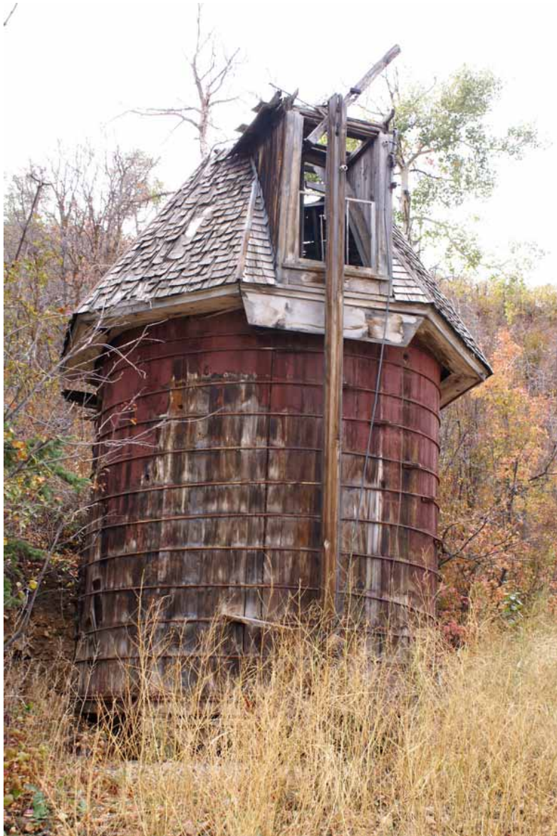
Silver King Consolidated Mine - Spiro Tunnel Site, Water Tank, 2006
