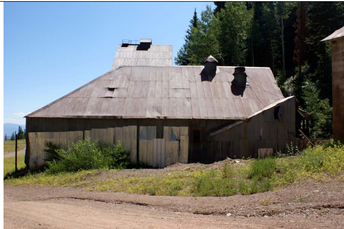
Hoist House (west elevation), 2009
