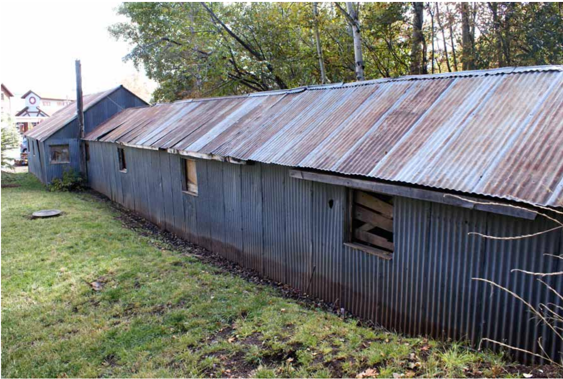
Silver King Consolidated Mine - Spiro Tunnel Site, Ivers Tunnel Portal Structure, 2006
