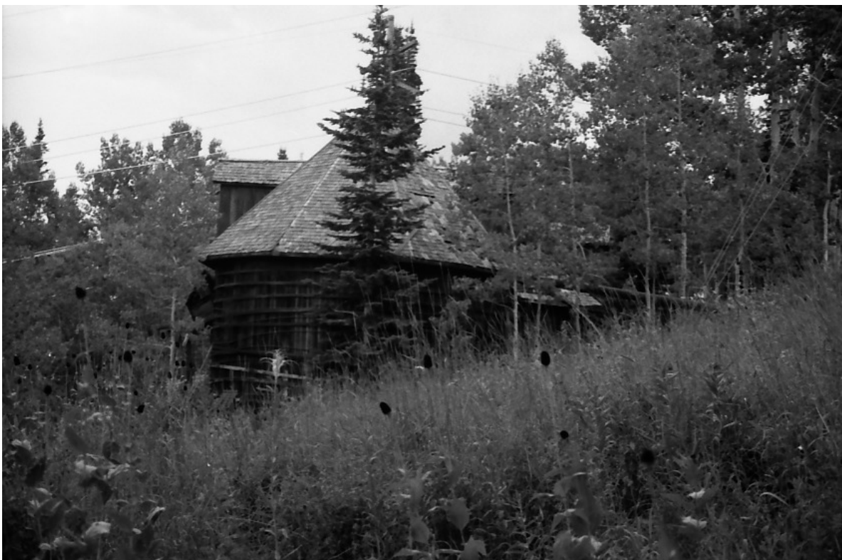
Water Tank D (west elevation), 1999
