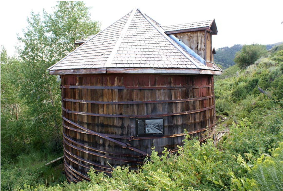
Water Tank A (north elevation), 2009
