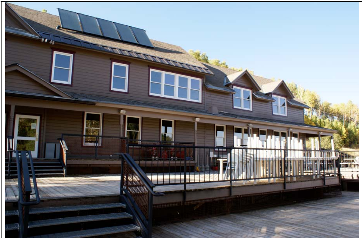
Boarding House (primary façade detail), 2009
