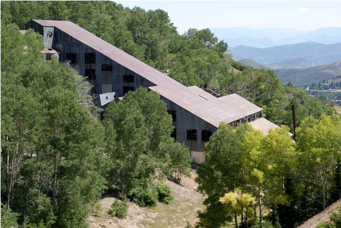
Mill Building (west elevation), 2009
