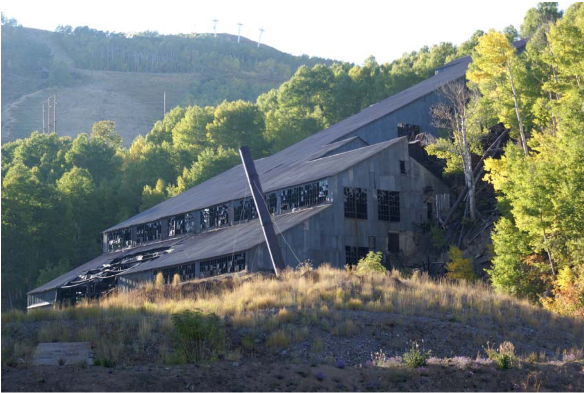
Mill Building (southeast oblique), 2009
