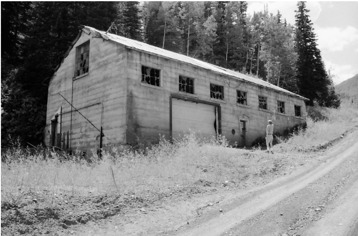
Change House (northeast oblique), 1999
