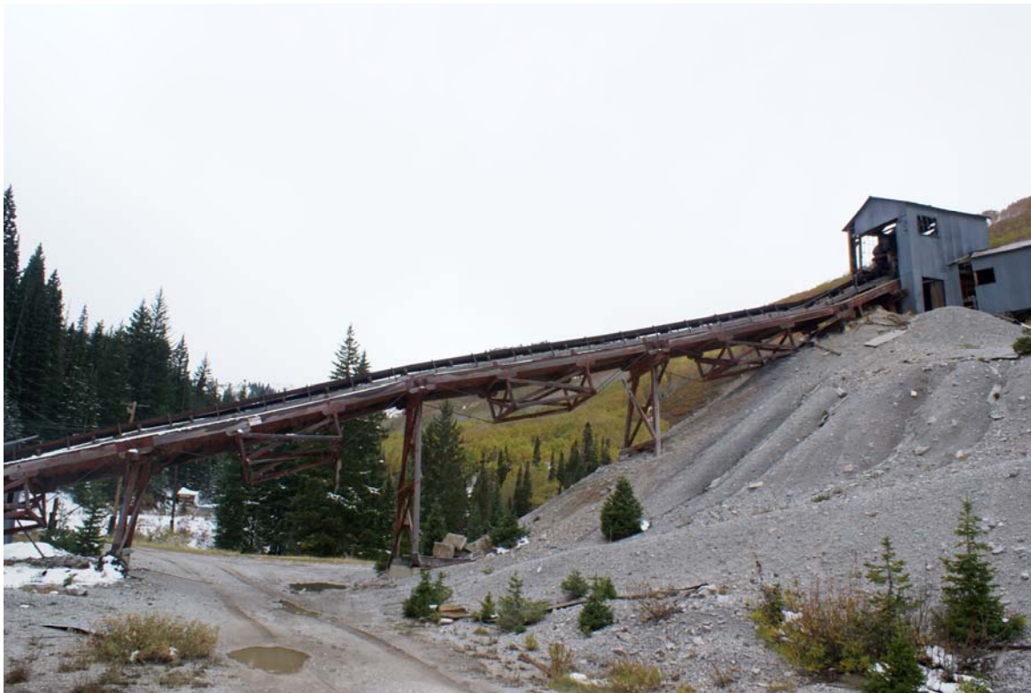
Conveyor Gallery (northeast elevation), 2009
