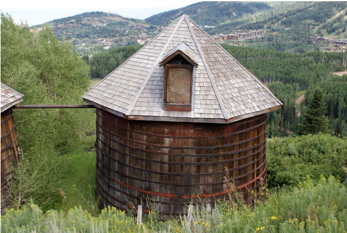
Water Tank B (northwest elevation), 2009
