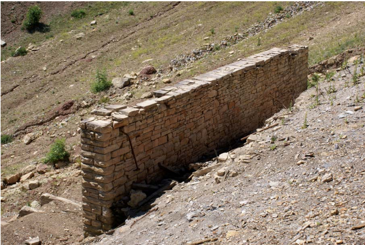
Stone Wall near Mill Building, 2009
