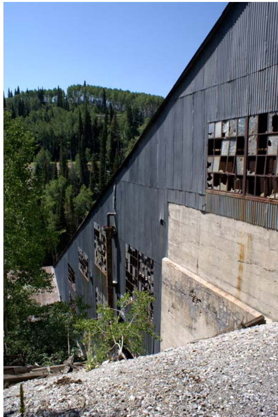
Mill Building (east elevation detail), 2009
