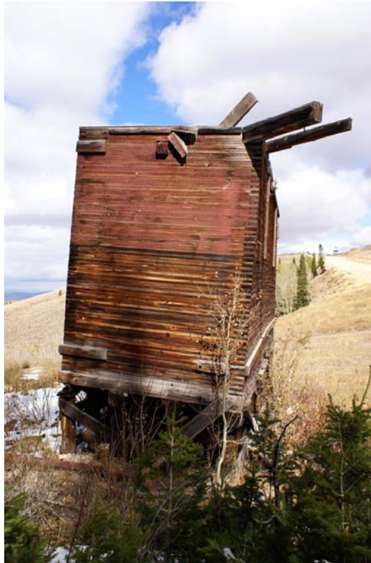
Ore Bin (southwest elevation), 2009
