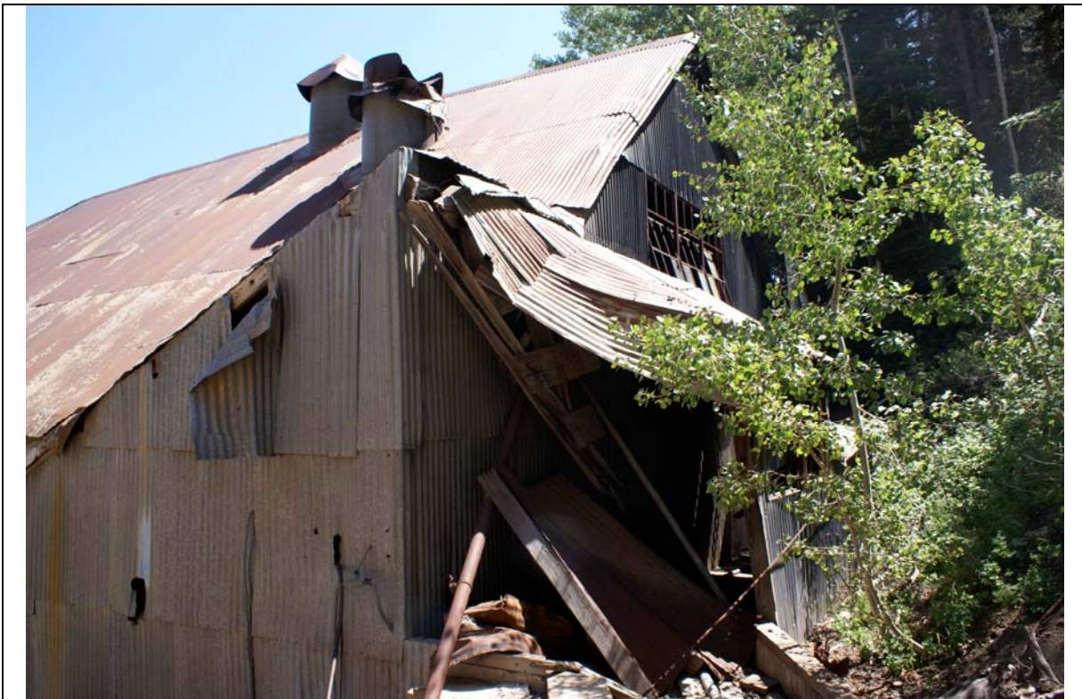
Hoist House (south elevation detail), 2009
