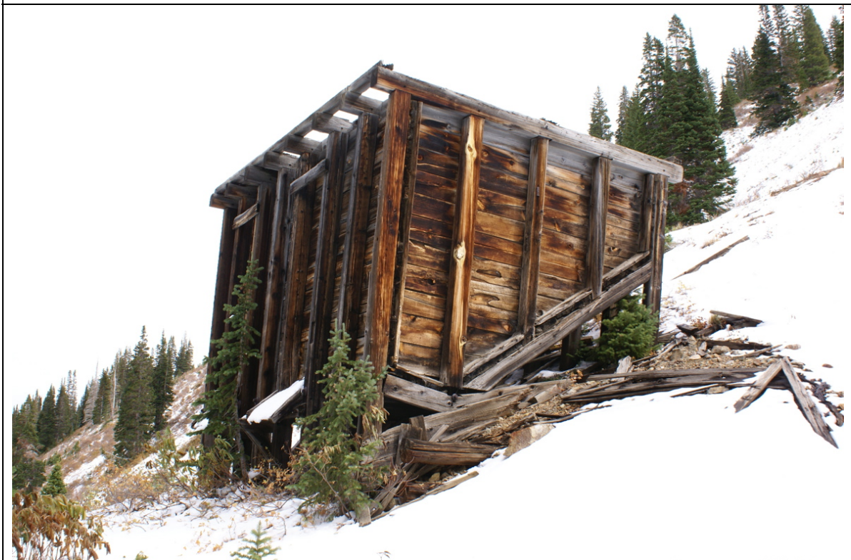
Jupiter Mine Ore Bin (west oblique), 2009
