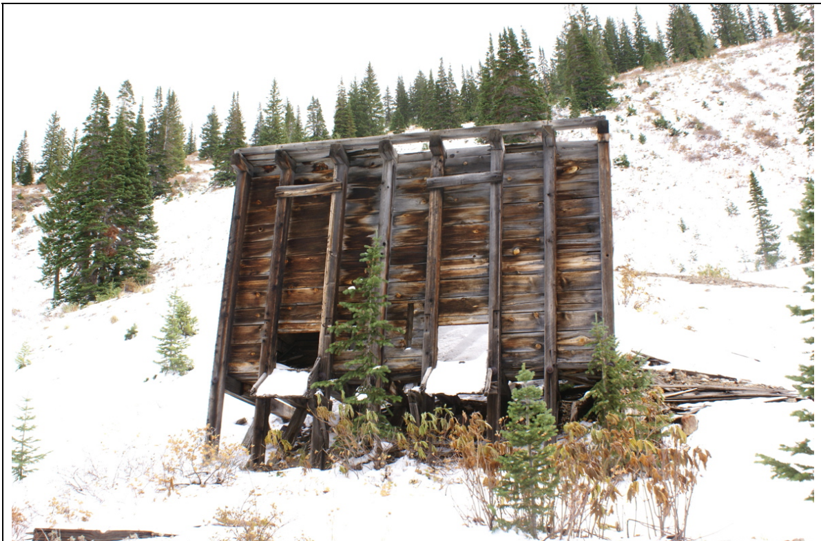
Jupiter Mine Ore Bin (northwest elevation), 2009
