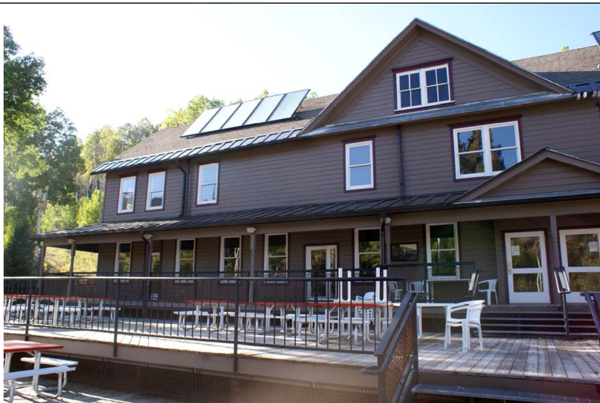
Boarding House (primary façade detail), 2009
