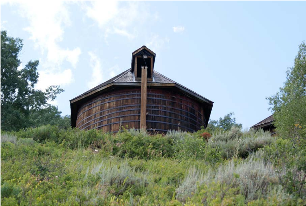
Water Tank B (southeast elevation), 2009
