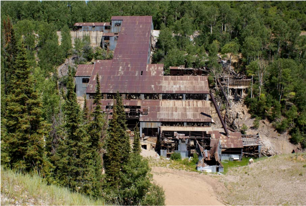
Mill Building (south elevation), 2009
