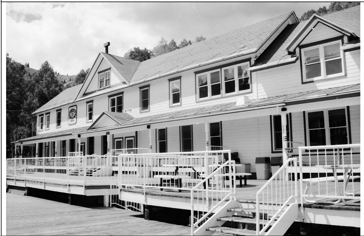
Boarding House (primary façade detail), 1999
