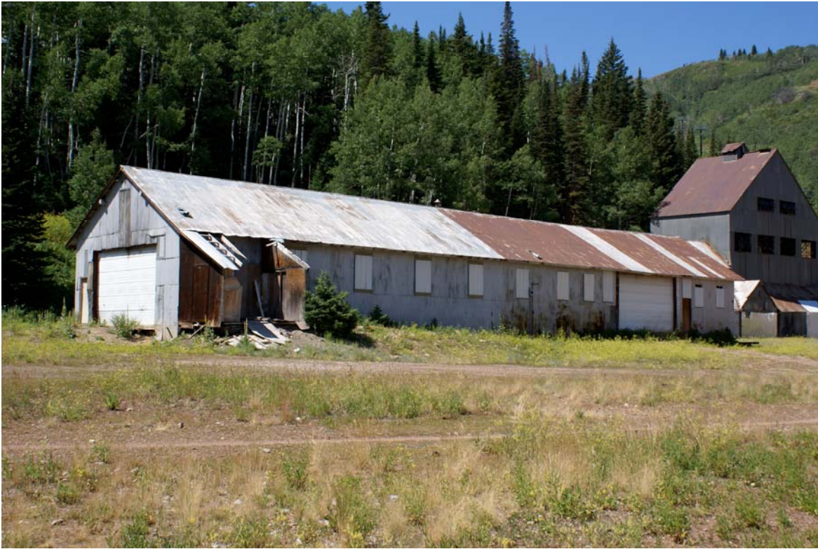
Stores Dept Building (northeast oblique), 2009
