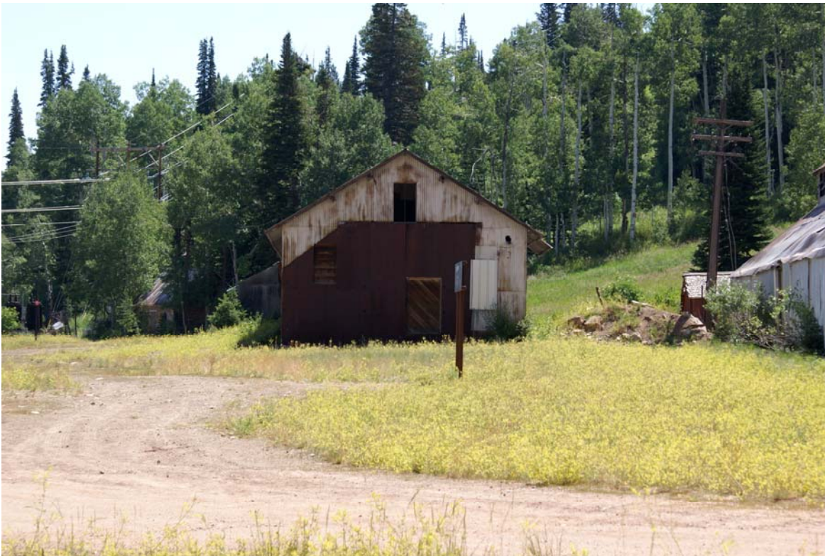
Stores Dept Building (west elevation), 2009
