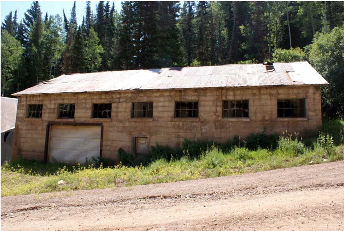
Change House (north elevation), 2009
