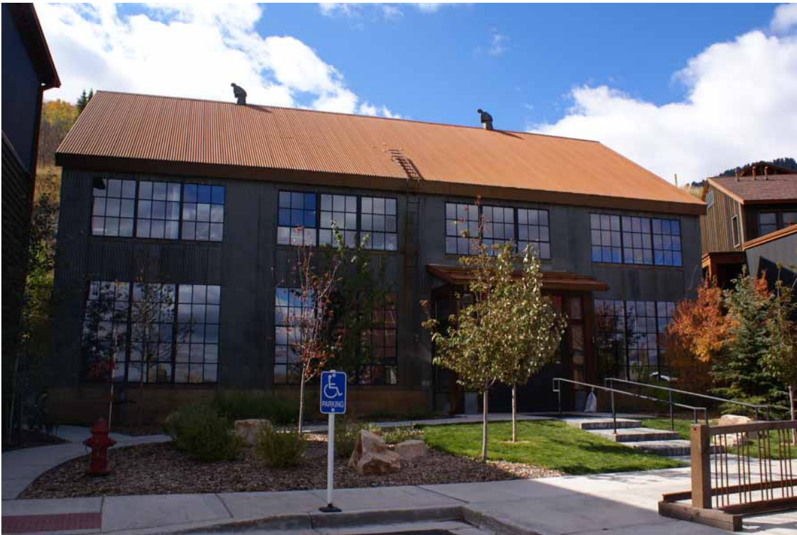
Silver King Consolidated Mine - Spiro Tunnel Site, Compressor House B, 2006
