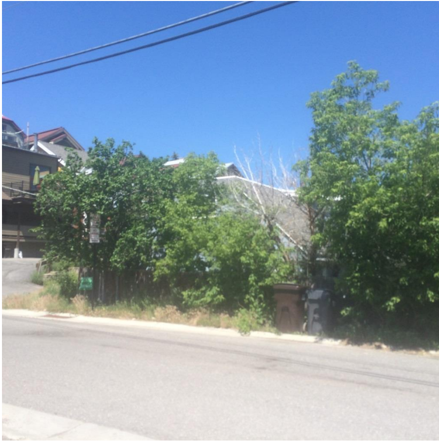
1302 Norfolk Avenue. South Elevation. June 2016.
