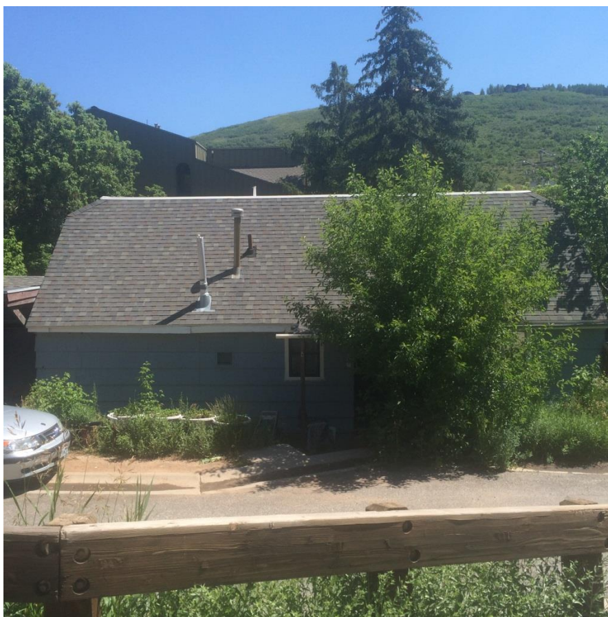
1302 Norfolk Avenue. West Elevation. June 2016.
