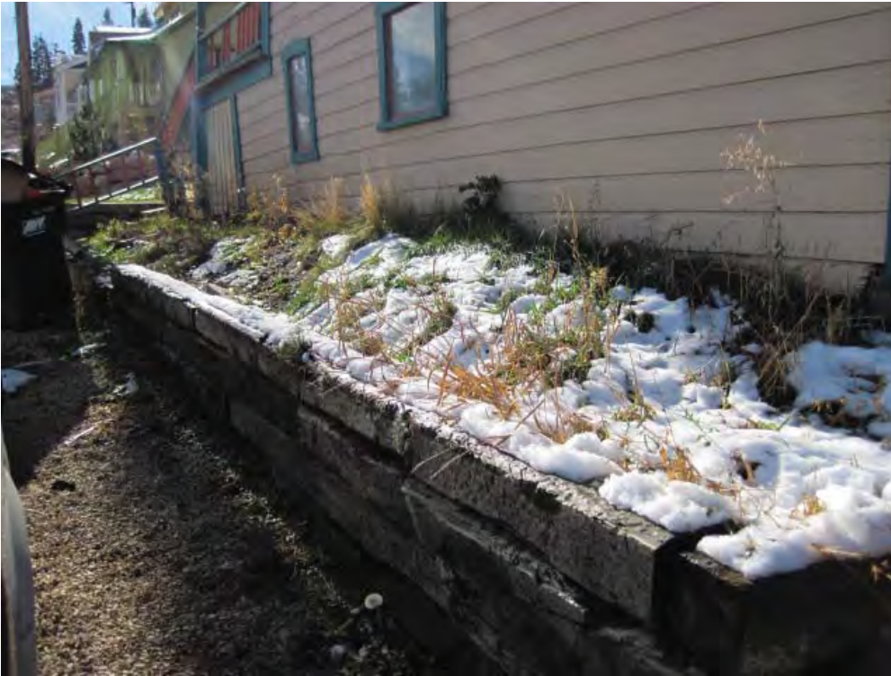
Photo #1: Wood tie retaining wall
