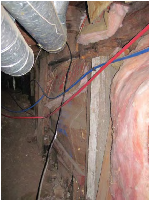
Photo #7: Bearing walls and post on soil
