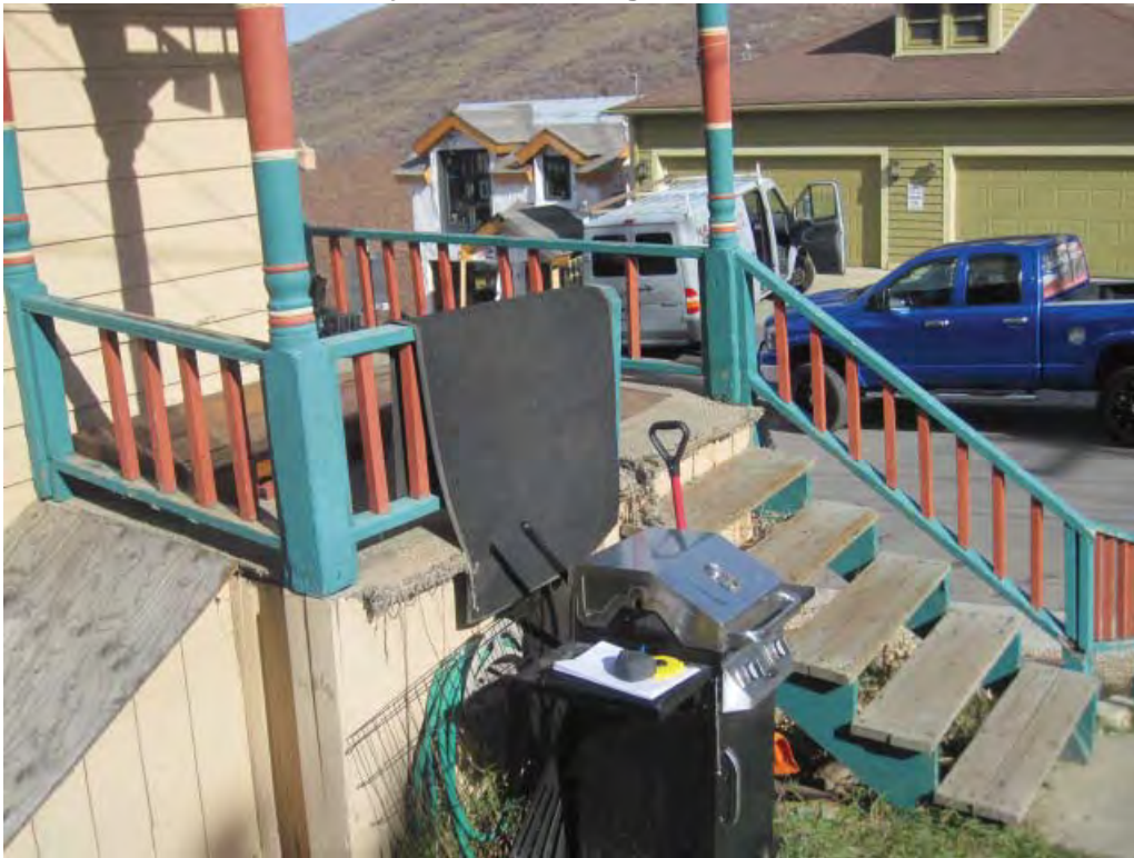
Photo #2: Southeast entry stairs & railing
