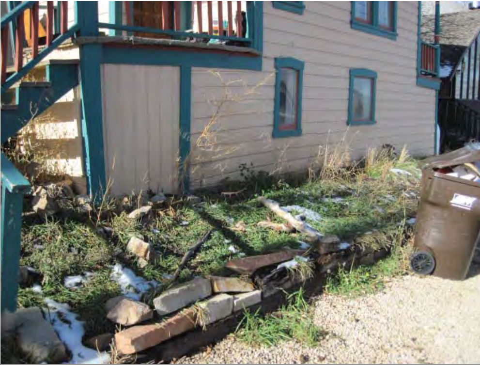
Photo #1A: Wood tie retaining wall
