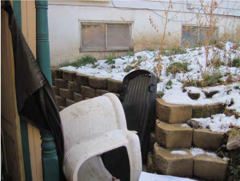
Photo #4: Concrete block retaining wall
