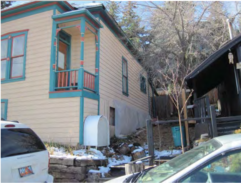
Photo #3: Northeast porch railing
