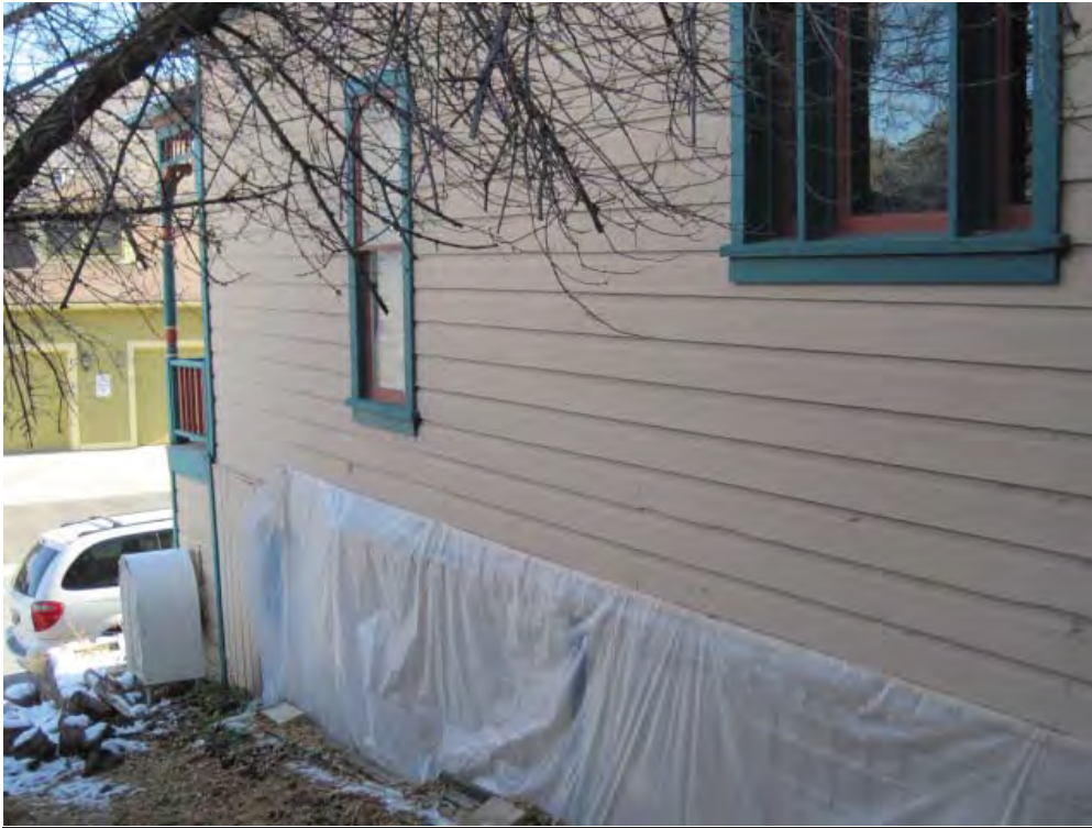
Photo #24: North elevation
