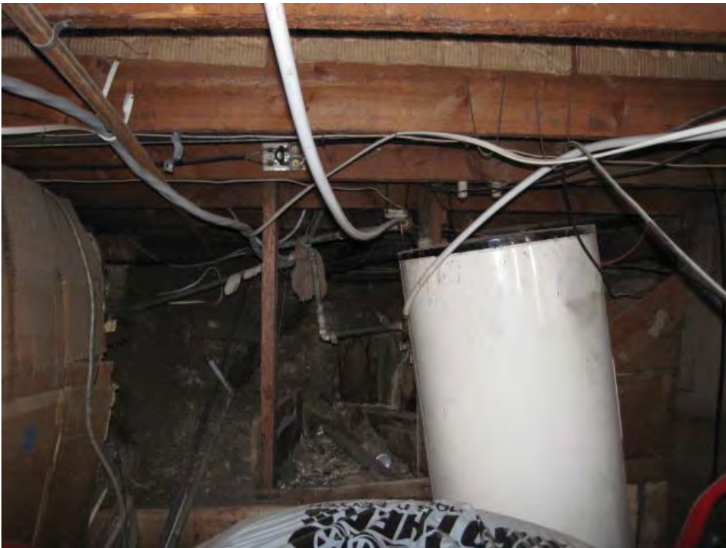
Photo #7: Bearing walls and post on soil
