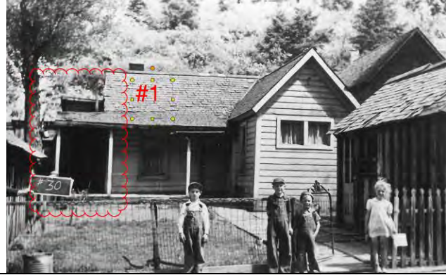
This c.1941 historic photograph shows a shed-roof addition that extends from the rear (east) elevation of the house to the north. It appears in this photograph that the wrap-around porch terminates at this addition on the north side.
