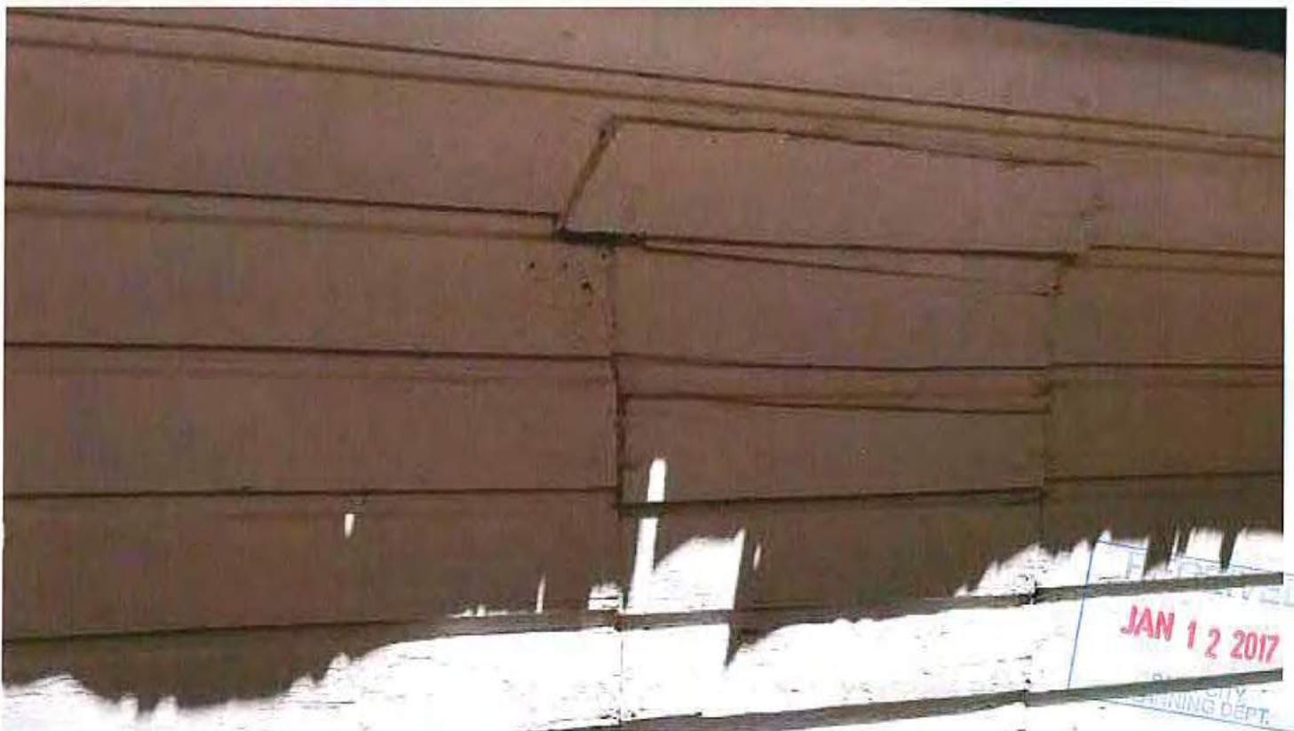
Photo #6: Infilled Window
