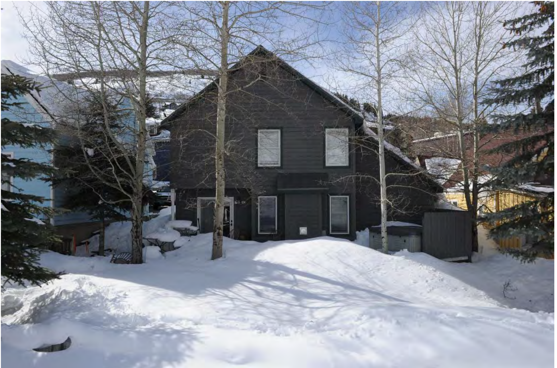
166 Main Street – looking westerly
