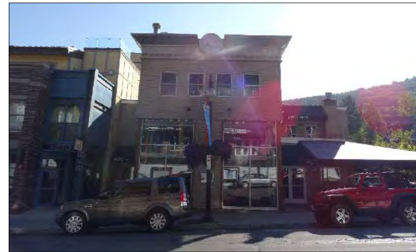
VIEW OF EXISTING BUILDING (LOOKING NORTHEAST)
