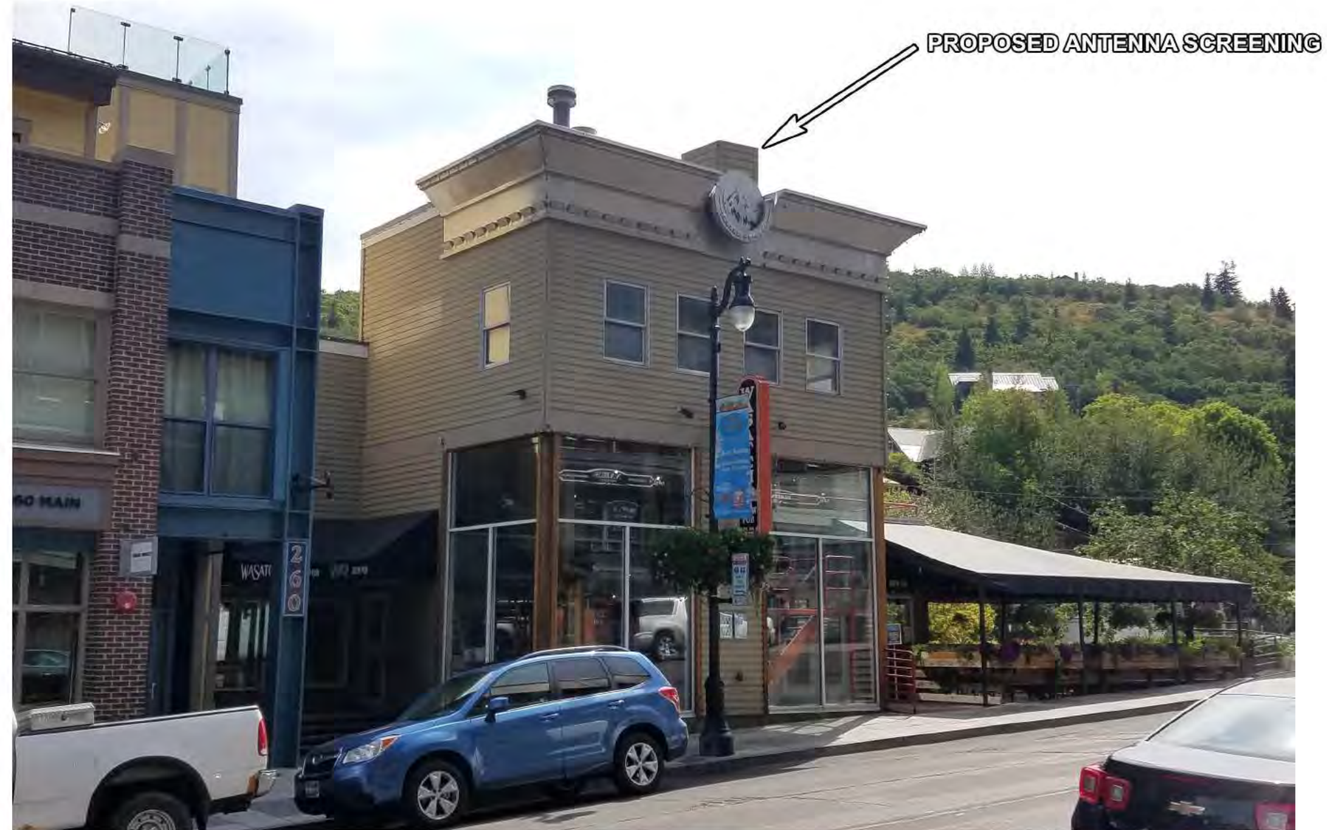
WEST ELEVATION (LOOKING EAST)
