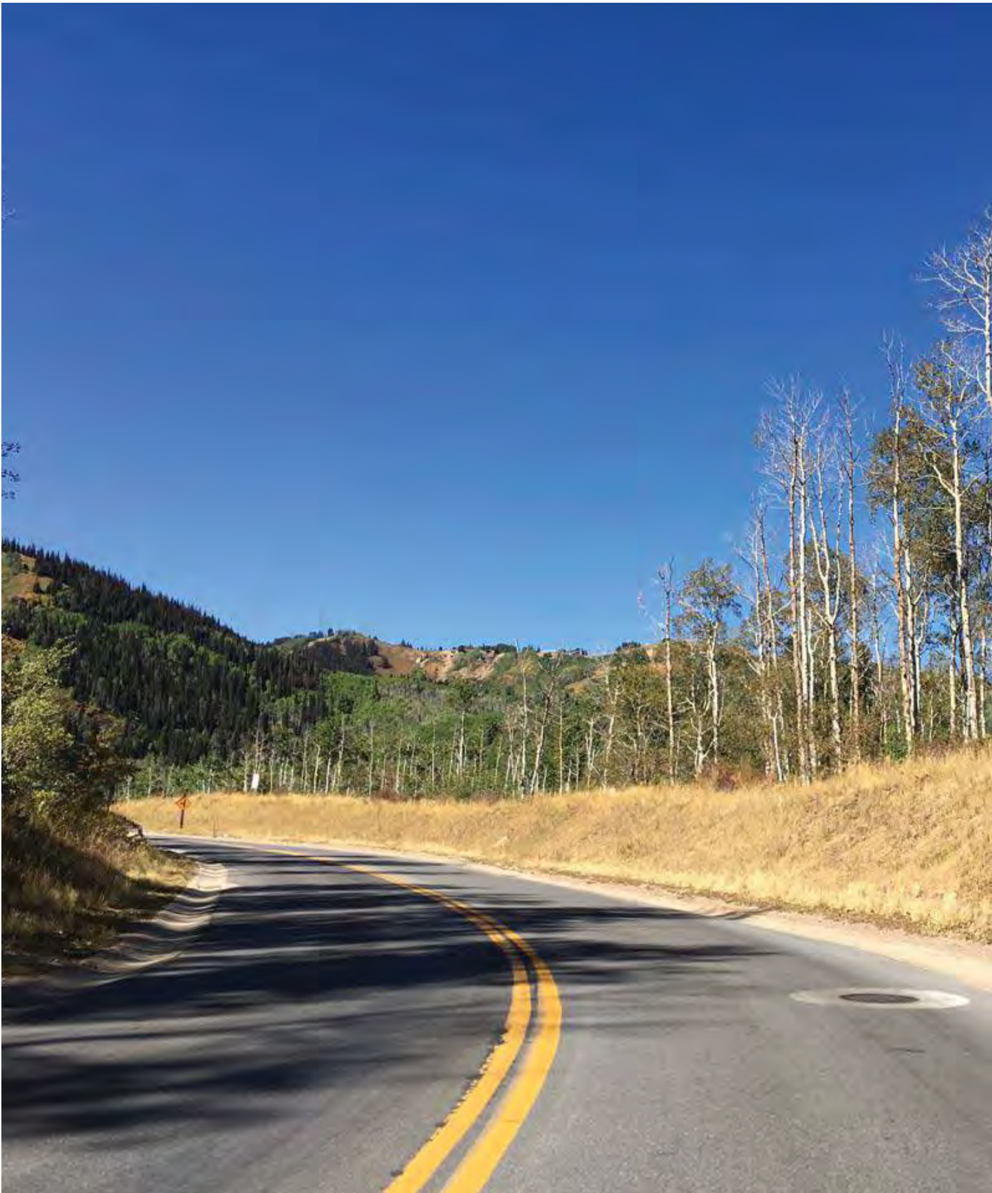
Looking northwest from Marsac - Lot 1 is on the right.
