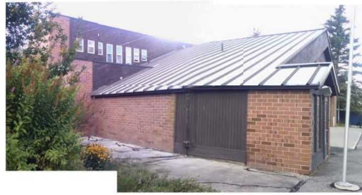
4. View From North Elevation
