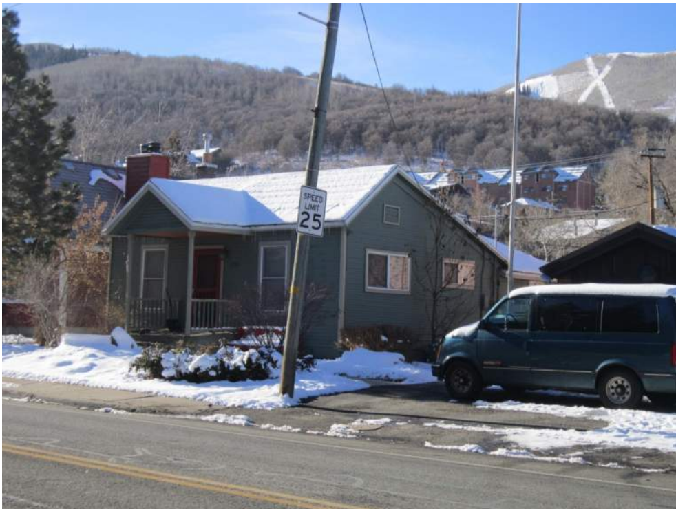
1333 Park Avenue. Northeast oblique. November 2013.
