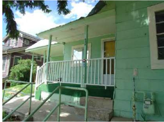
Current photograph of the house showing contemporary wood railing.
