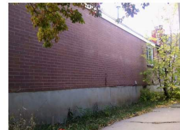
8. View From South Elevation
