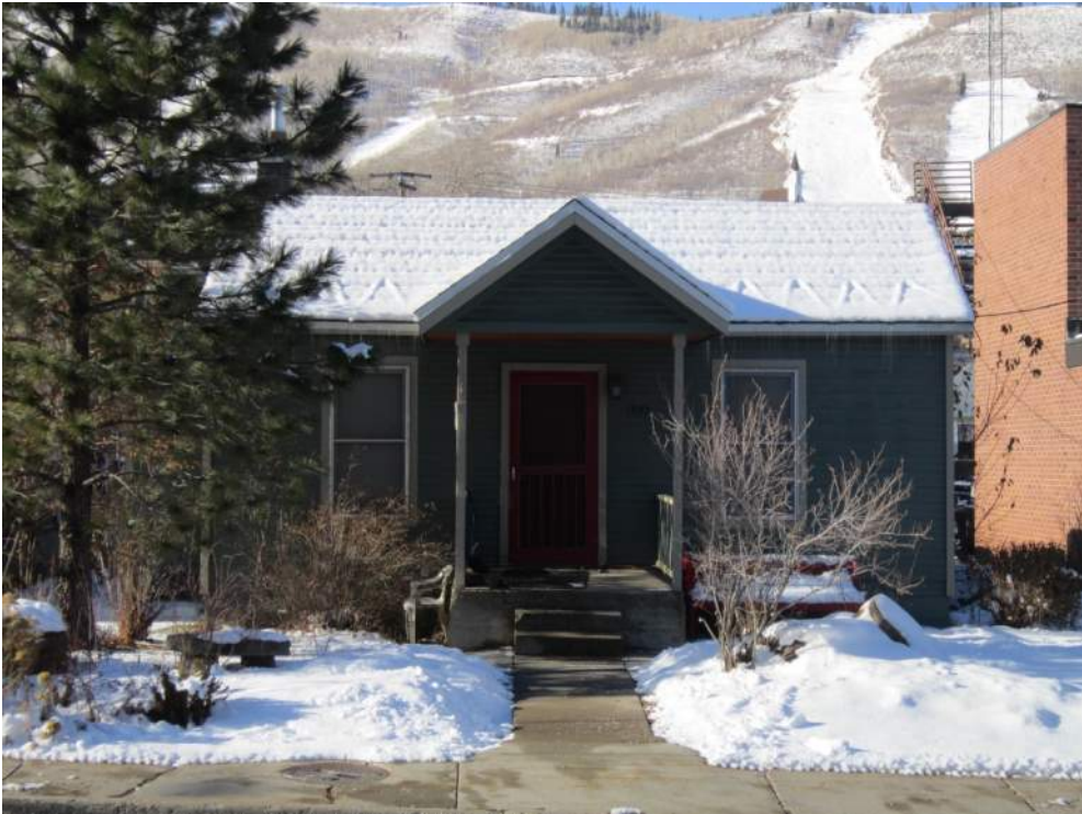
1333 Park Avenue. East elevation. November 2013.
