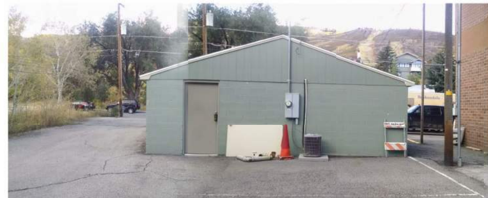
6. View From West Elevation
