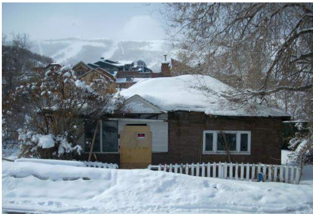
Figure 4: Photograph prior to removal ca. 2009.
