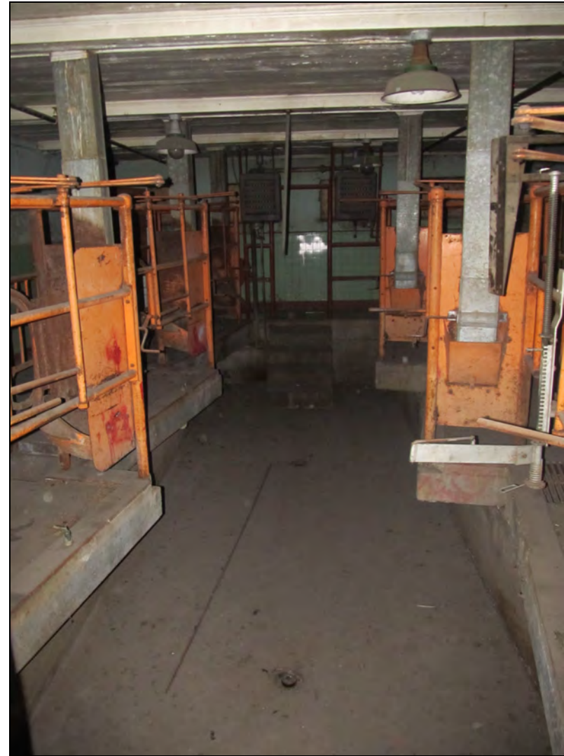
Figure 50. Lower-level work area between milking pens, facing northeast.
