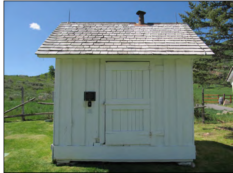
Figure 66. Bunkhouse, facing southwest.
