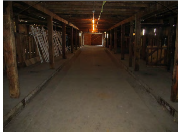
Figure 38. General view of main level, facing southwest.
