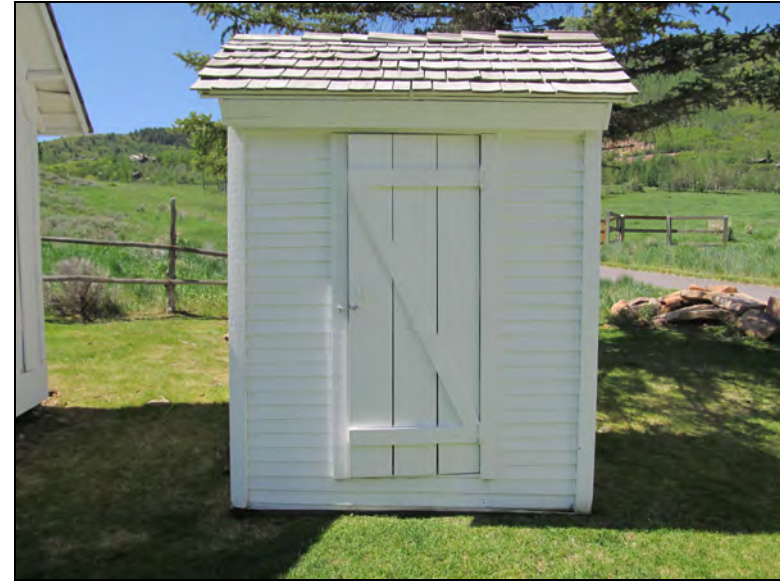
Figure 64. Outhouse, facing southwest.
