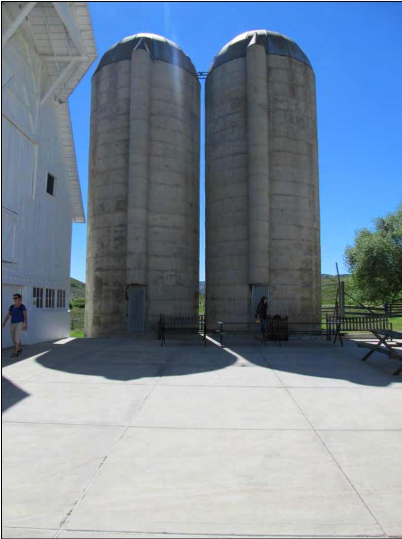
Figure 68. Grain silos, facing southeast.
