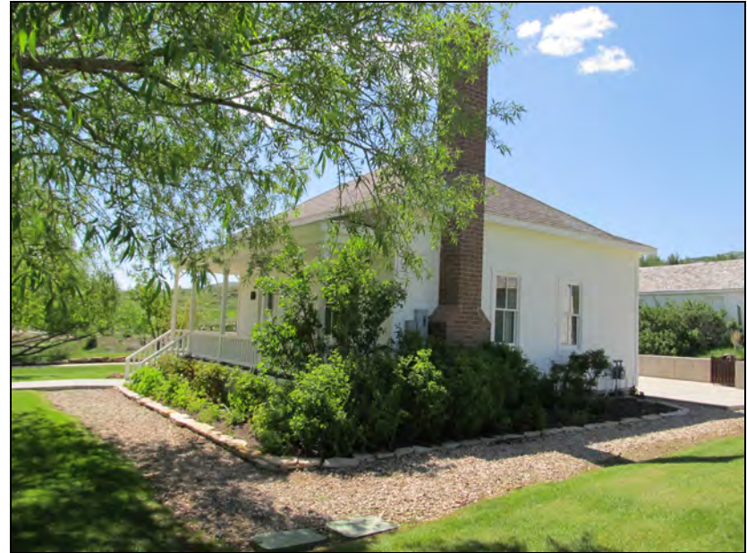
Figure 72. Reconstructed farmhouse, facing south.
