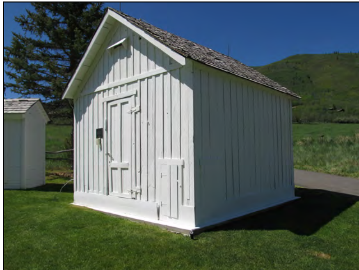
Figure 62. Tool shed, facing south.
