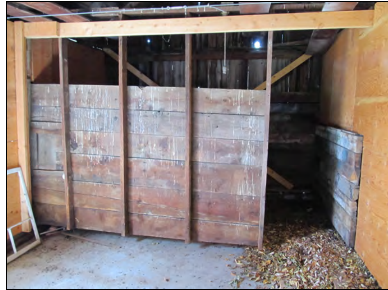
Figure 59. Half wall dividing interior of granary, facing southeast.
