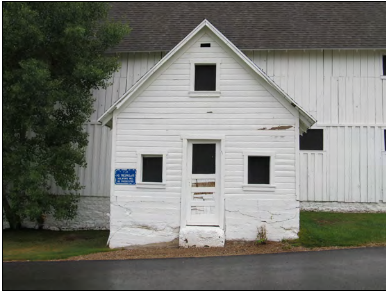
Figure 42. Milk house, facing southeast.
