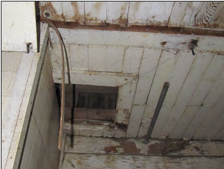
Figure 46. Attic access door in ceiling of milk house.
