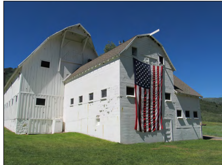
Figure 33. McPolin barn, facing west.
