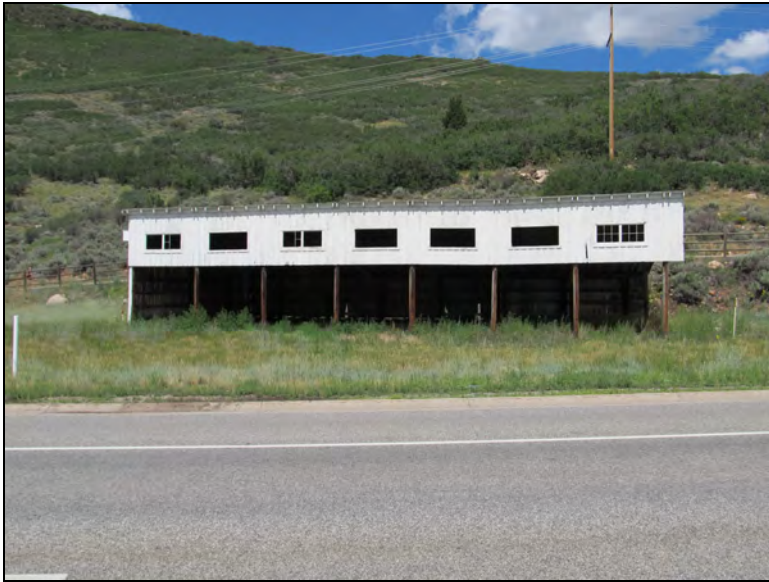
Figure 9. Osguthorpe shed, facing northeast.
