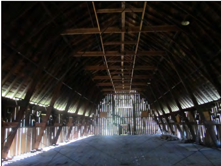
Figure 41. Upper-level hay mow, facing southwest.
