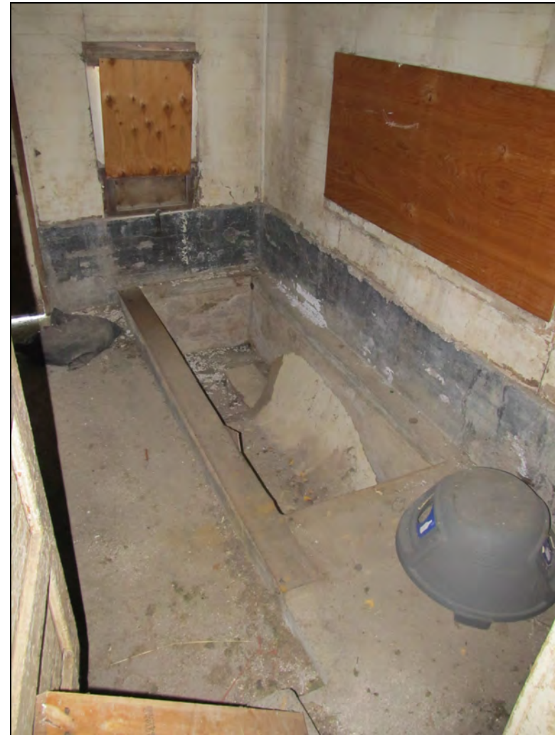
Figure 44. Concrete cooling tank built into milk house floor, facing north.
