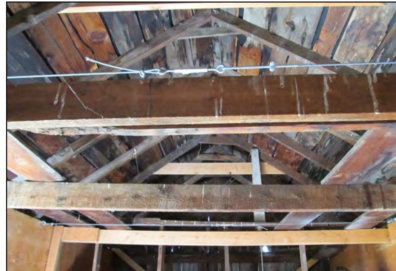
Figure 60. Exposed roof framing and cable bracing on granary interior, facing southeast.
