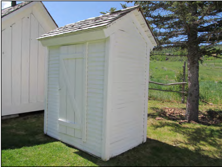
Figure 6. Outhouse, facing southeast.
