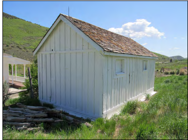
Figure 4. Granary, facing east.
