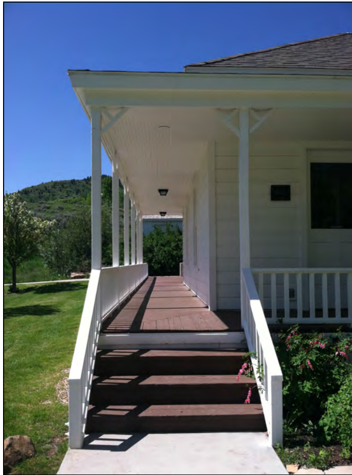
Figure 73. Stairs and porch on southeast side of farmhouse, facing southwest.
