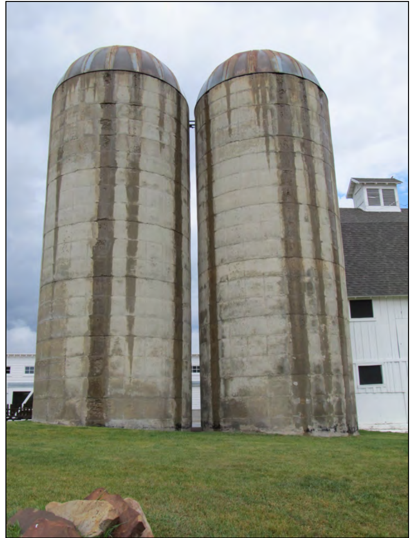
Figure 8. Grain silos, facing northwest.
