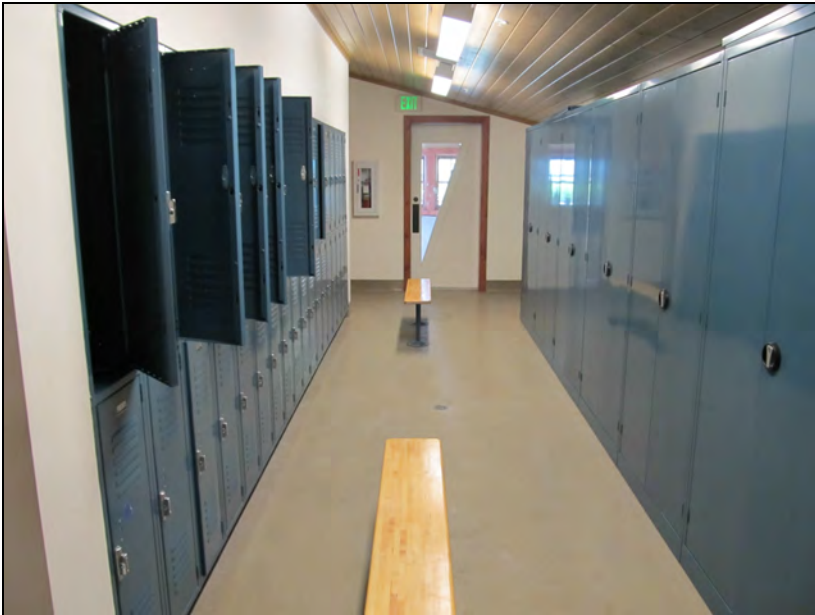
Figure 80. Locker room at southwest end of reception center, facing southwest.
