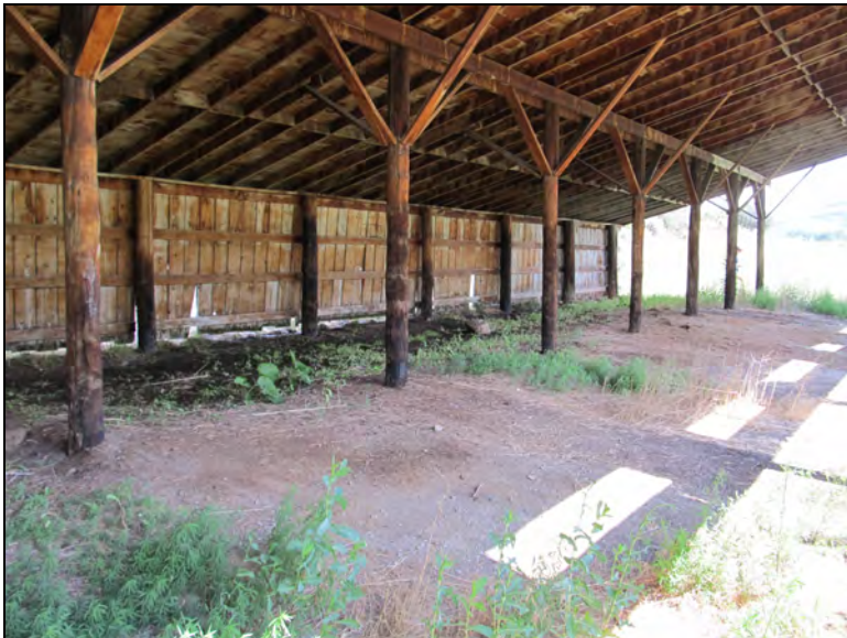
Figure 70. Osguthorpe shed interior, facing east.
