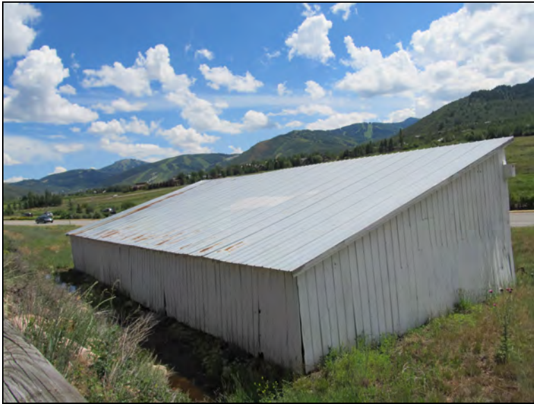
Figure 69. Osguthorpe shed, facing south.
