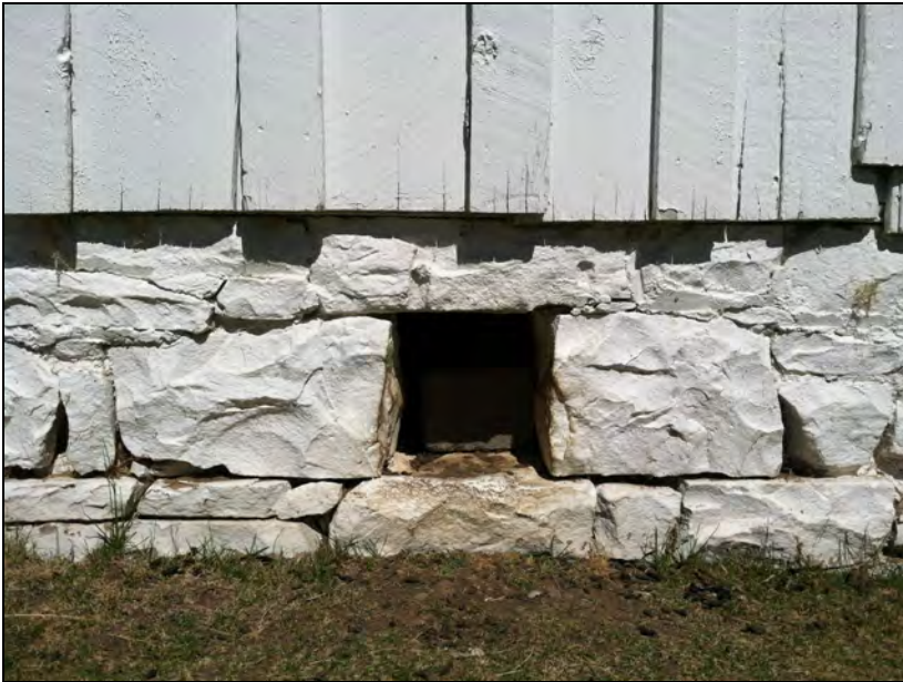
Figure 36. Sandstone foundation, painted white, with opening for basement ventilation.
