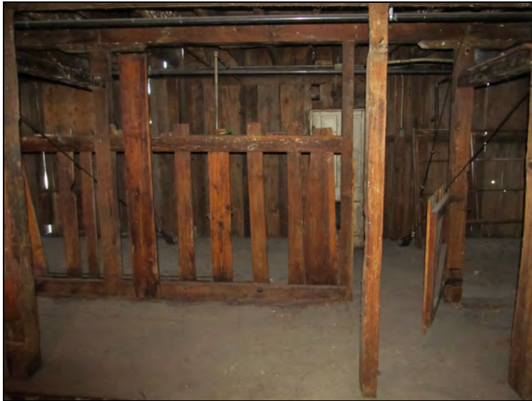
Figure 40. Wood stanchions on main level, facing northwest.
