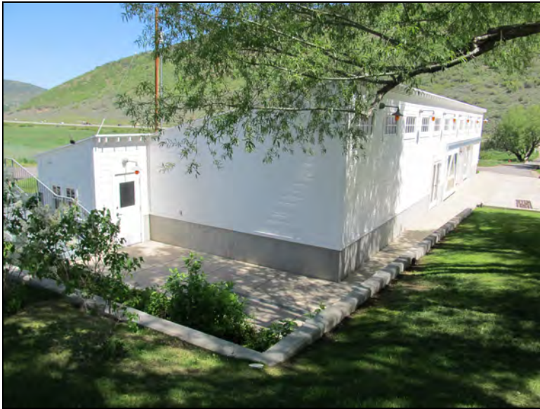
Figure 76. Reception center and locker room entrance, facing north.
