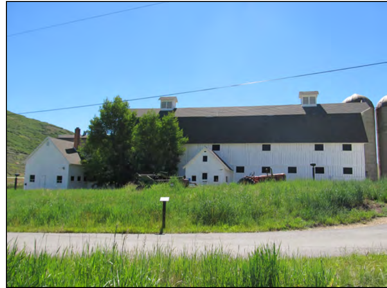
Figure 32. McPolin barn, facing southeast.
