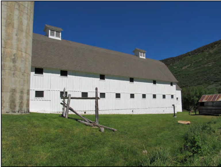
Figure 34. McPolin barn, facing north.
