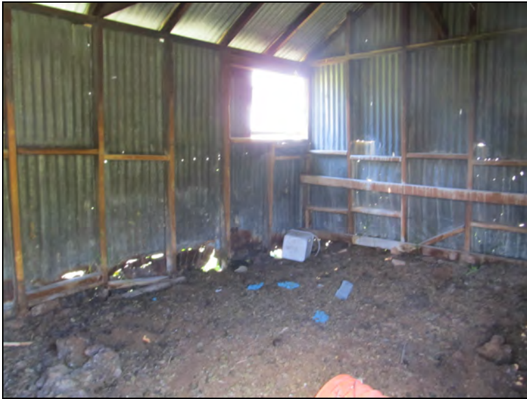
Figure 56. Interior of animal shelter, facing southwest.
