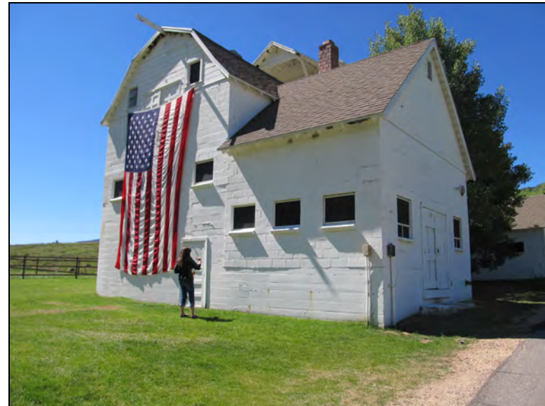
Figure 47. Milking parlor, facing south.
