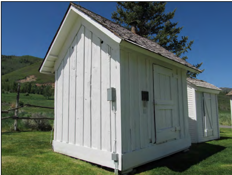
Figure 7. Bunkhouse, facing southwest.
