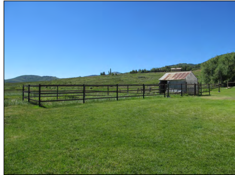
Figure 54. General view of corral with animal shelter, facing southeast.
