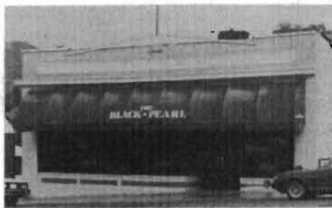
This building, shown as the Golden Rule Mercantile Company in the historic photo above, is now the Black Pearl.
