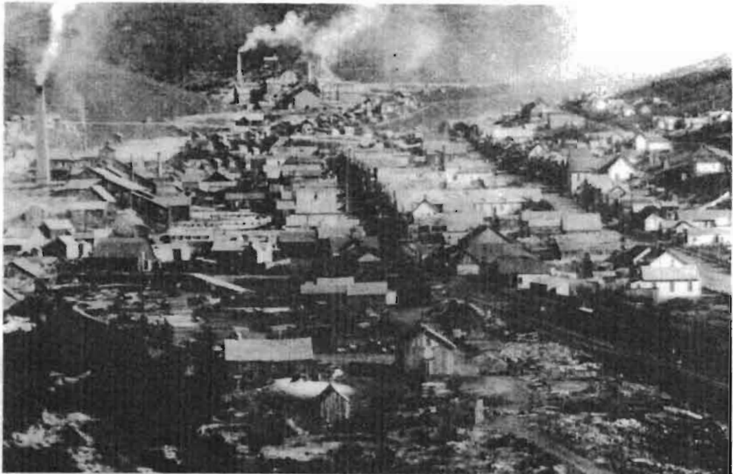
Park City's heritage derives from its days as a mining center. The buildings that survive from this period represent the character of life in a mountain mining town. (Bea Kummer collection)
