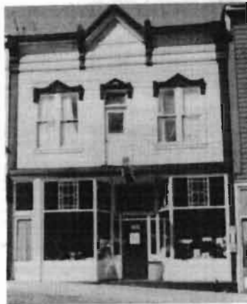
The door at the second level indicates a balcony once was on this building.
