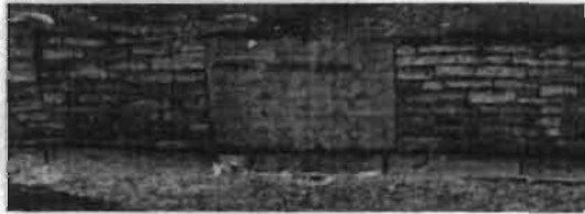
Patches in historic retaining walls should match the original. The mortar joints in this patch are not appropriate.
