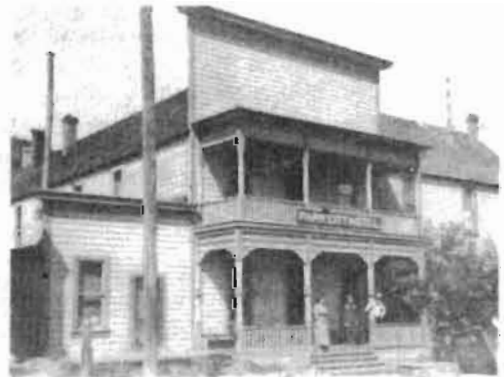
Park City Hotel—now the site of the Claimjumper. (Demolished)
