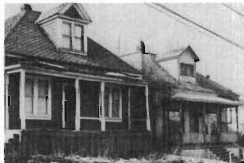
These roof shapes should be retained. The windows in the far dormer should be restored to a vertical emphasis.
