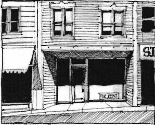
Inappropriate: Original storefront components removed.
