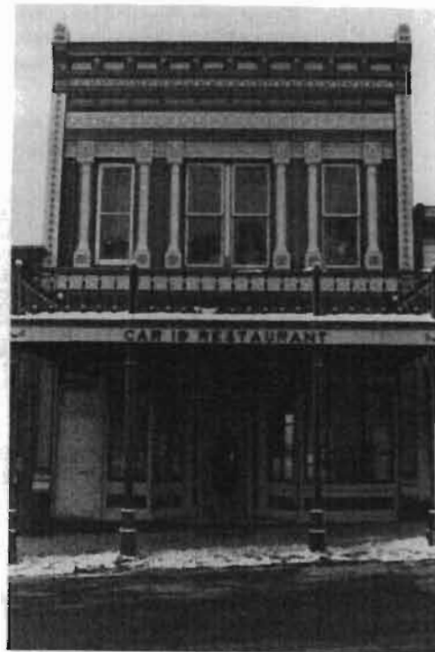
Notice how the paint scheme has highlighted the details of this pressed metal facade.
