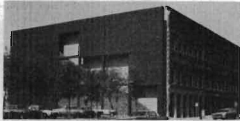
An addition to the side of this building houses a new exit stair. Its simple design is subordinate to the front facade.
