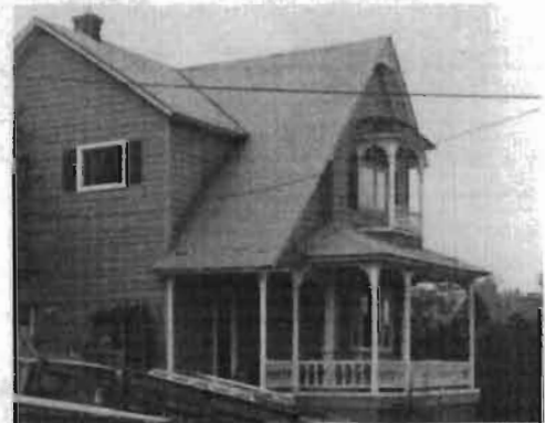
These porch details are appropriate: turned wood posts, decorative trim and railing. The railing heights are typical.
