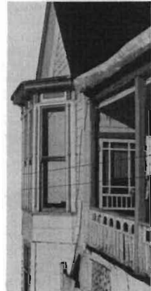
A contrasting trim color accentuates the unique details of window bands. Notice the brackets on the bay window, and the cut out arches on the balustrade. The screen doors are also typical.
