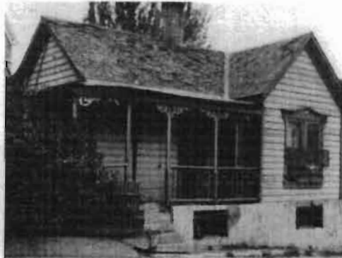
These asbestos shingles cover the original wood siding of this house. Compare the perceived scale of this house with that of the house below.
