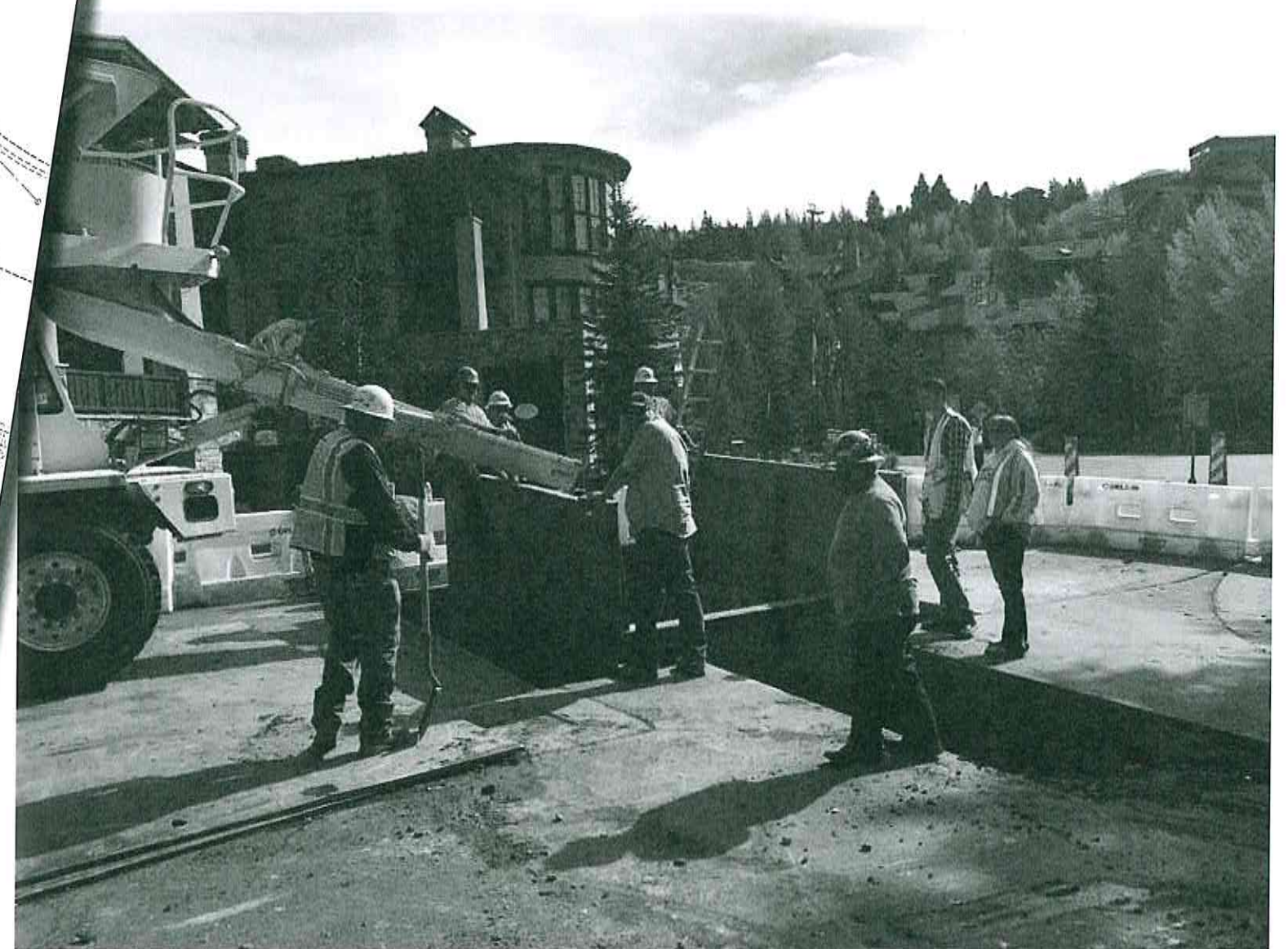
SEWER EASEMENT/ UTILITY WORK COMPLETED
