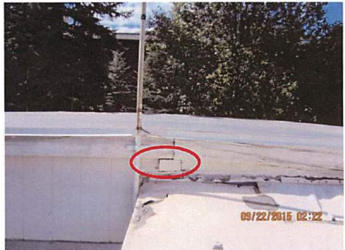
Photo 8 Note structural beam. Refer to photo 9
