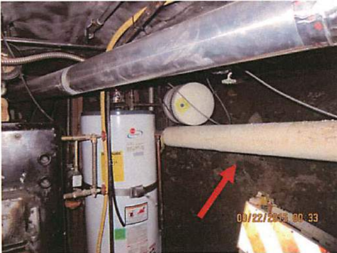
Photo 1 The structure has no concrete or stable foundation. The foundation consists of rubble, dirt and lose stone matter.
