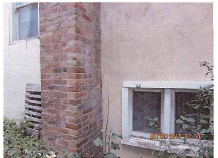
Photo 40 Egress path from other side of building. No safe access to main street
