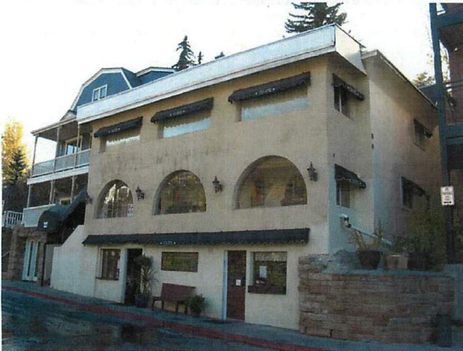
227 Main Street. Northeast oblique. October 2013.
